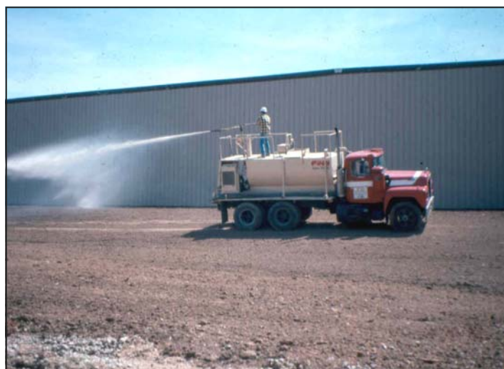
Figure 3: Hydroseeding
