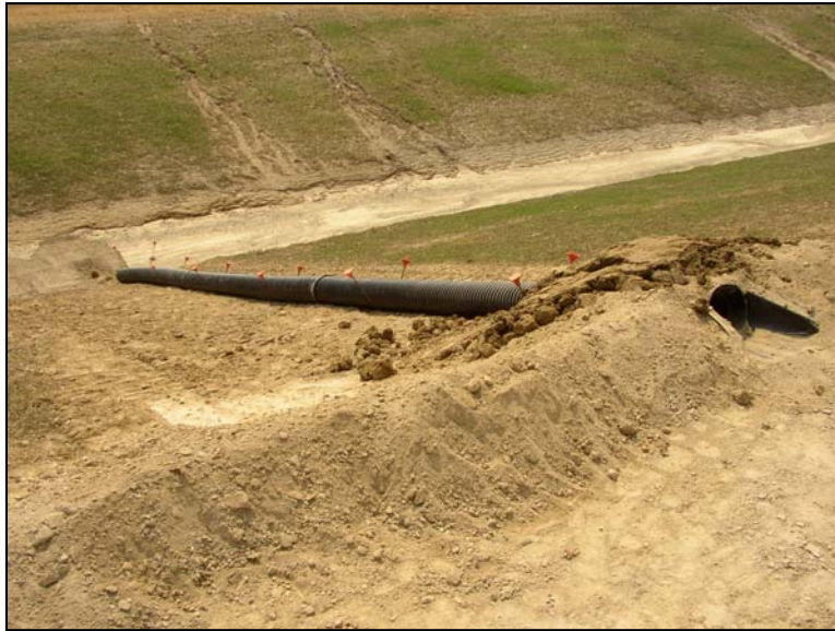
Figure 1: Temporary Slope Drain with Flared-End Section
