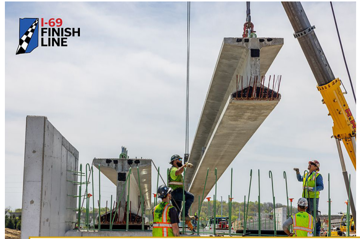
I-69 Finish Line beam setting over Little Buck Creek, May 2022
