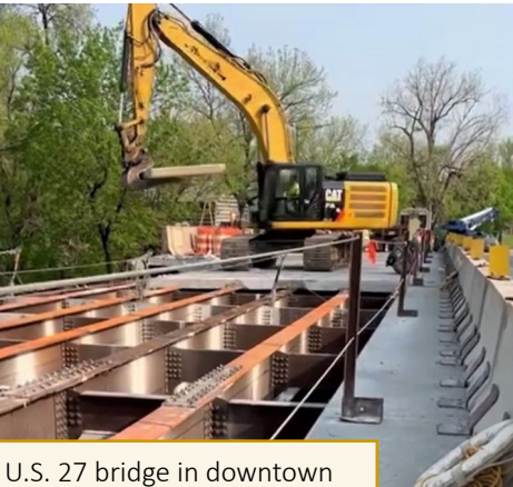
U.S. 27 bridge in downtown Fort Wayne, May 2022.
