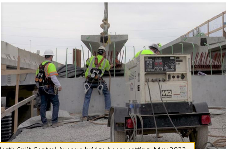
North Split Central Avenue bridge beam setting, May 2022
