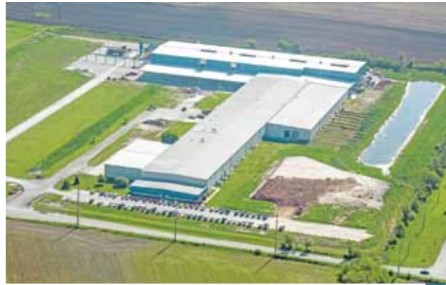
Completed Modern Forge facility in Merrillville.
