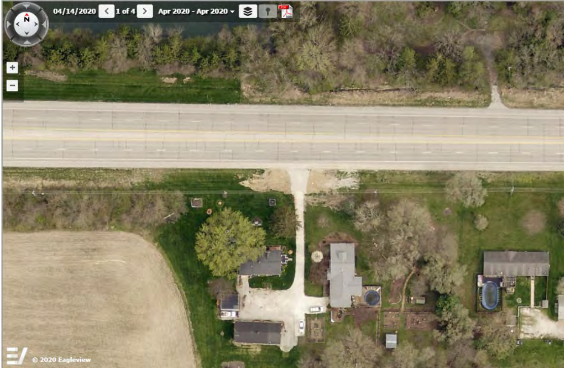
Figure 2 – Aerial view of the sewer repair site at 3725 US 52 showing construction on both sides of the restored driveway.
