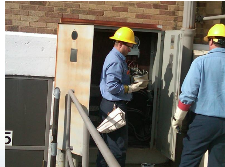
IPL Metering installs new AMI demand meter at an IPS school.
