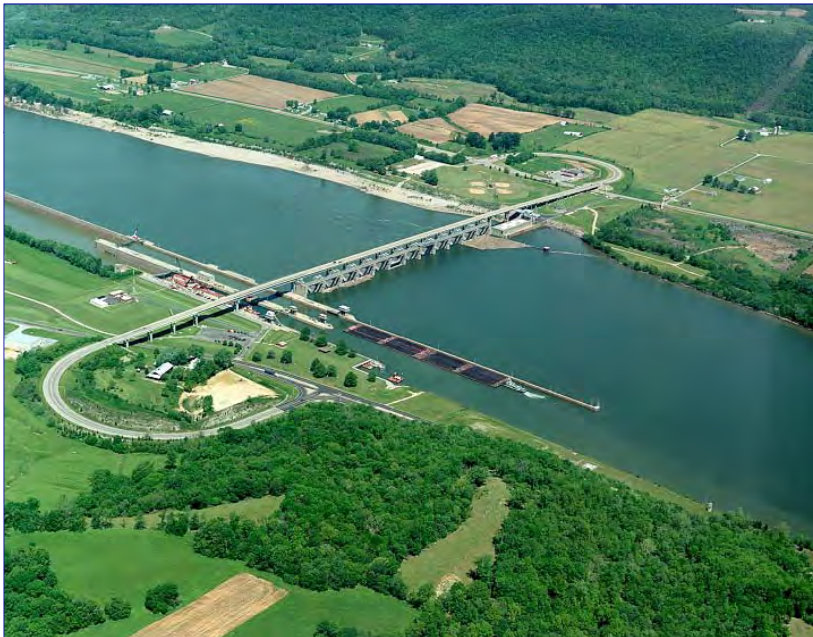
Markland Hydro Generating Station
