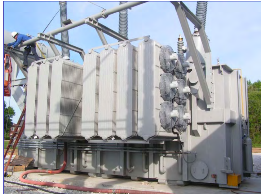
Installation of Dresser 450 MVA 345/138 kV Transformer
