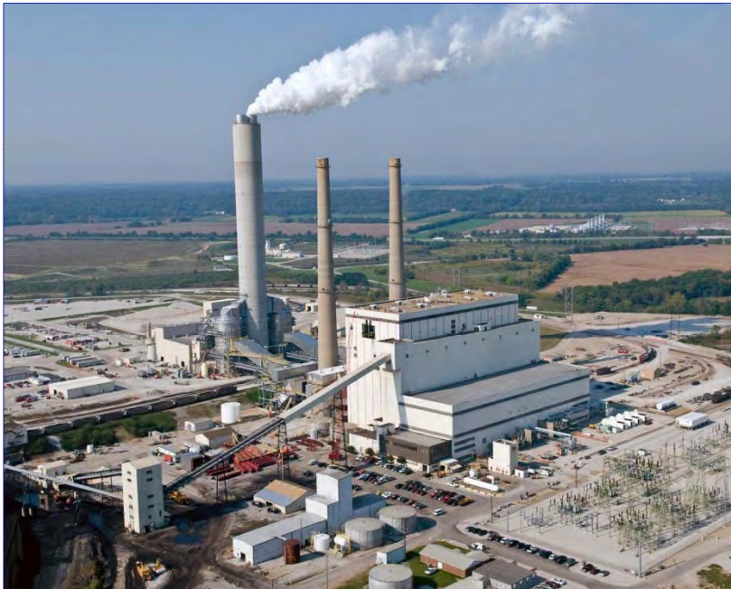
Cayuga Generating Station with New FGDs
