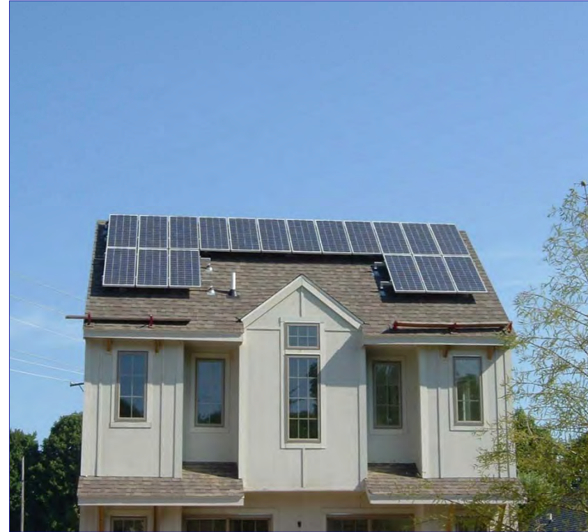
2 kW Solar Installation in Evergreen Village, Bloomington, IN
