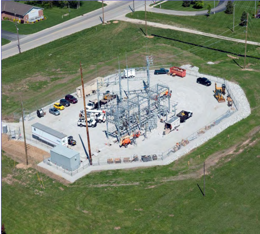
Plainfield West Substation Construction – April 2010
