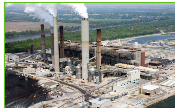
Gibson Station – April 2008
