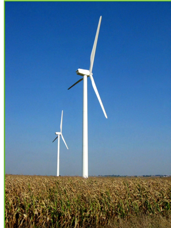
Benton County Wind Farm
