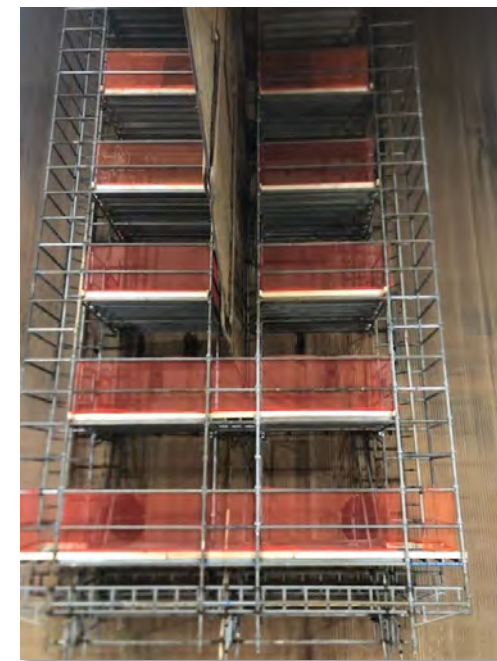
Gibson Unit 3 – Boiler Division Wall Scaffold
