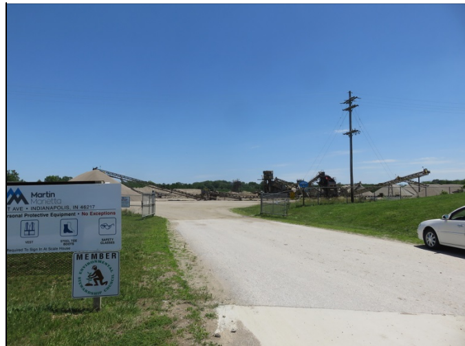
Figure 5.15-4: Entrance to Martin Marietta Aggregates
