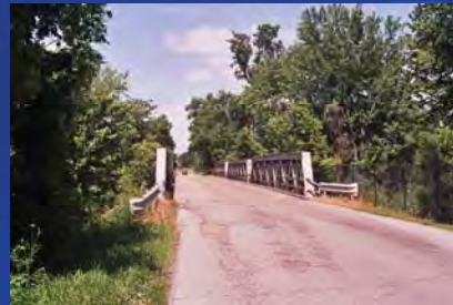
County Bridge No. 224, Old SR 37, c.1925 Morgan County
