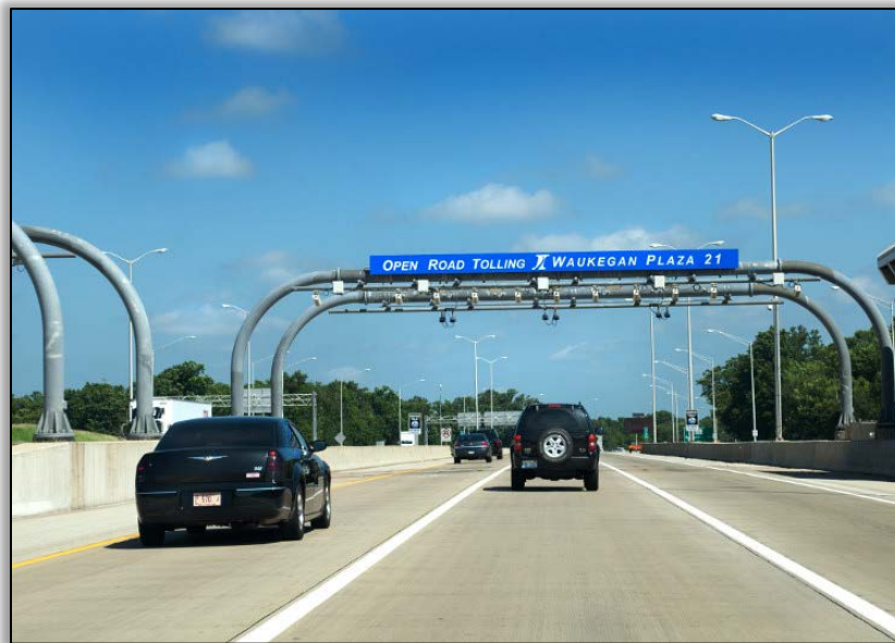
Figure 4-1. Example of Monotube Toll Gantries (Illinois Tollway)
