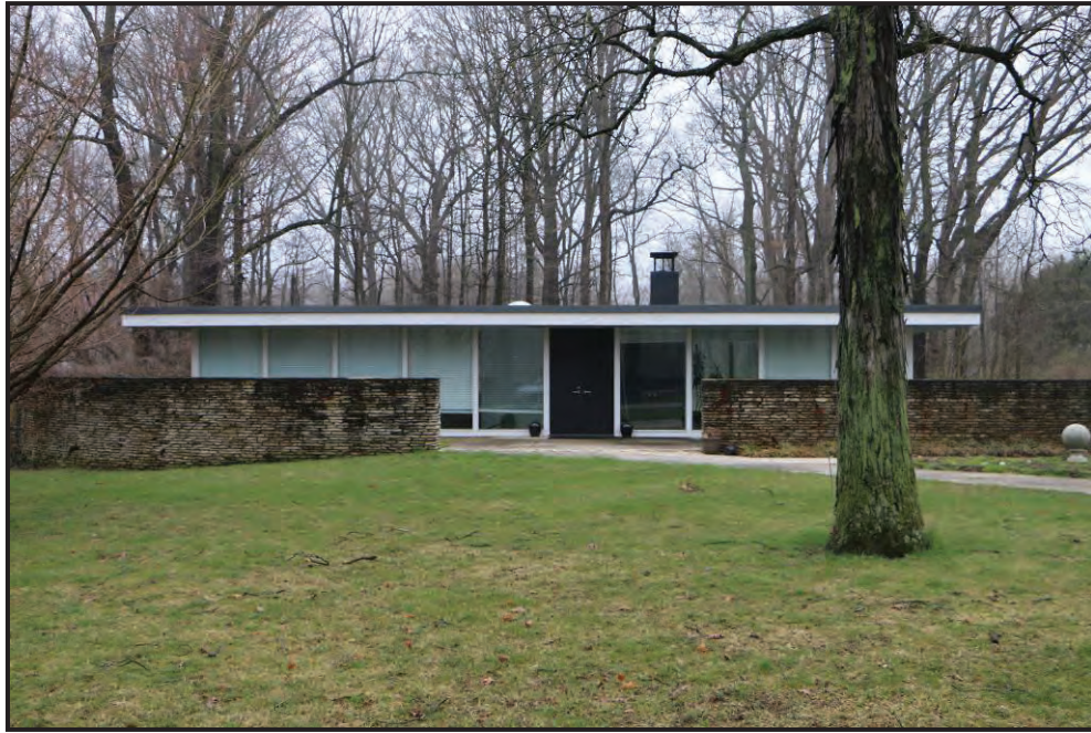
FIGURE 91. CONTEMPORARY-STYLE ORUS EASH HOUSE, BRIERWOOD HILLS SUBDIVISION, FORT WAYNE, ALLEN COUNTY
