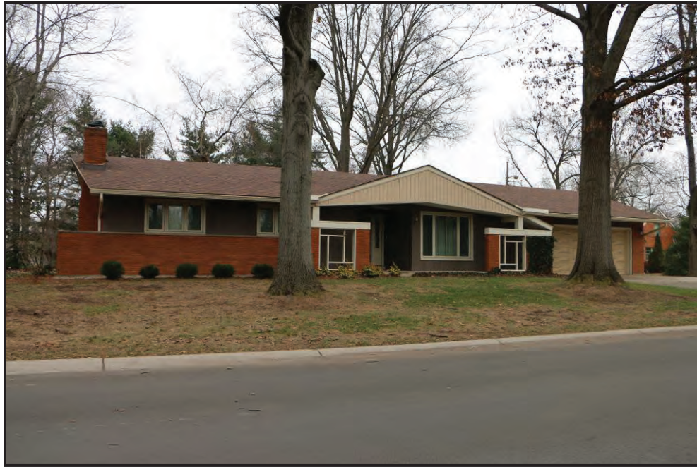
FIGURE 89 RANCH HOUSE WITH CONTEMPORARY INFLUENCES, CHEROKEE HEIGHTS SUBDIVISION, JEFFERSONVILLE, CLARK COUNTY
