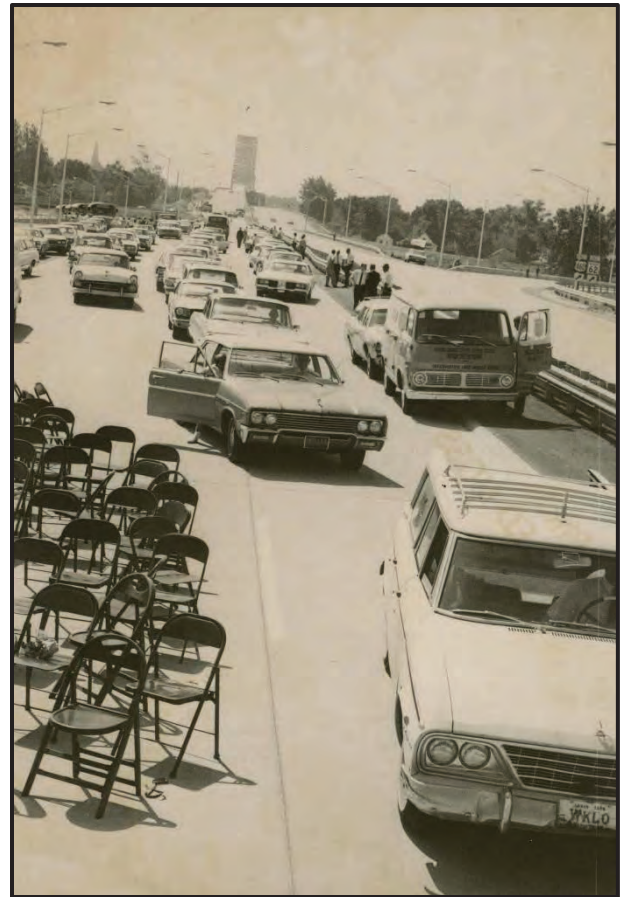
FIGURE 31. OPENING OF THE I-64 SPRING STREET RAMP IN NEWALBANY, 1968
