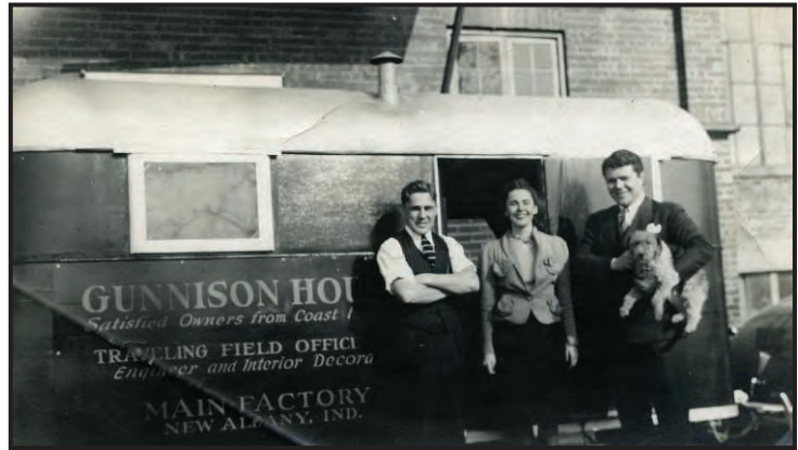
FIGURE 59 GUNNISON HOMES TRAVELING FIELD OFFICE, c. 1940
