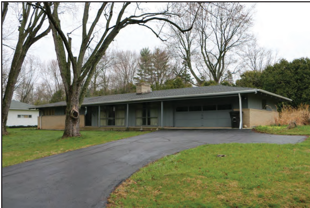
FIGURE 77. LINEAR RANCH, BRIERWOOD HILLS SUBDIVISION, FORT WAYNE, ALLEN COUNTY
