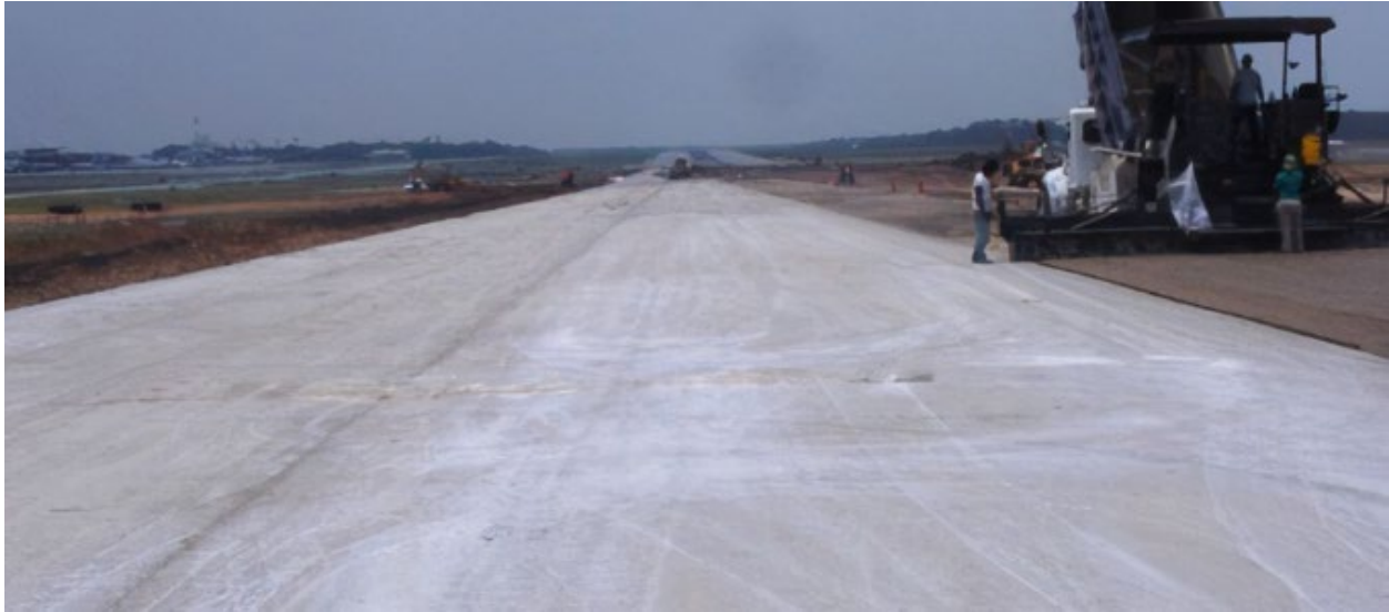
Figure 1. Cement Treated Subgrade
