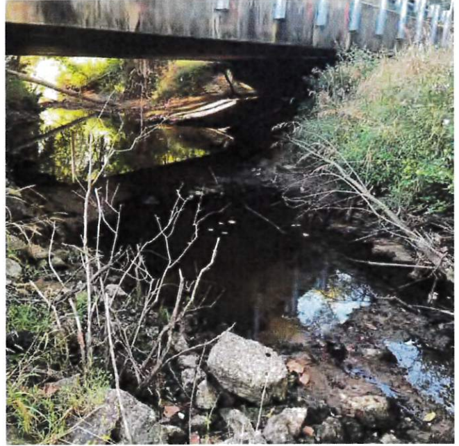
Photo 6: Side view of the SR 58 bridge.
