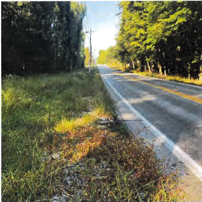
Photo 3: SR 58 just south of the bridge.
