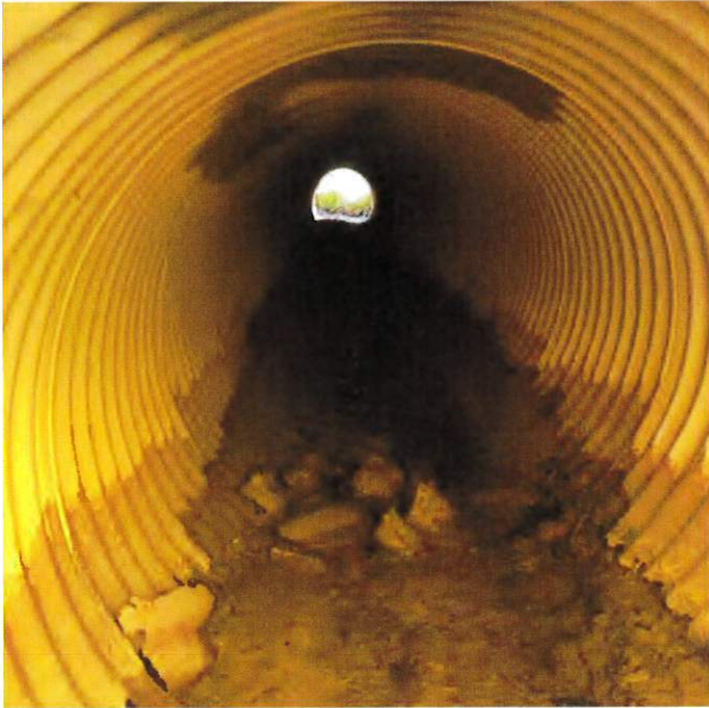
Photo 5: View of inside the corrugated metal pipe.
