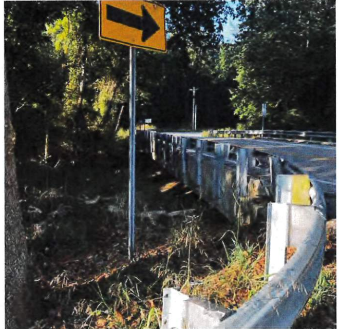
Photo 2: CR 700 looking south at the SR 58 bridge.
