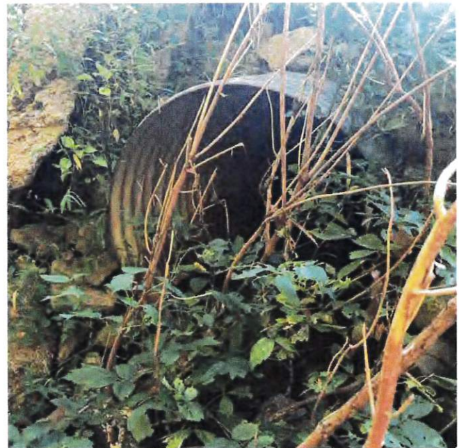
Photo 4: View of the 36-inch corrugated metal pipe.
