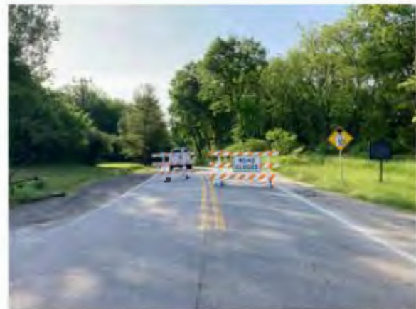
File Description Road Closure Signage northwest of the bridge
