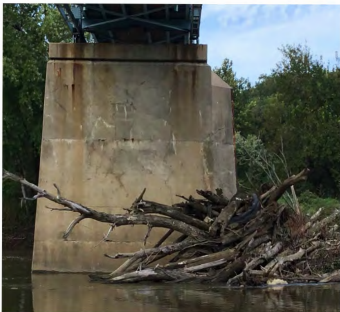
PHOTO 3 Description Looking north at Pier 4
