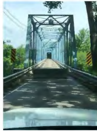
File Description Concrete Barrier at the northwest end of the bridge pic 1 File Type Category CF Closeout
