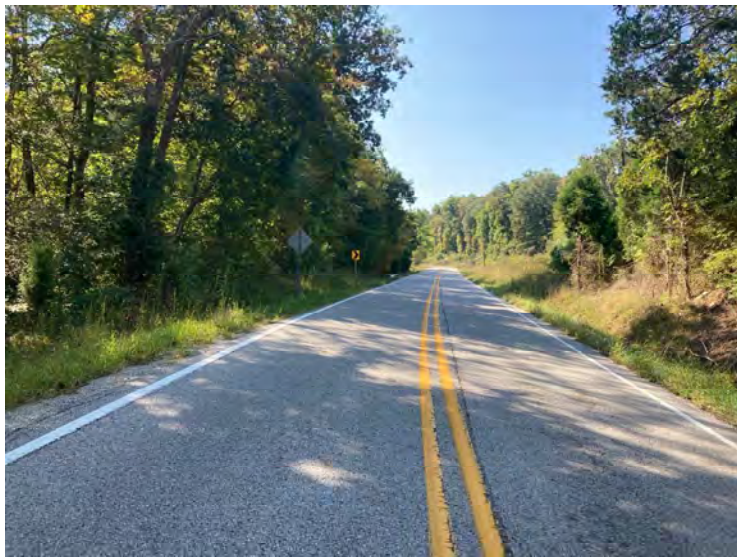
7 – View of survey area facing southwest
