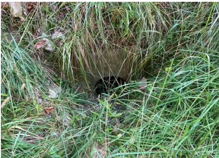
17 – View of 15 inch diameter concrete culvert (CLV-237-013-5.75) inlet facing east
