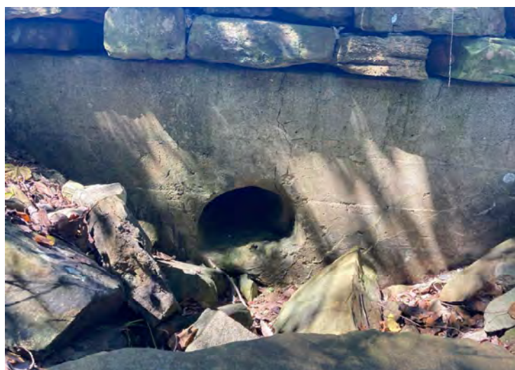
18 – View of 15 inch diameter concrete culvert (CLV-237-013-5.75) outlet facing west
