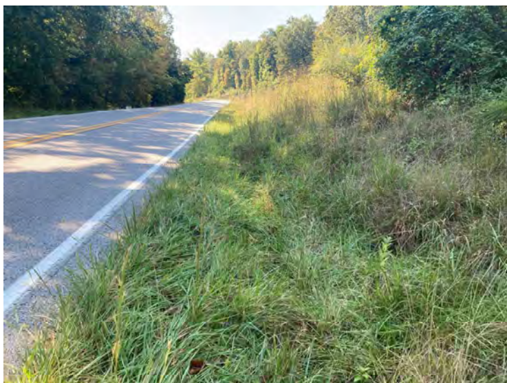
9 – View of RSD1 facing southwest
