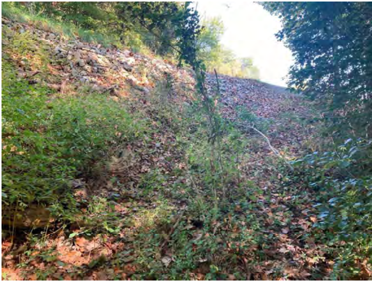
3 – View of SR 237 road embankment facing northwest
