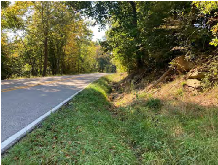
1 – View of RSD1 facing southwest showing roadside grasses, bedrock, and forest
