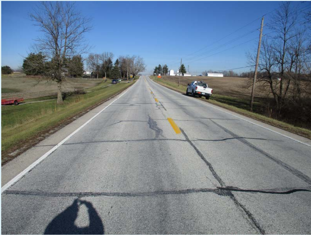
3. View Looking North along SR 3 at small structure
