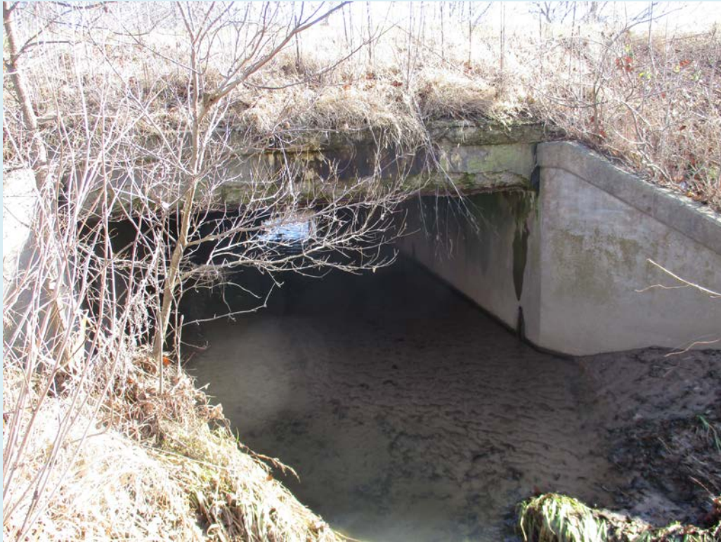
1. View looking East to CV 003-016-6037
