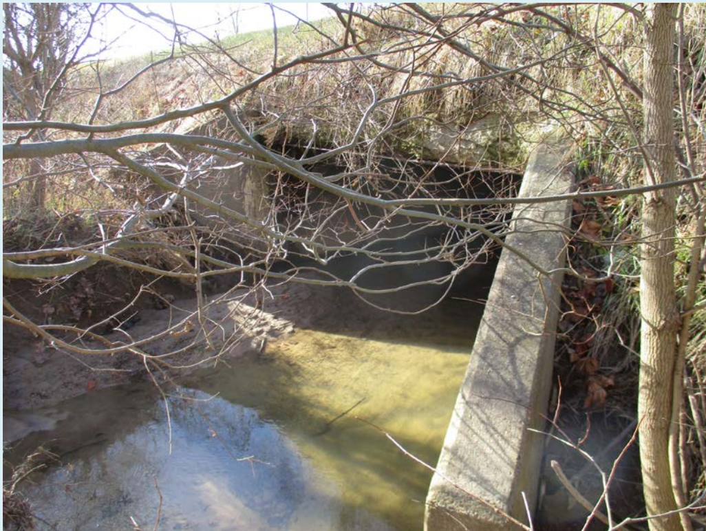
2. View Looking West to CV 003-016-60.37
