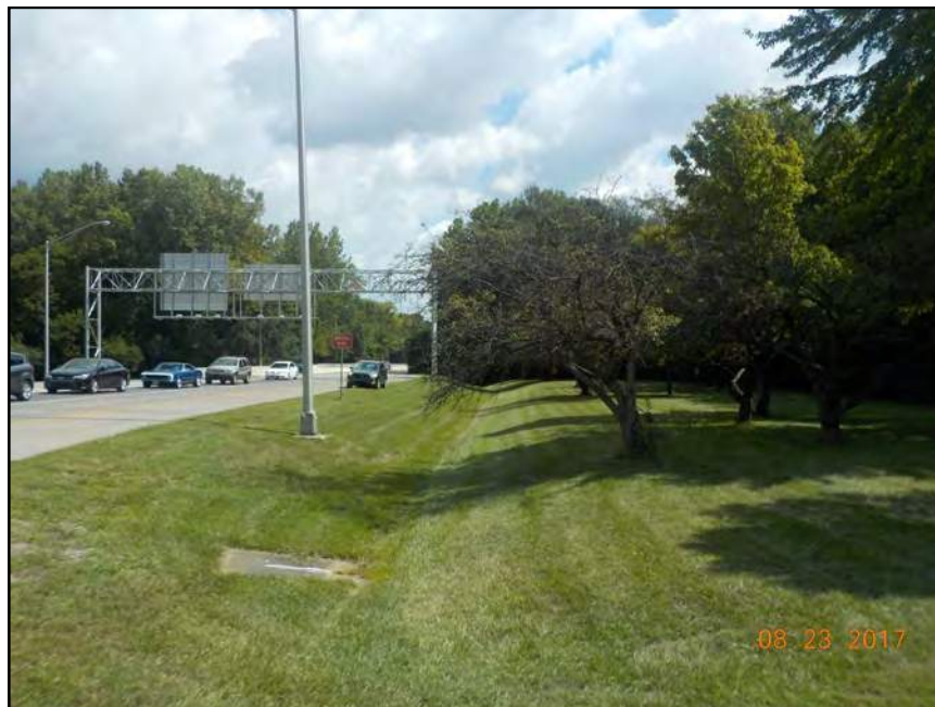
38. View from S.R. 46 interchange looking northeast at S.R. 46 West right-of-way and RSD 4.
