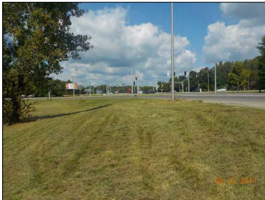
32. View from southern side of S.R. 46 East looking northwest at S.R. 46 interchange.
