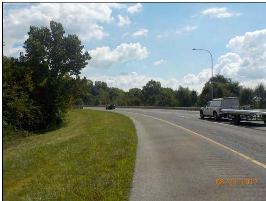
36. View from northern side of S.R. 46 East looking east at S.R. 46.
