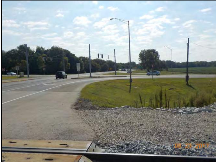
11. View looking east at S.R. 46 interchange with S.R. 11
