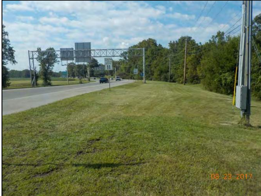
15. View looking south at S.R. 11 right-of-way.
