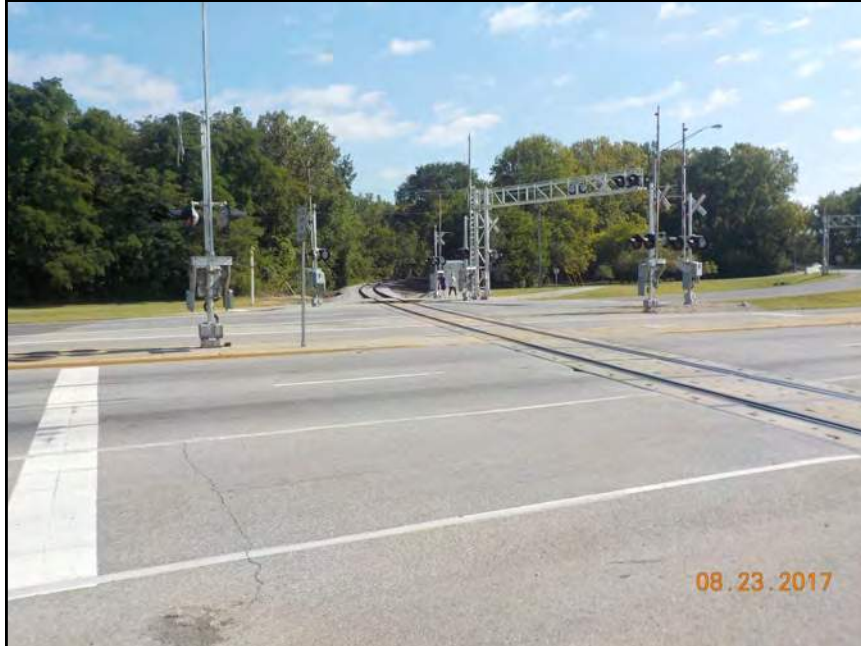
9. View looking northeast at intersection of S.R. 46 at railroad.
