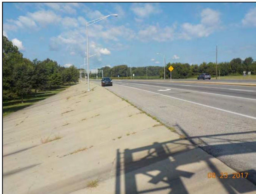
8. View looking west at S.R. 46.
