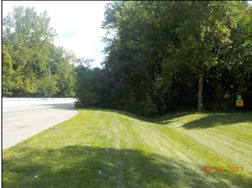
35. View from southern side of S.R. 46 West looking northeast at S.R. 46 right-of-way and RSD 4.
