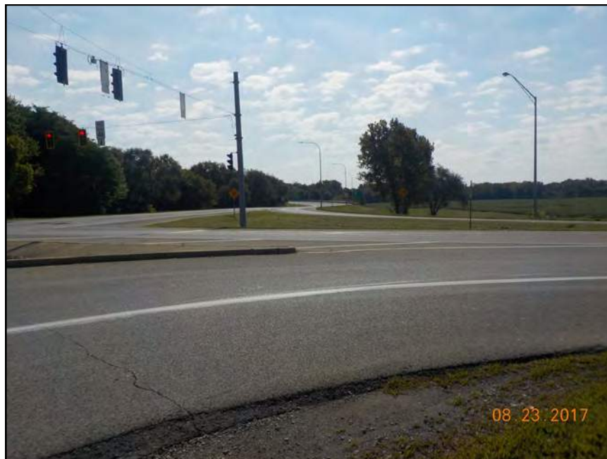
14. View looking east at S.R. 46 interchange with S.R. 11.
