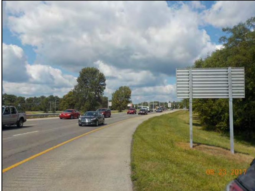
37. View from northern side of S.R. 46 East looking west at S.R. 46.
