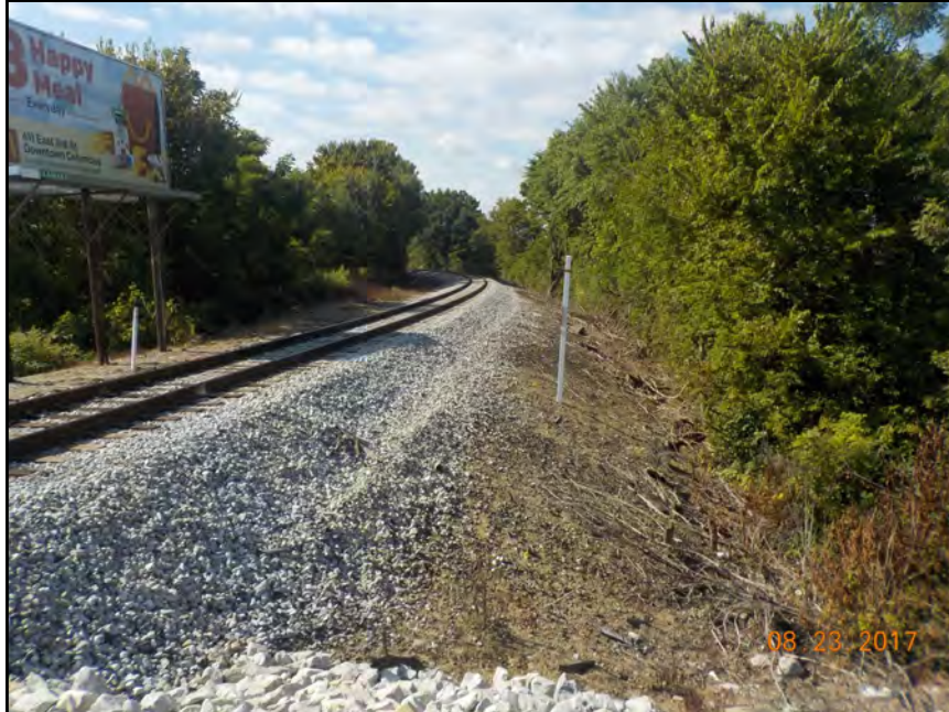
7. View west of S.R. 11 looking southwest at railroad tracks.
