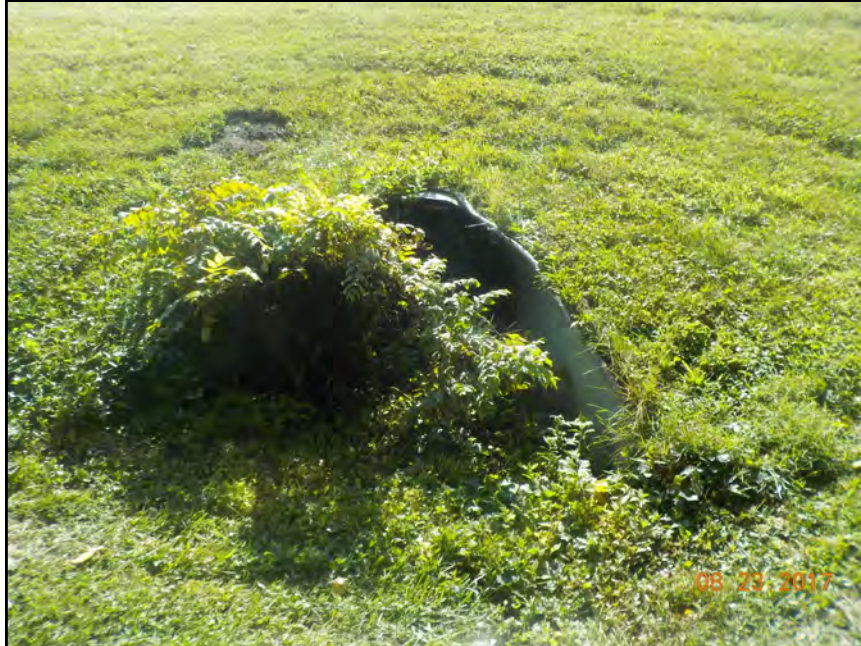
69. View of Culvert on western side of S.R. 11 looking southeast.
