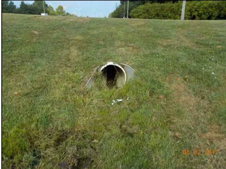
65. View of culvert draining into RSD 1.
