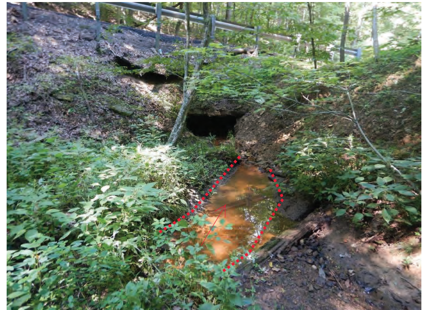
Photo 12: Within UNT 1/Wetland 1 to Tipton Creek Facing Northeast Towards Structure on Southside of SR 58
