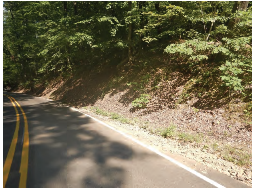
Photo 26: Facing Northeast Along SR 58 ROW
