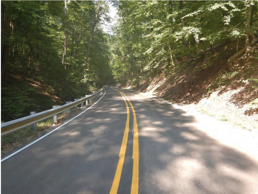
Photo 25: Facing Northeast Along SR 58 Towards Eastern Termini
