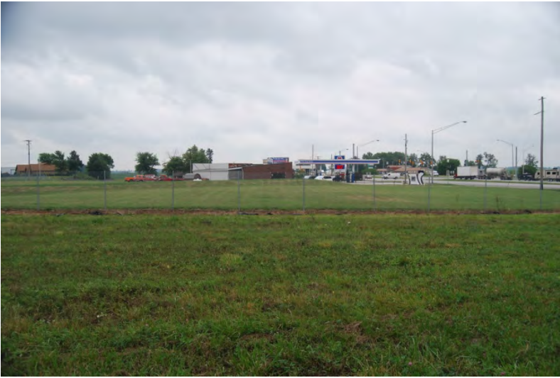
065 – View S from middle stormwater basin.
