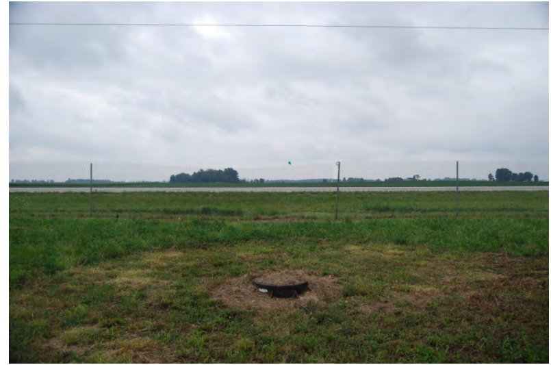
070 – View S from S stormwater basin, showing stormwater standpipe/overflow.
