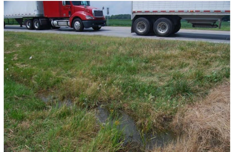
140 – View N of S ditch of SR 28, just W of interchange.
