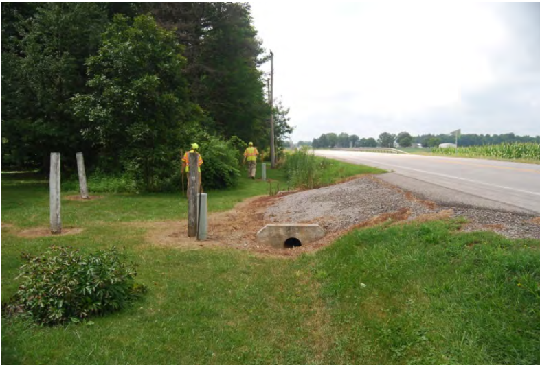
103 – View W of S ditch leading to Dixon Cr at SR 28.
