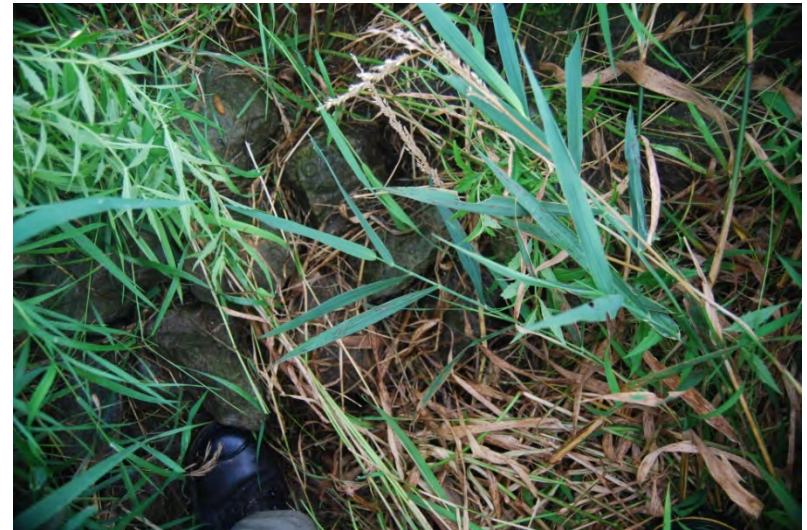
024 – View of SW ditch riprap bottom.
