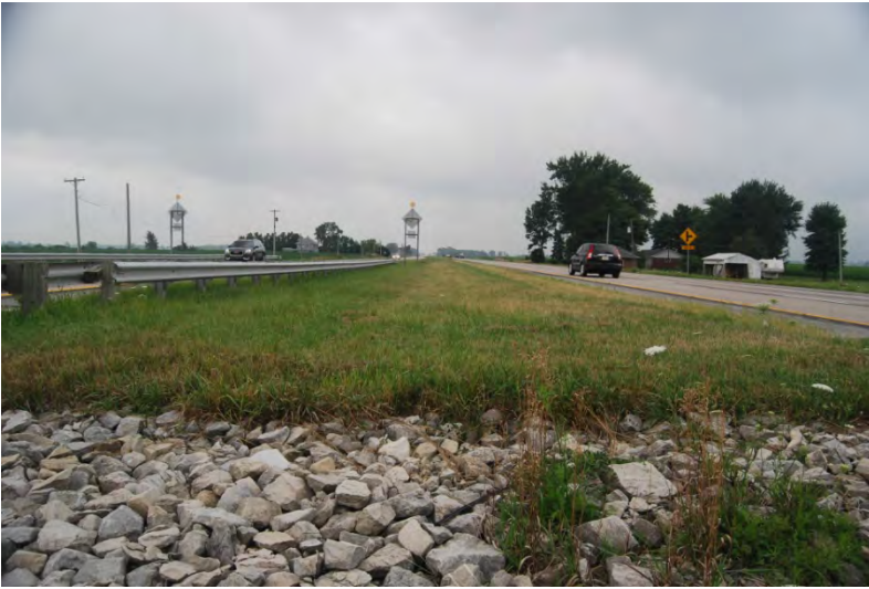
025 – View S from Dixon Cr from between SB and NB US 31.
