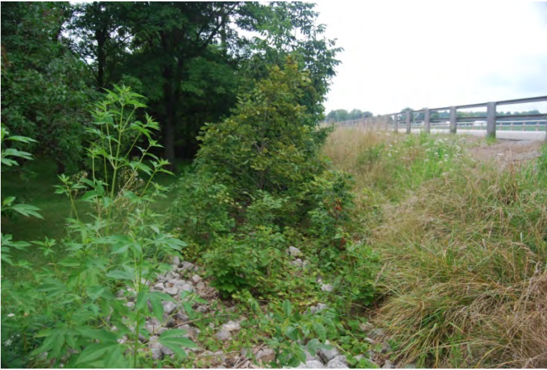
105 – View W of S ditch before entering Dixon Cr at SR 28
