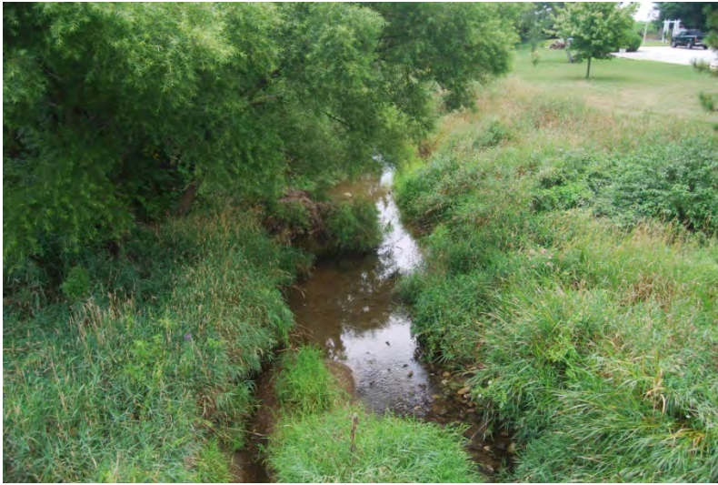
109 - View S of Dixon Cr at SR 28 from bridge.
