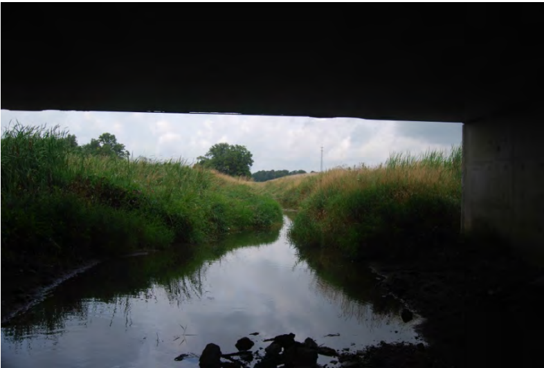
115 – View N of Dixon Cr at SR 28 from under bridge.
