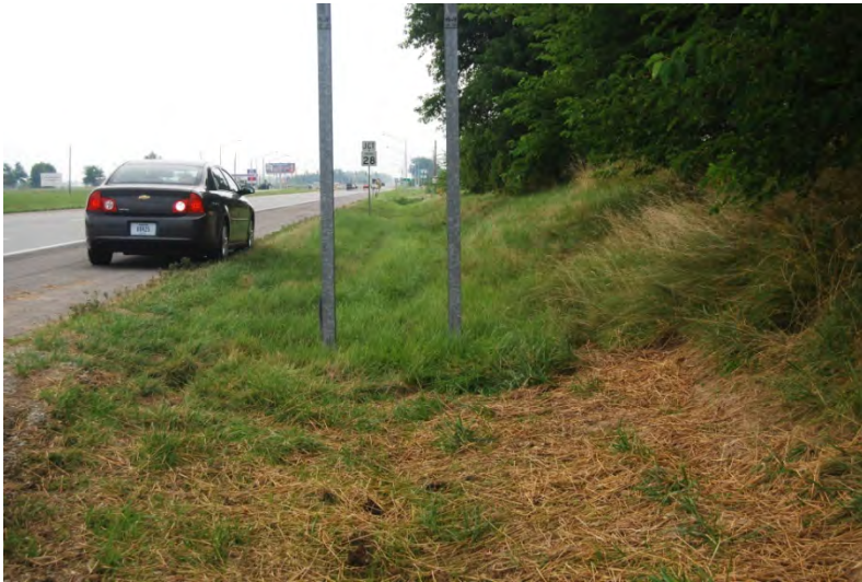
087 – View of W ditch on SB US 31, north of the interchange.
