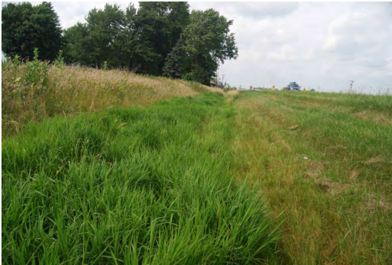
175 – View N of Roadside Ditch H.
