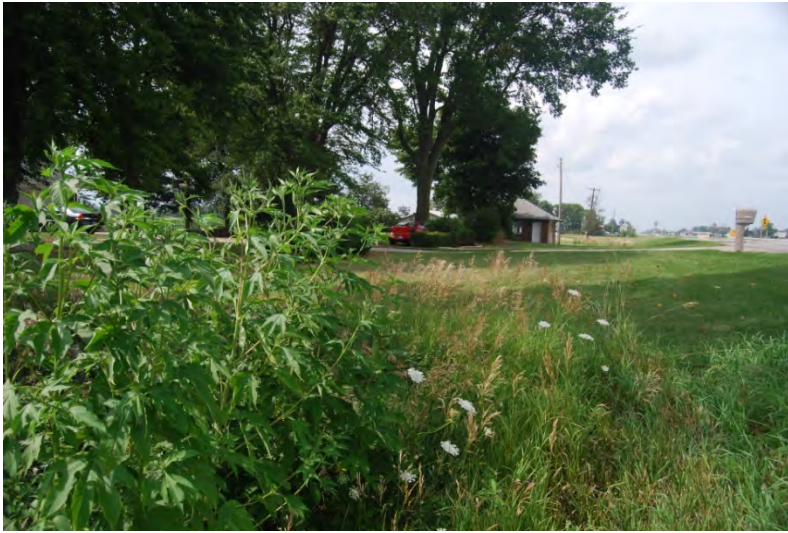
173 – View N of Roadside Ditch H where pipe outlets to out from residential property.
