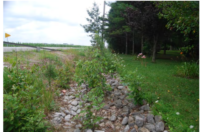
104 – View E of S ditch before entering Dixon Cr at SR 28.
