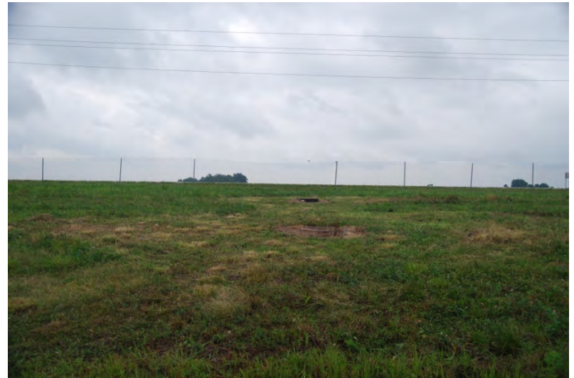
068 – View S from S stormwater basin.
