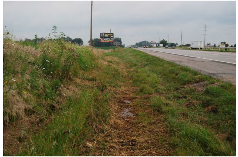
086 – View of W ditch on SB US 31, north of the interchange.
