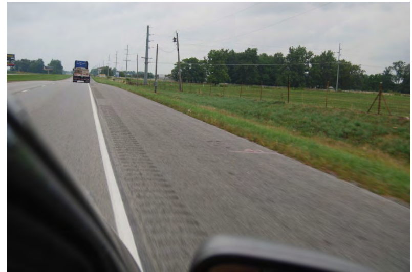
072 – View W along SR 28 north ditch.
