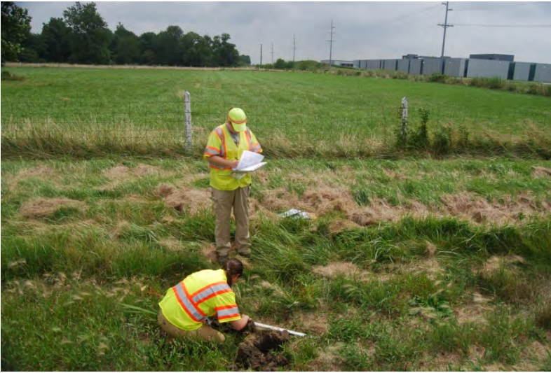
077 – View E of Roadside Ditch C from soil point C1.
