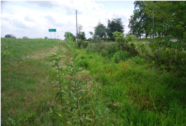
151 – View S at Roadside Ditch G.
