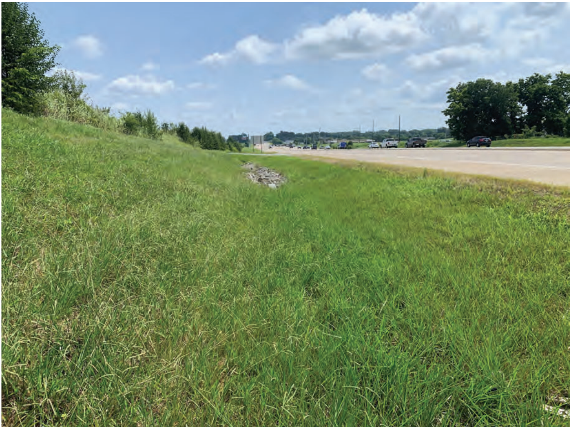
18. Looking east along westbound SR 66 (08/10/21)
