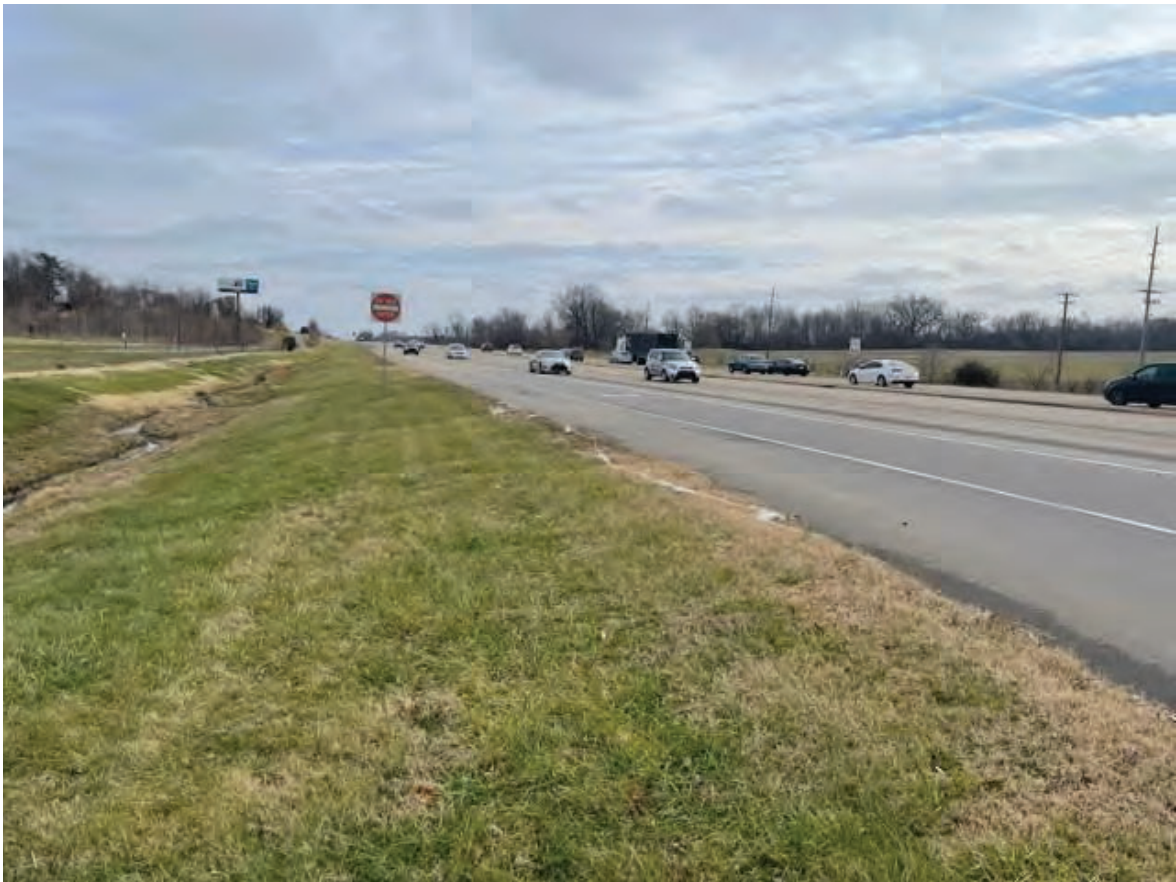
16. Looking east along westbound SR 66 (12/29/21)
