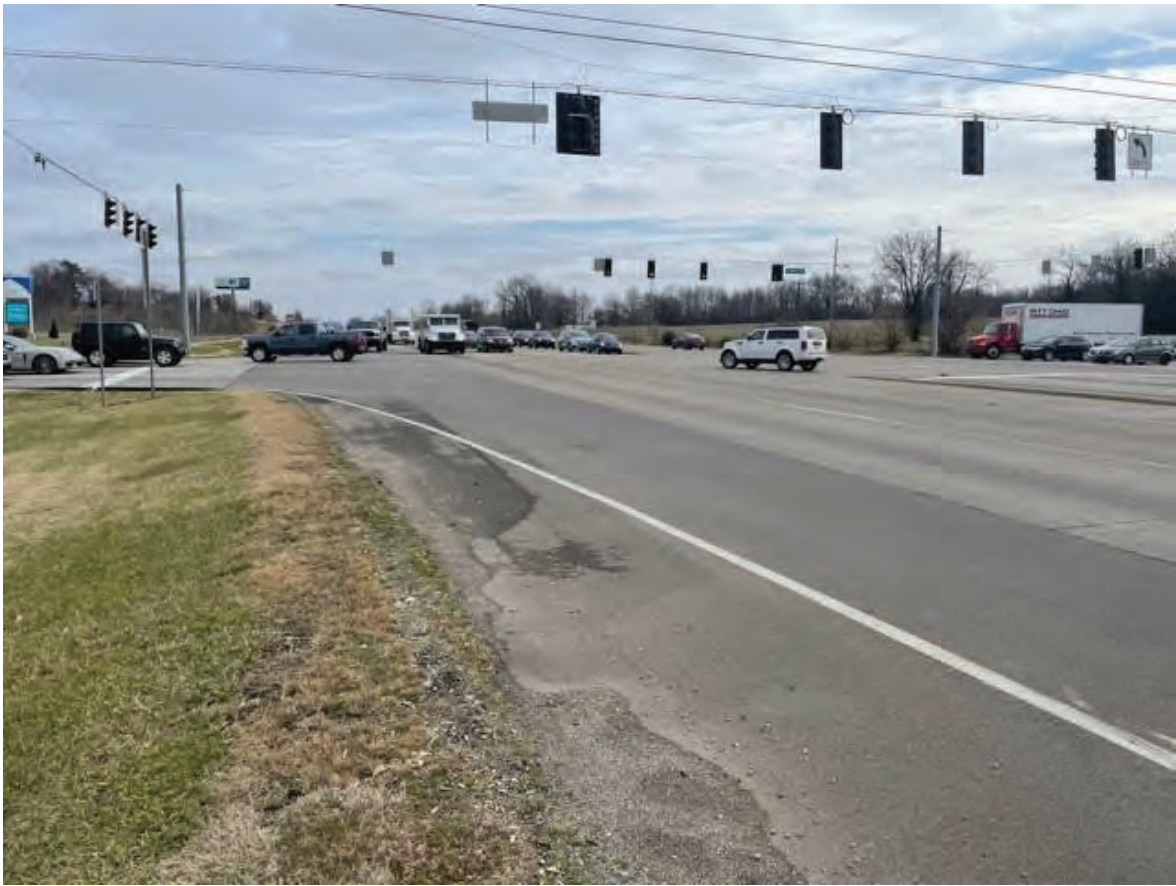
5. Looking east at SR 66/Epworth Rd intersection (12/29/21)
