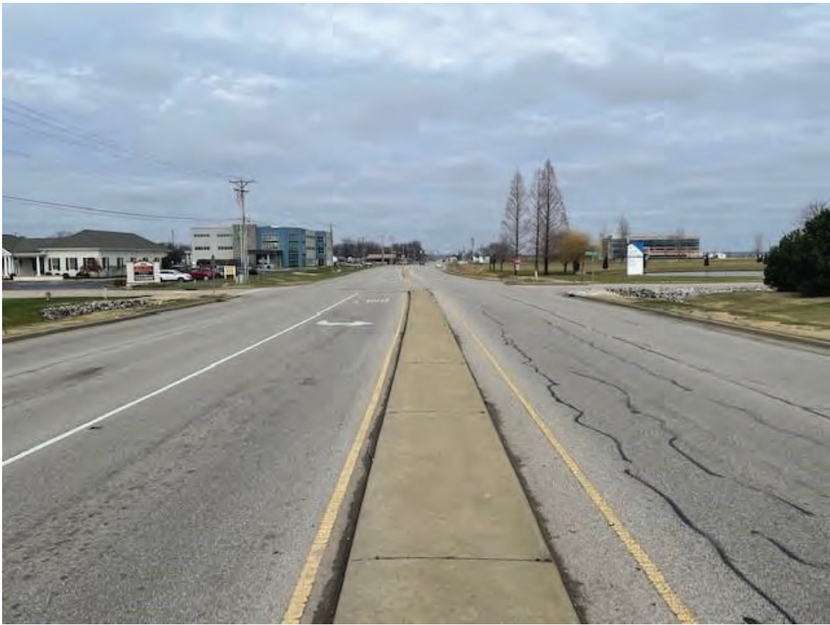
11. Looking north along Epworth Rd (12/29/21)
