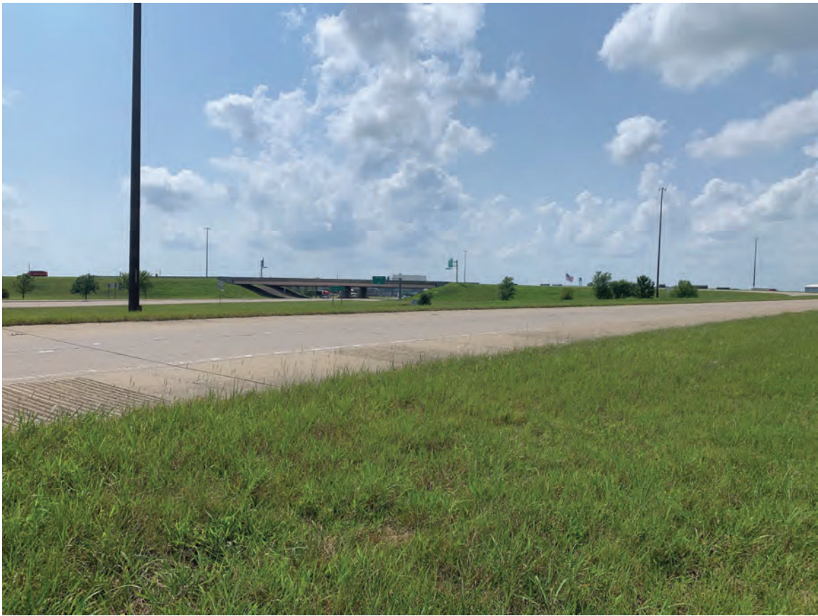
3. Looking southwest across the SR 66 W to I-69 N entrance ramp (08/10/21)
