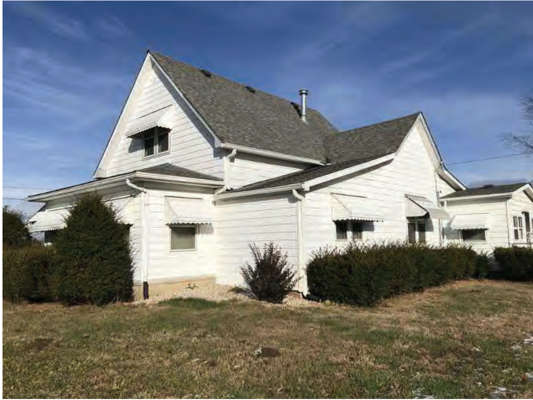
32. Facing northeast toward non-contributing residential building at 667 S. Nineveh Rd
