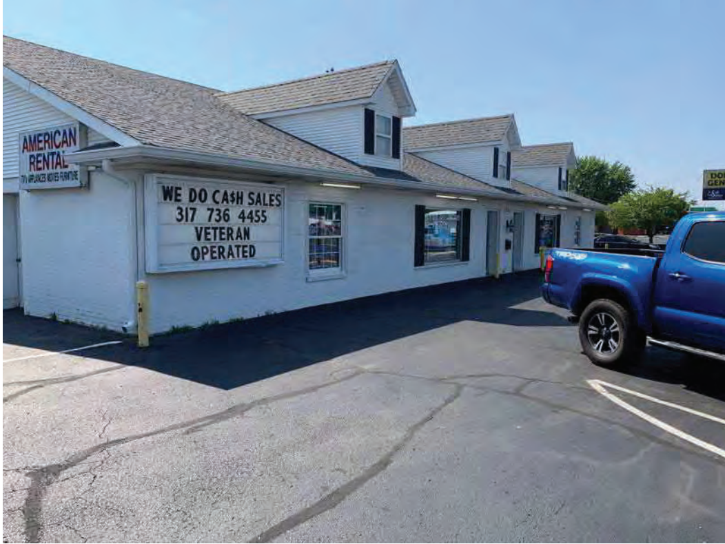
21. Facing southeast toward non-contributing commercial building at 201 N. Morton Street
