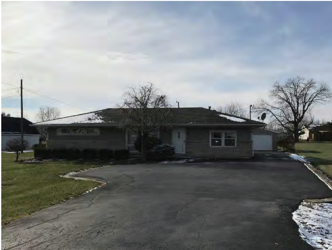
4. Facing west toward non-contributing residential building at 2820 N. Morton Street (US 31)
