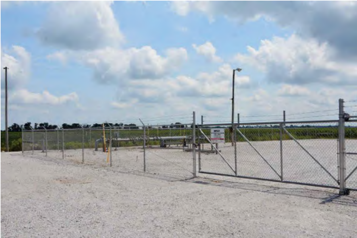
8. The NIPSCO utility station has no above-ground structures, looking southeast.
