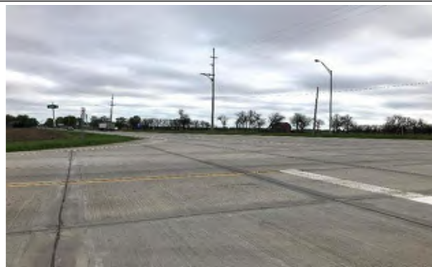
Photo 13. Looking northeast toward the US 6 and US 421 intersection.
