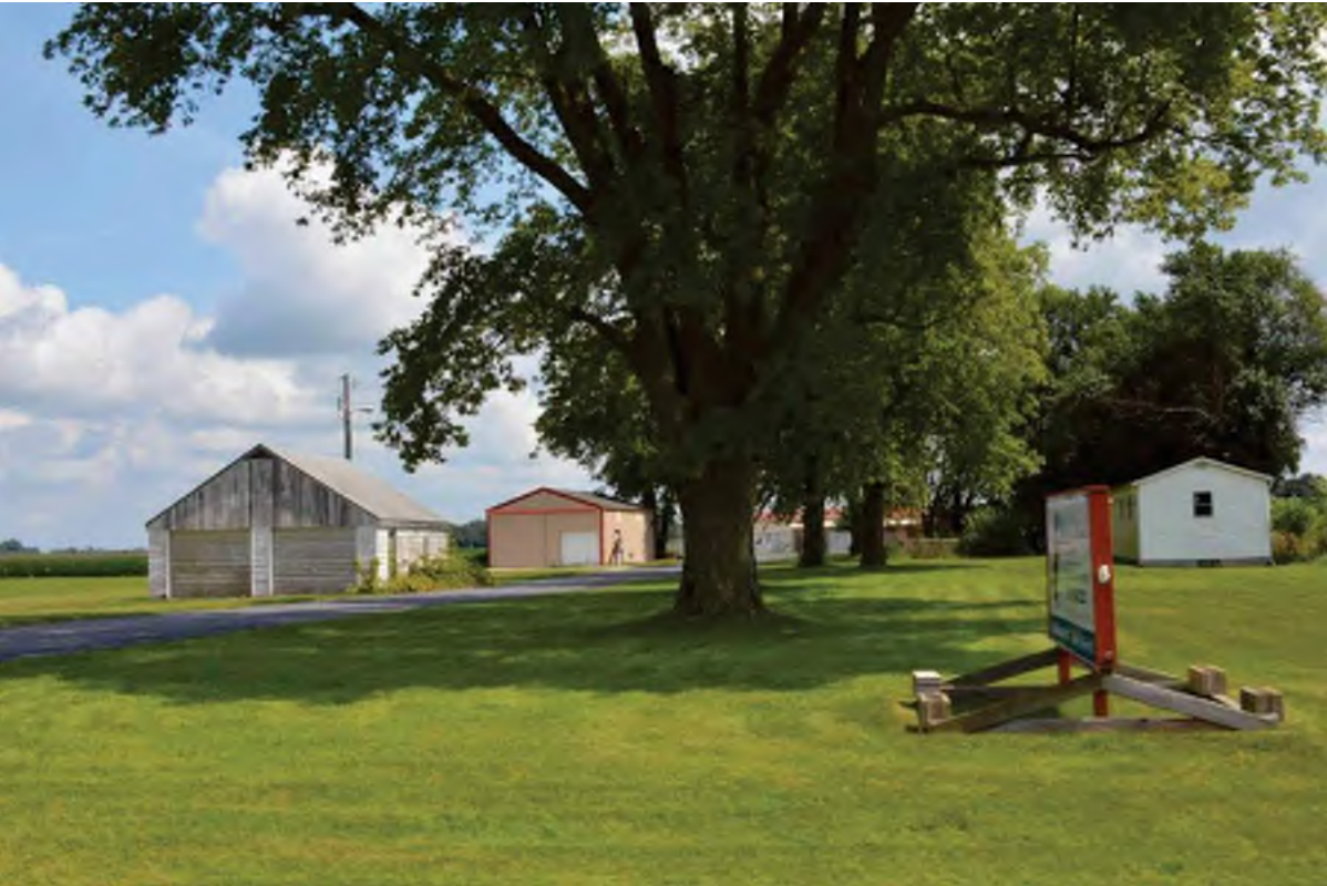
2. The Bed & Biscuit pet resort at 5701 US 421 has a collection of buildings that mostly date to the 2000s, looking east.
