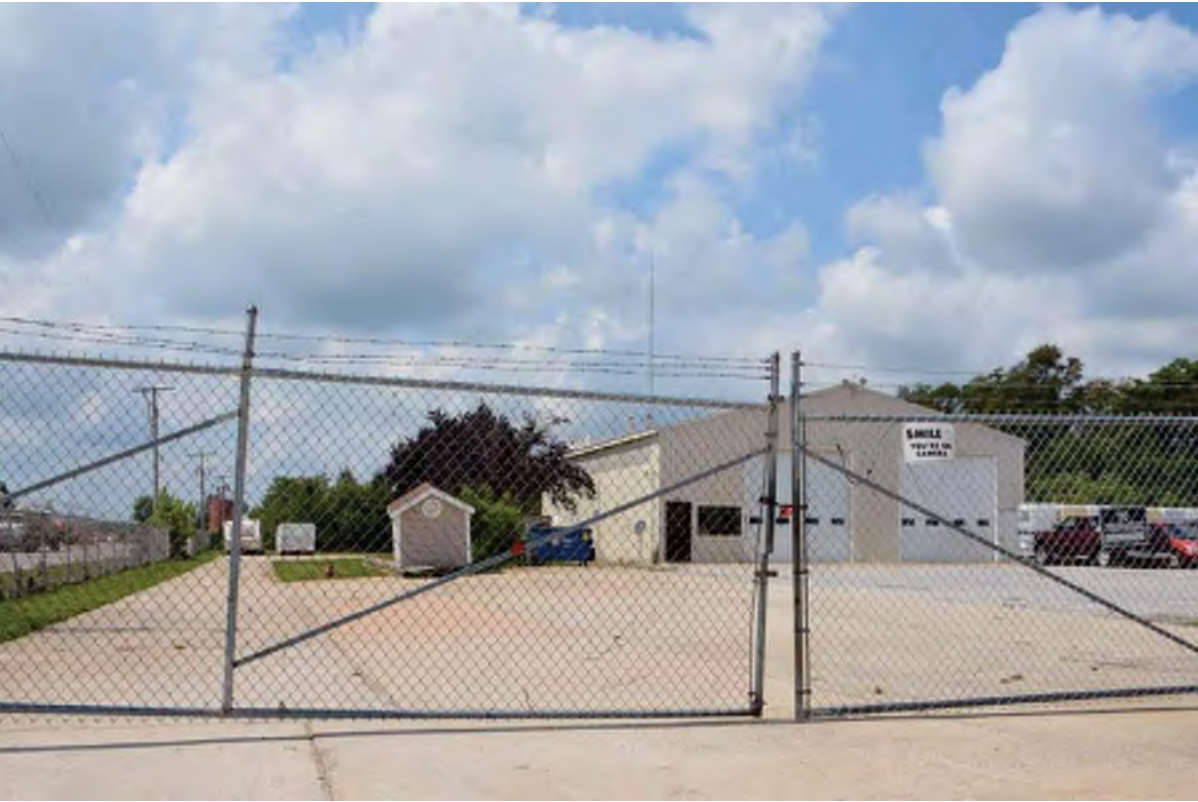
1. The commercial garage at 5606 US 421 (c. 1973) is a Non-Contributing resource in the northern APE, looking north.
