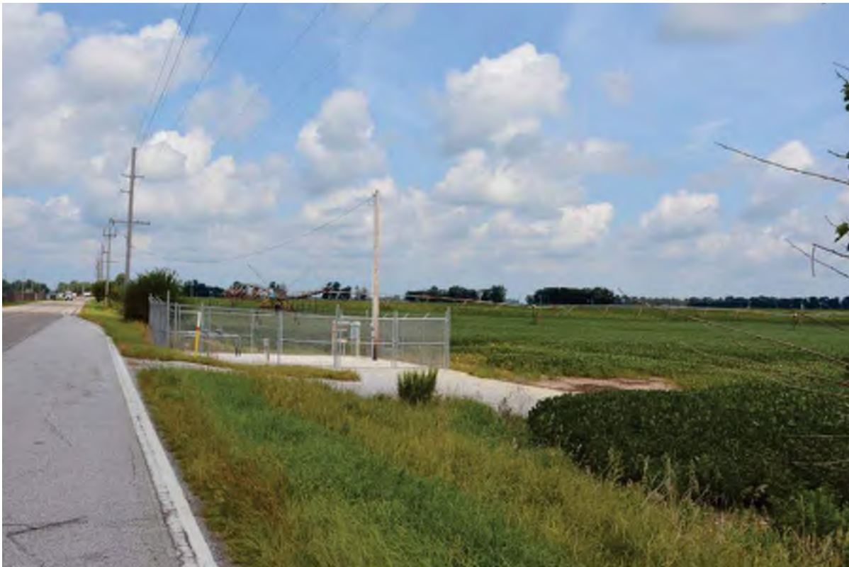
10. Irrigation equipment and utility facilities line US 421 at the south end of the APE, looking north-northeast.
