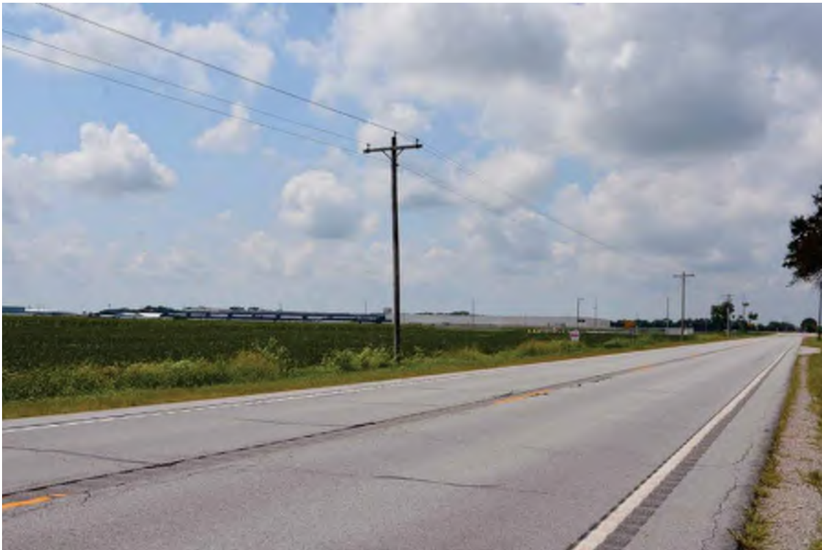
9. The sprawling Dollar General Stores distribution center (c. 1975) can be seen across agricultural fields from the east end of the APE, looking southwest.
