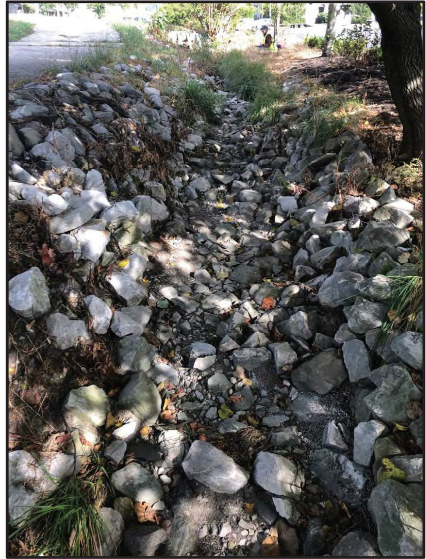
2. View of UNT looking east (upstream). 10/1/2020
