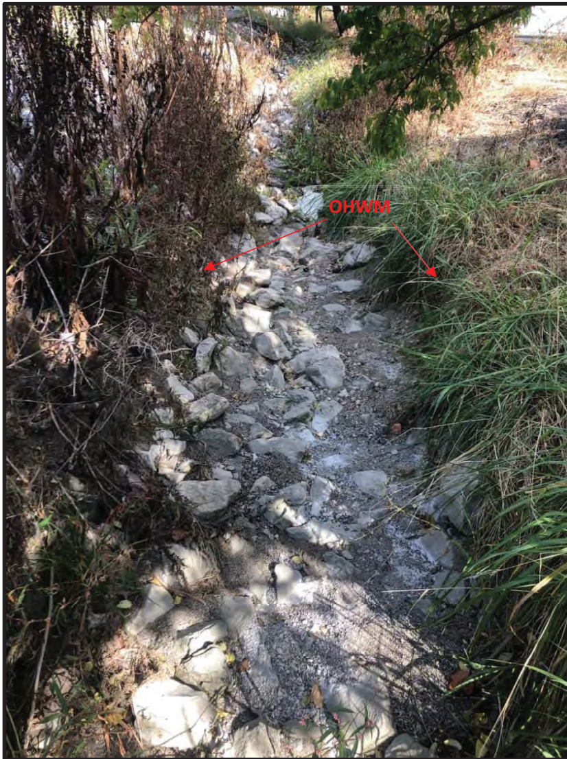
3. View of UNT looking east (upstream). 10/1/2020
