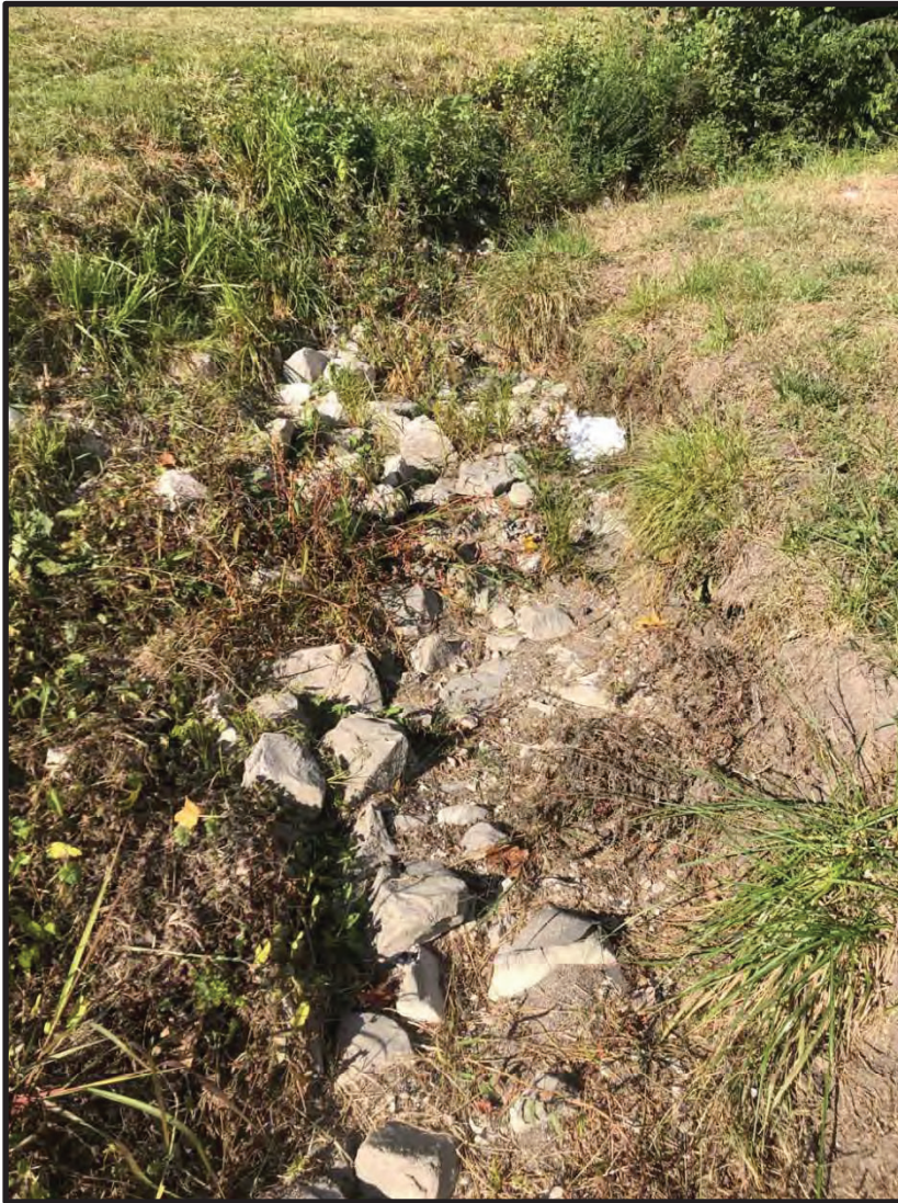
5. View of UNT looking north (upstream). 10/1/2020
