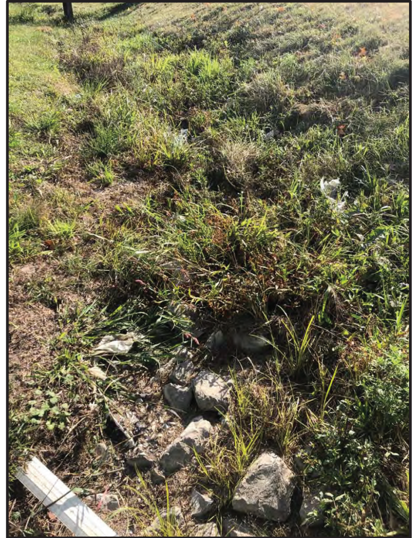
6. View of UNT looking south (downstream). 10/1/2020
