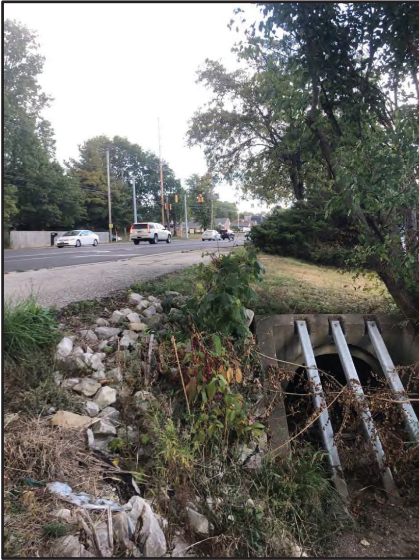
1. View existing culvert outlet to UNT looking east (upstream). 10/1/2020
