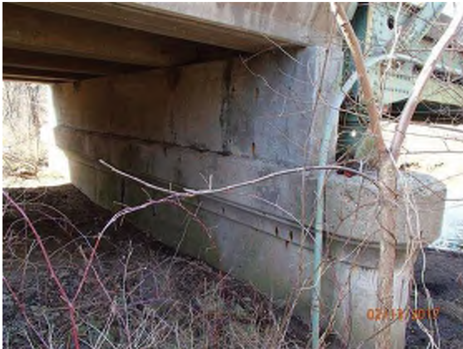
PHOTO 8 Condition Description 02-13-2017 (421)39-12-01792 B Pier 2 south face condition
