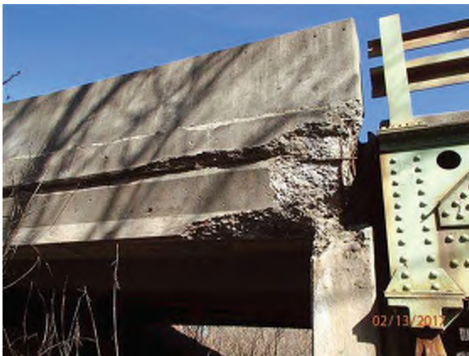
PHOTO 34 Condition Description 02-13-2017 (421)39-12-01792 B Span C beam 1 above pier 3 condition
