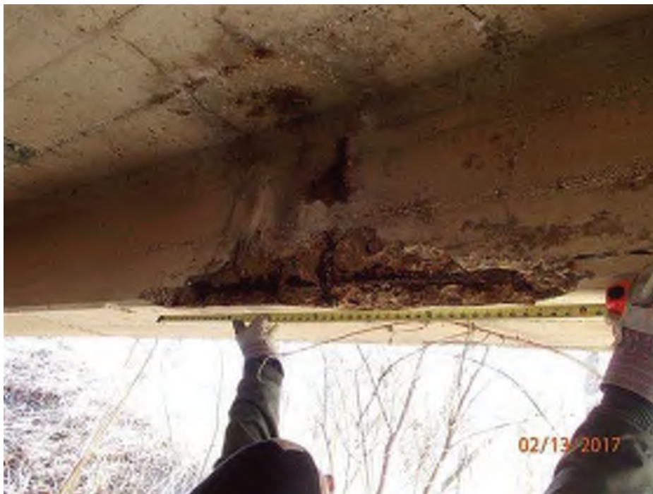
PHOTO 19 Condition Description 02-13-2017 (421)39-12-01792 B Span A beam 1 condition
