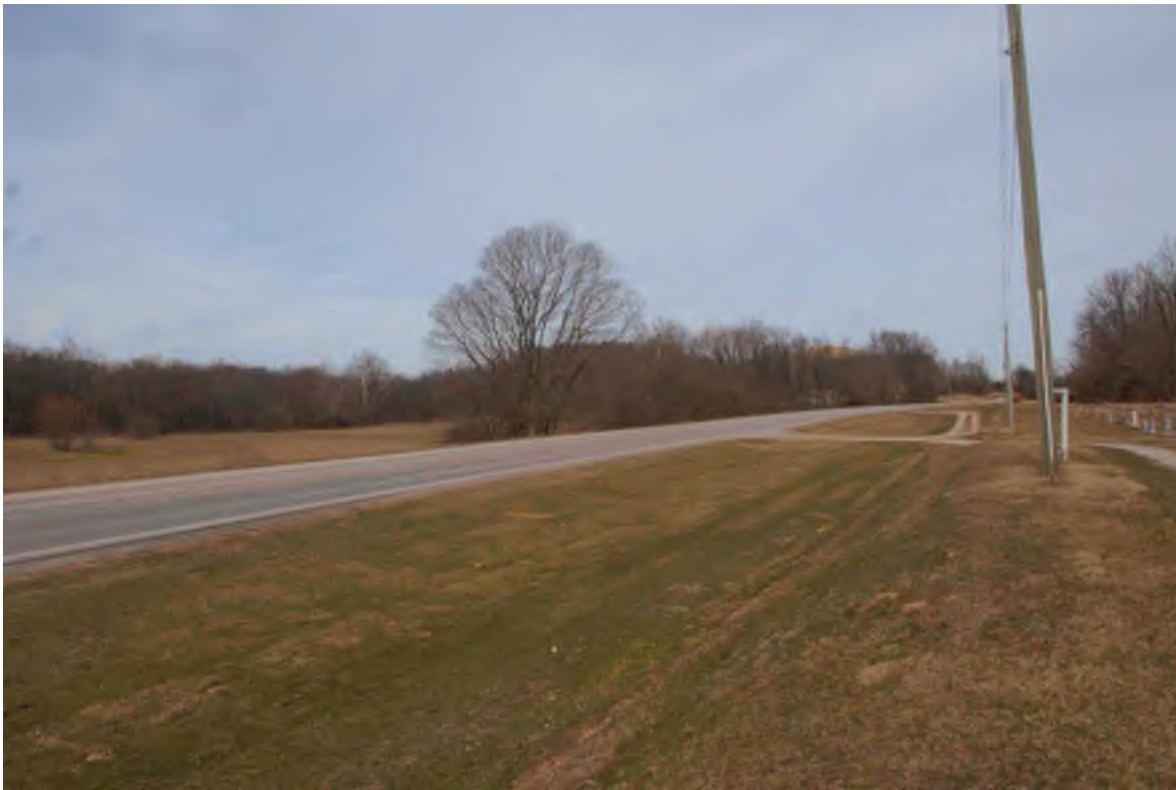
1. Looking north-northwest to the end of the APE along US 421
