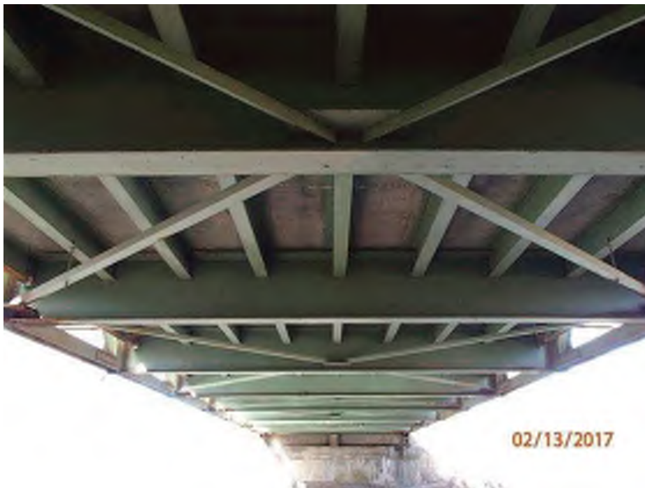
PHOTO 33 Condition Description 02-13-2017 (421)39-12-01792 B Span B truss span underside condition
