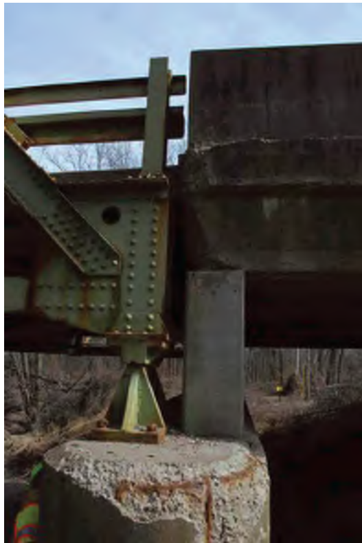
11. The central and approach spans rest on concrete piers
