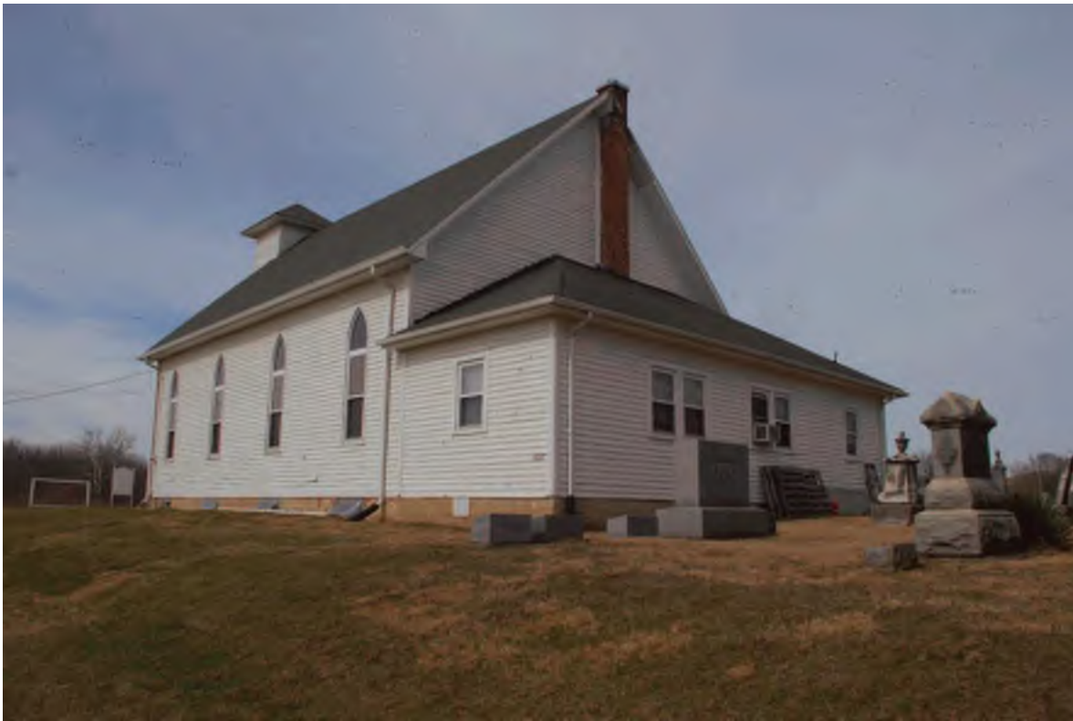
7. A Sunday School addition on the rear of St. Luke's (023-221-30039) was added in the 1920s
