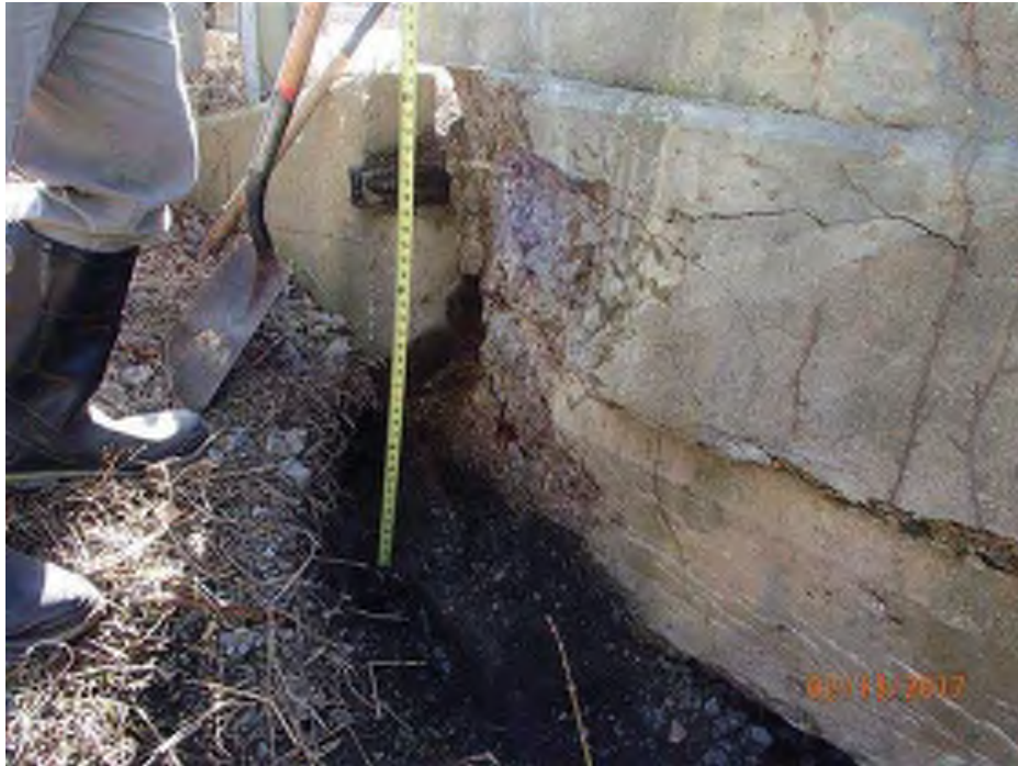
PHOTO 23 Condition Description 02-13-2017 (421)39-12-01792 B Span A beam 5 and coping condition
