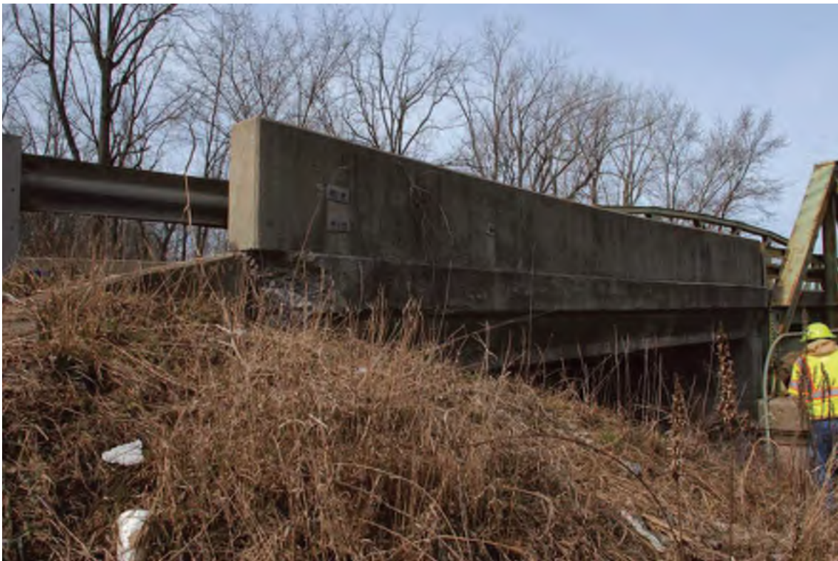
10. Concrete approach spans have modern concrete and w-beam rail
