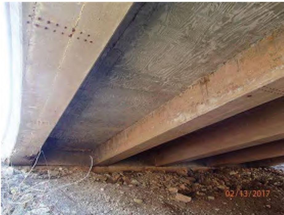
PHOTO 29 Condition Description 02-13-2017 (421)39-12-01792 B Span A deck underside condition
