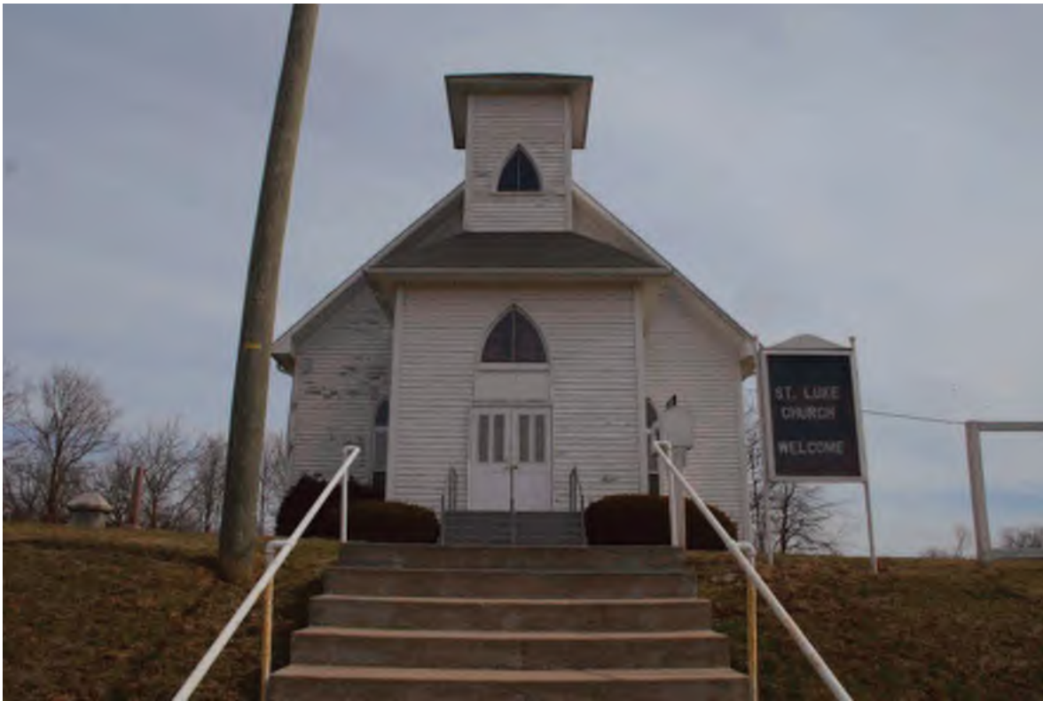
5. The facade (west elevation) of St. Luke's Church (023-221-30039) is on a rise above US 421
