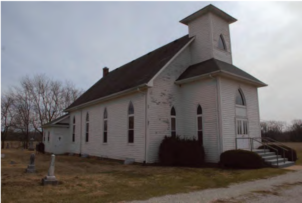
3. View to the west and north elevations of the St. Luke Church (023-221-30039)
