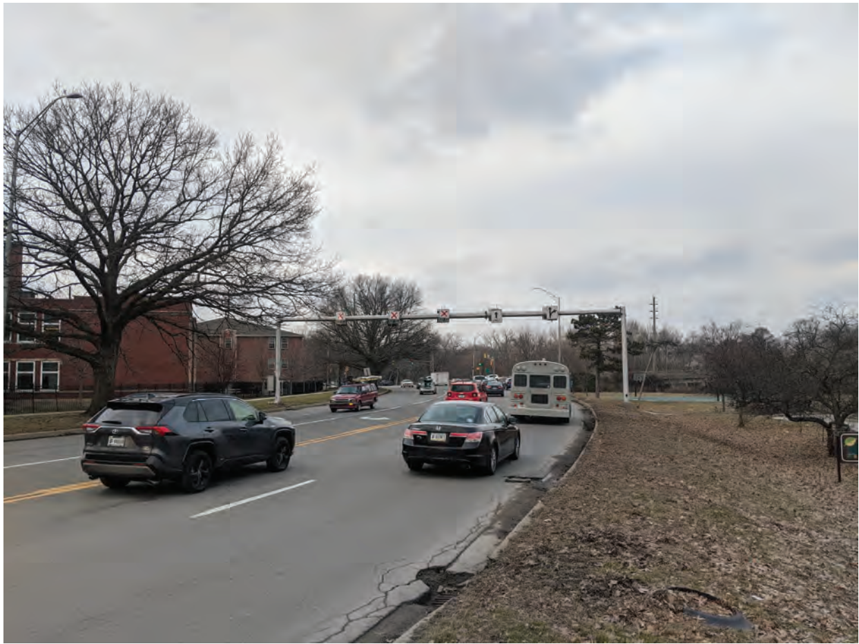
1. Looking north towards 30 th St. along Fall Creek Parkway. Note center left turn lane which will become reversible lane.
