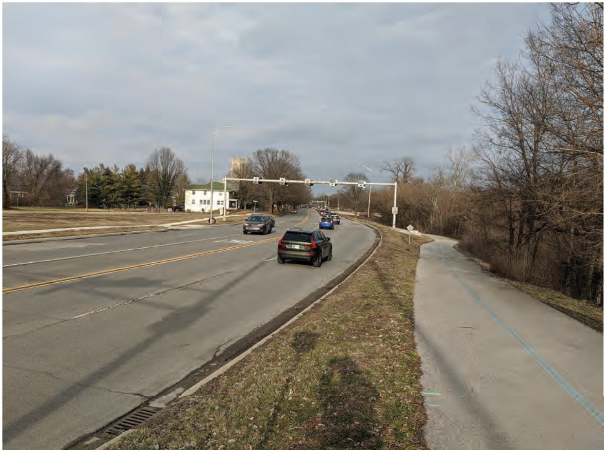
4. Looking northeast along Fall Creek Parkway from Central Avenue. Note center turn lane which will become reversable lane Des. No. 2001151 Appendix B, Page 6 of 15
