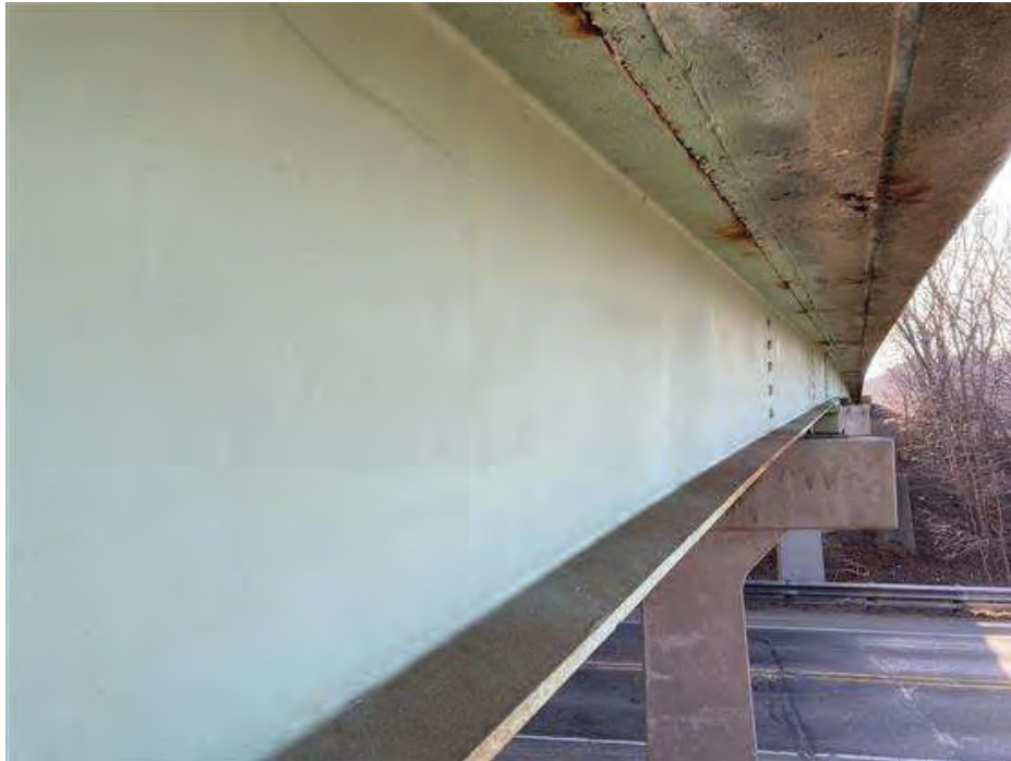
PHOTO 19 Description Along South Fascia (SW corner)
