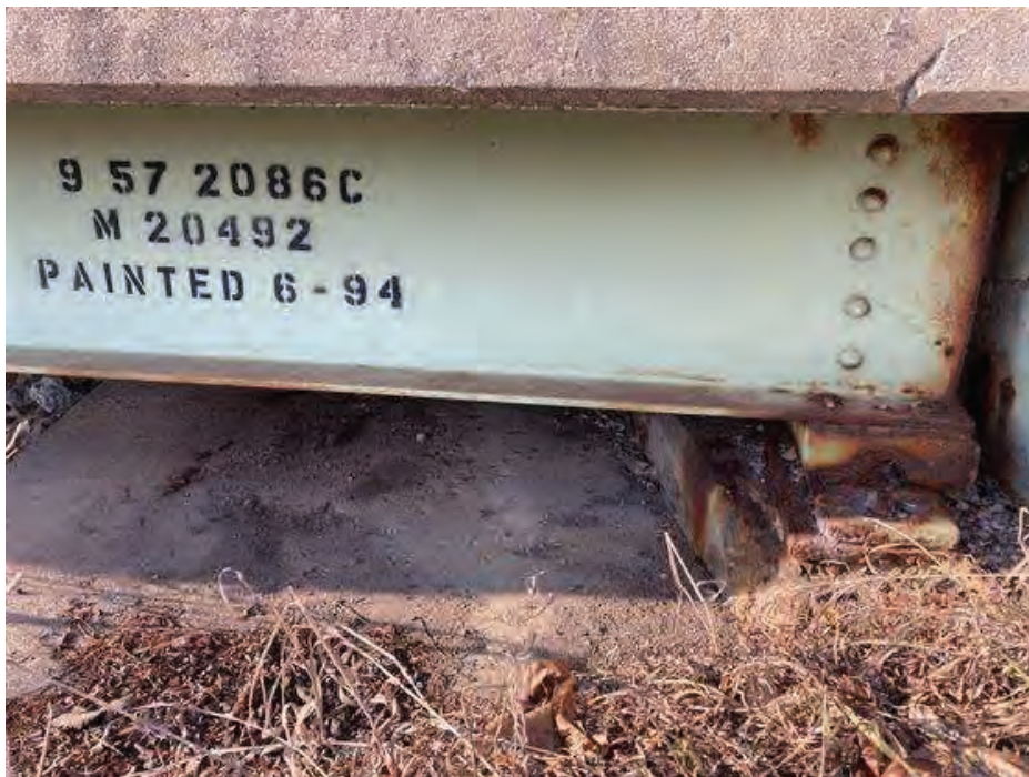
PHOTO 20 Description Abutment 1 (NW Corner)
