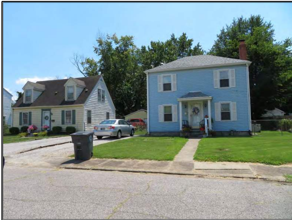
Figure B-24. Overview of Akin Park Historic District (IHSSI No. 163-196-430[01-213]) along Akin Drive, facing southeast.
