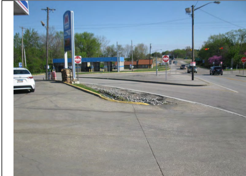
1. Looking S at SR 61 from NE quadrant of SR 61/SR 68 intersection.
