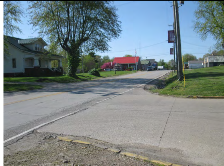
2. Looking NW at SR 61 from NE quadrant of SR 61/SR 68 intersection.
