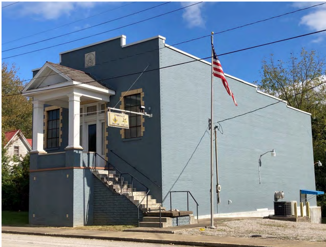
Looking northeast at the Lynnville Masonic Lodge (173-374-06003; “notable”). ROW will be acquired from the existing sidewalk and lawn.
