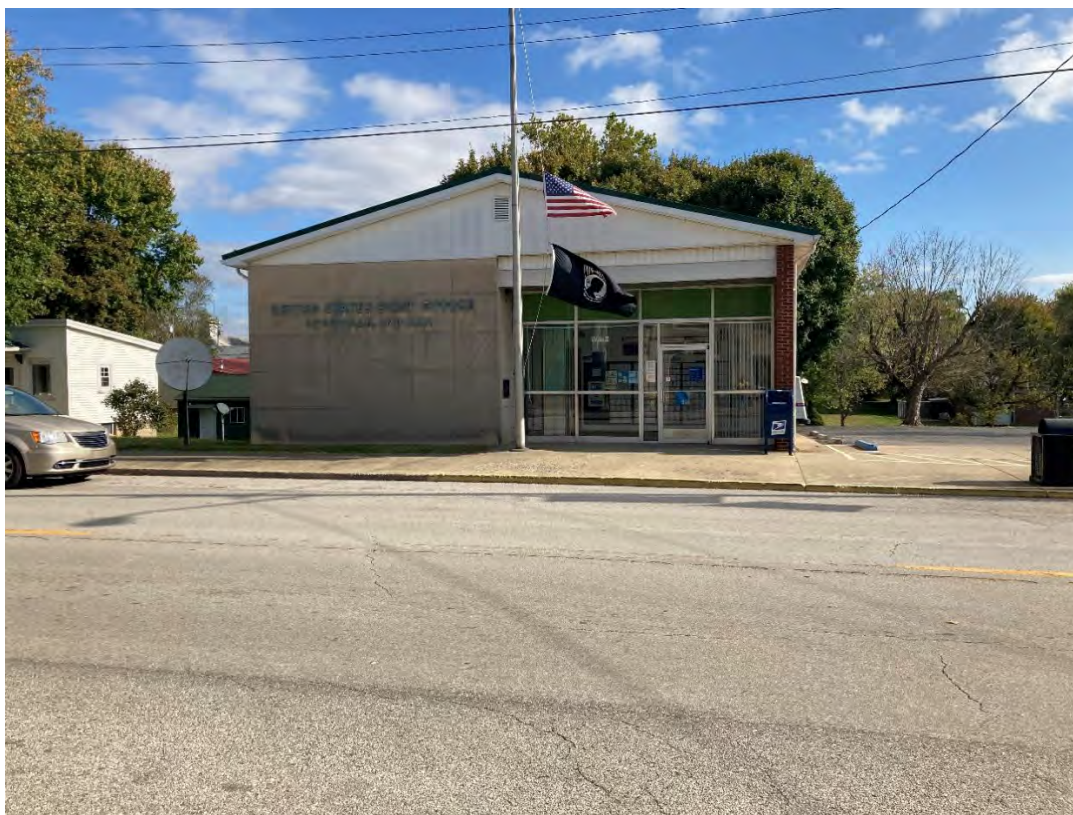
Looking east at the Lynnville Post Office (IHSSI #173-374-06002; notable). The flagpole will be avoided or removed and reset. ROW will be acquired from the existing sidewalk and drive.
