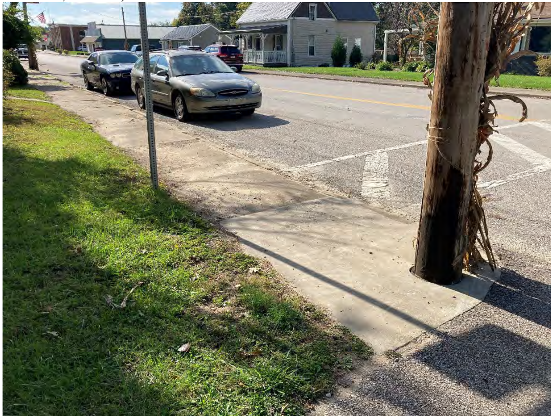
Looking southwest at the southeast corner of SR 61 & 3 rd Street. ROW will be acquired at this corner for the existing sidewalk and a portion of the yard in order to reconstruct the sidewalk, install ADA-compliant curb ramps, and relocate the existing utility pole.
