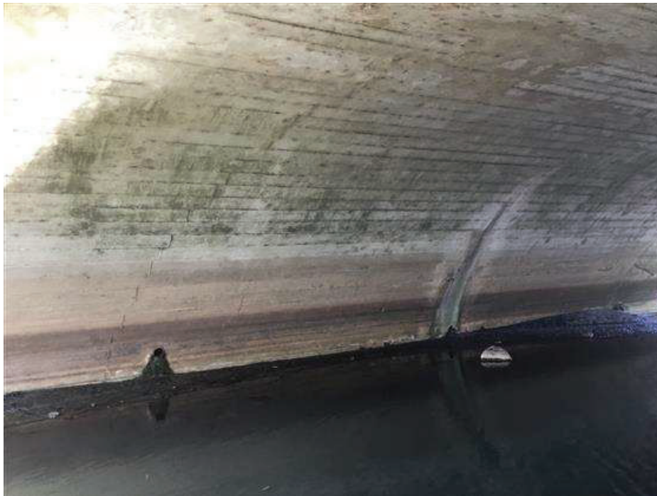
PHOTO 4 Condition Description Abutment 1 looking north west
