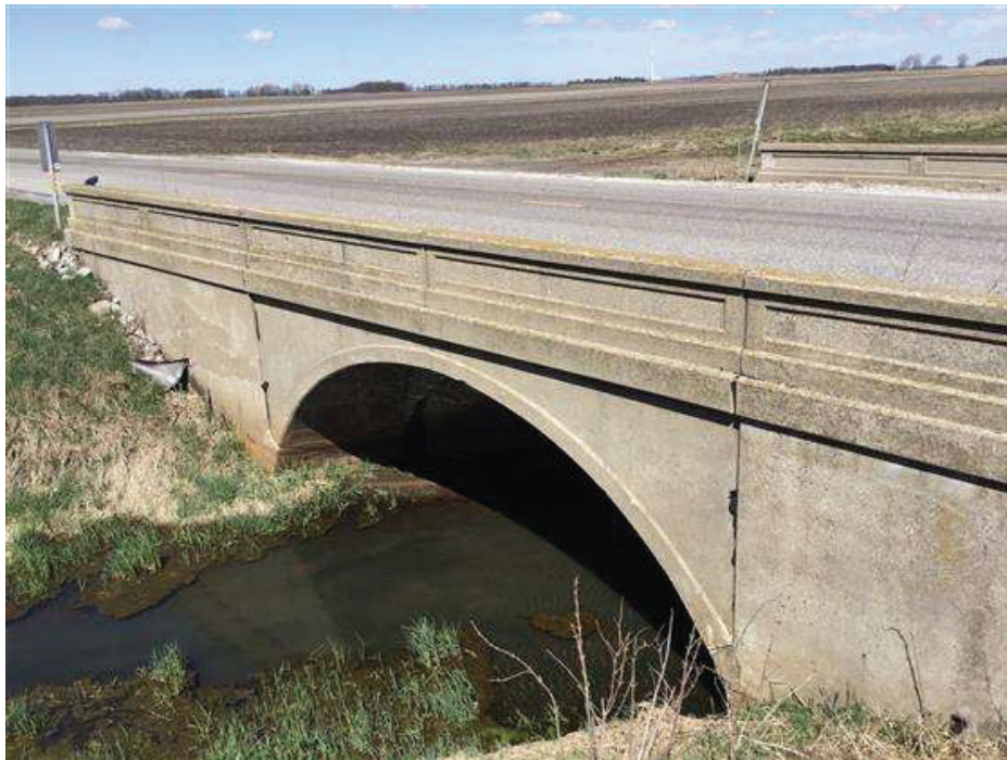
PHOTO 2 Condition Description South profile
