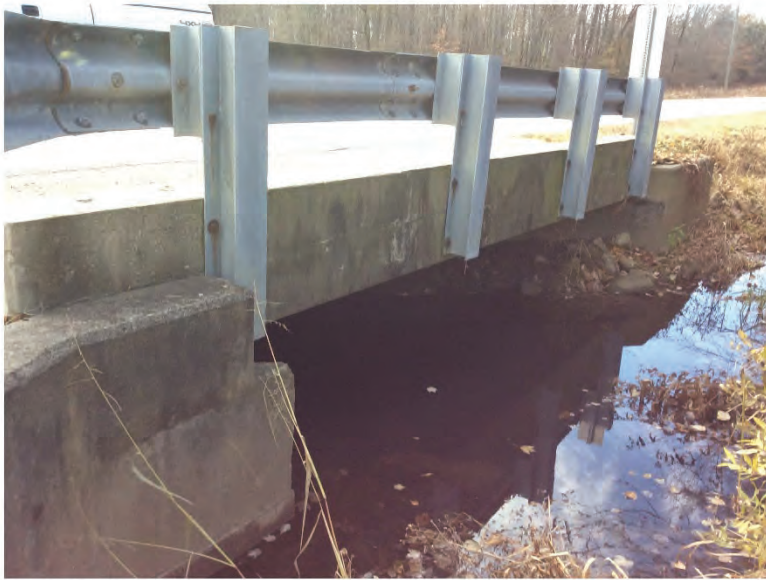
PHOTO 4 Elevation, Condition Description N side, facing SW
