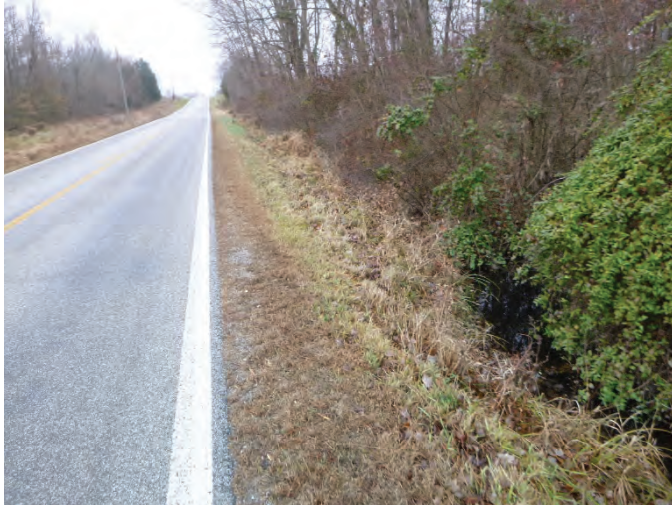
TYPICAL CONDITION OF SHOULDER AT NORTHWEST CORNER OF STRUCTURE
