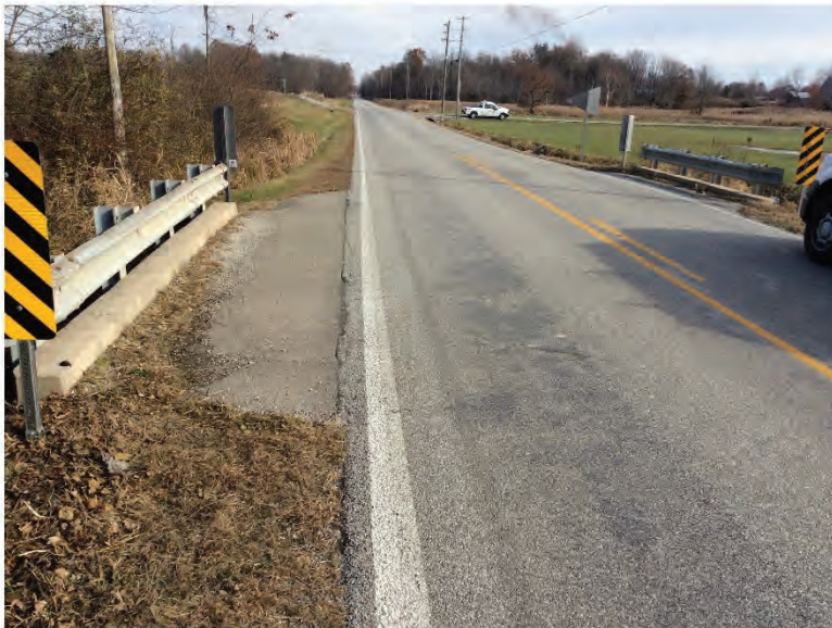
PHOTO 3 Condition Description Roadway facing East
