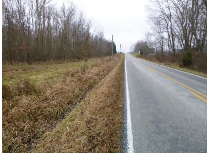
TYPICAL CONDITION OF SHOULDER AT SOUTHWEST CORNER OF STRUCTURE
