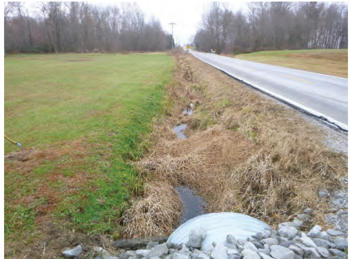
TYPICAL CONDITION OF DOWNSTREAM CHANNEL LOOKING TOWARDS STRUCTURE
