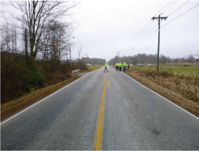
APPROACH LOOKING EAST
