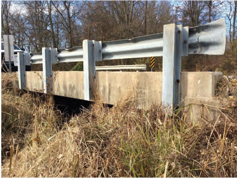
PHOTO 2 Elevation, Condition Description S side, facing NW
