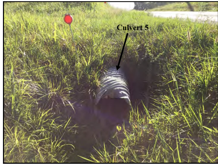
46. View of Culvert 5, looking northeast.
