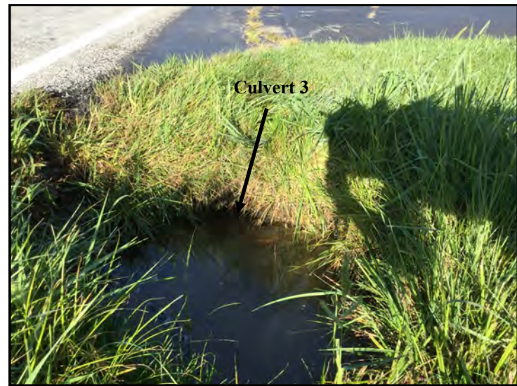
42. View of Culvert 3, looking southwest.
