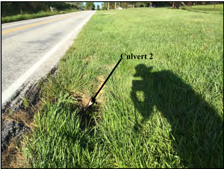
37. View of Culvert 2, looking southwest.
