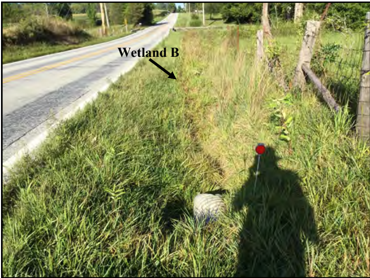
47. View of Wetland B from Culvert 5, looking southwest.
