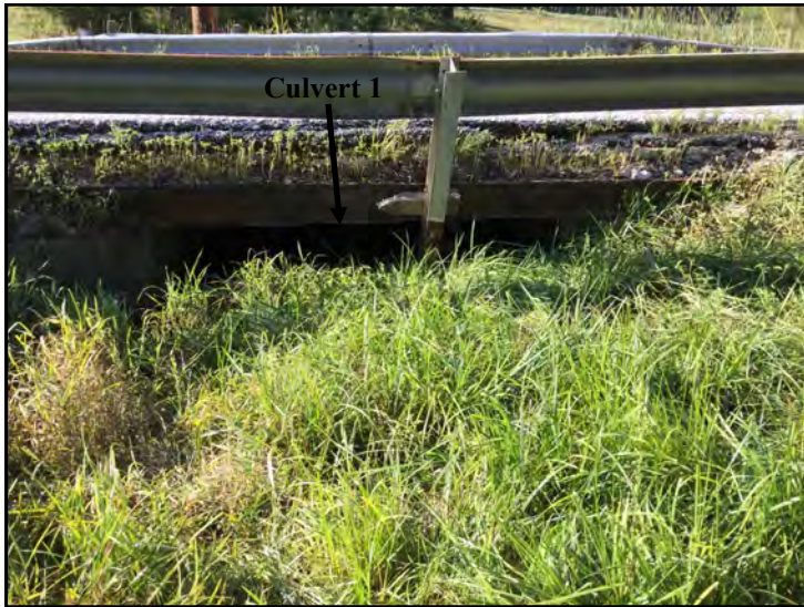
23. View of Culvert 1, looking southwest.
