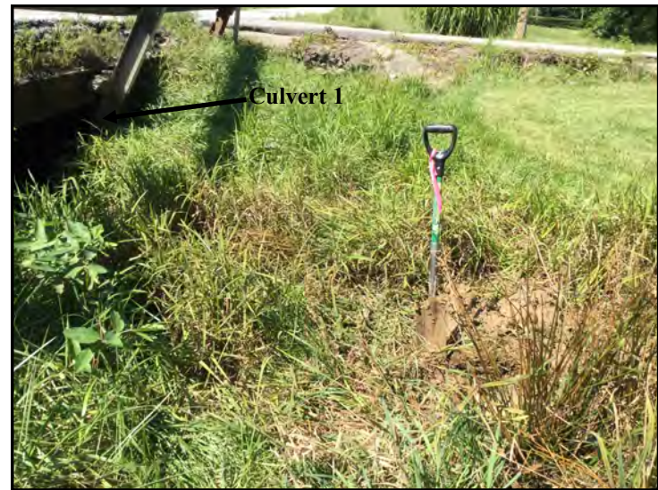
8. View of SP-B1, Wetland B, and Culvert 1, looking southwest.
