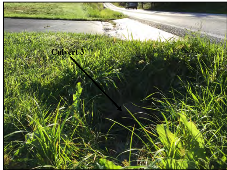
40. View of Culvert 3, looking northeast.
