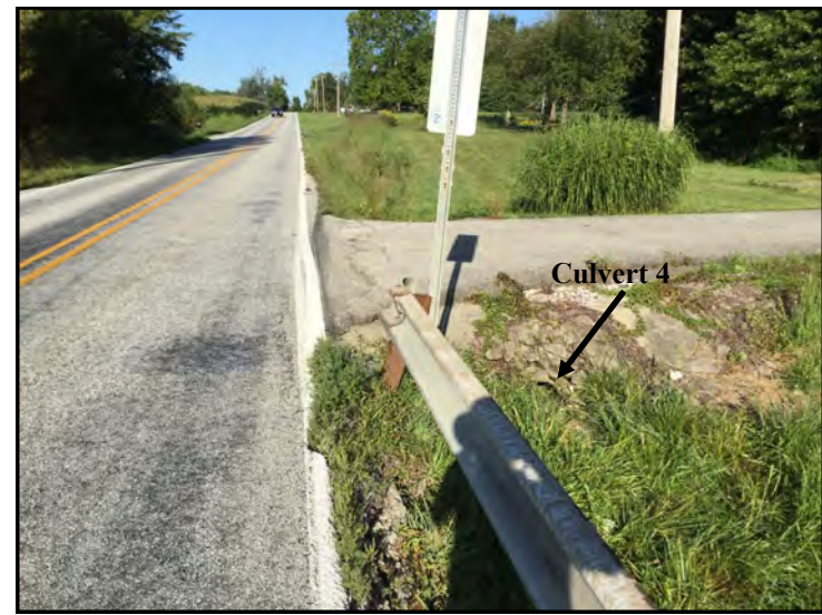
22. View of Culvert 4, looking west.
