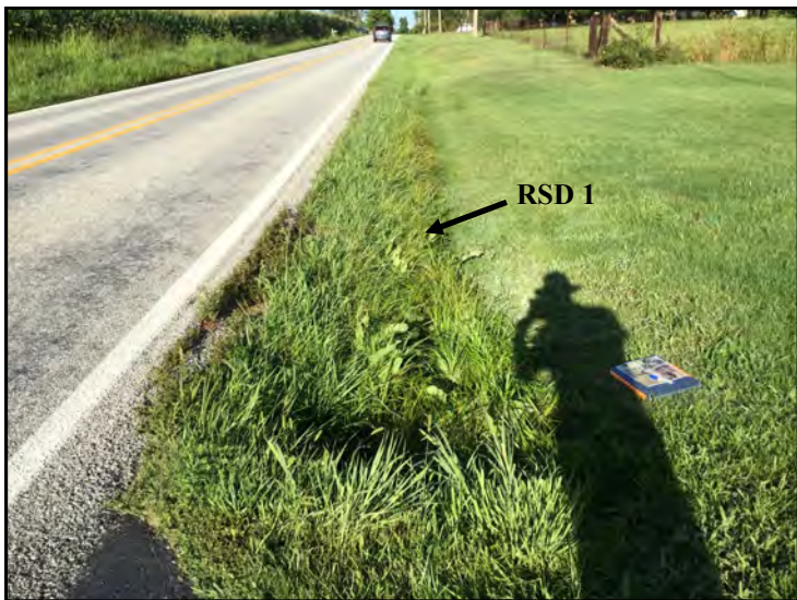
41. View of RSD 1 from Culvert 3, looking southwest.
