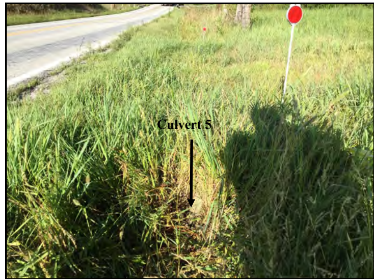
48. View of Culvert 5, looking southwest.
