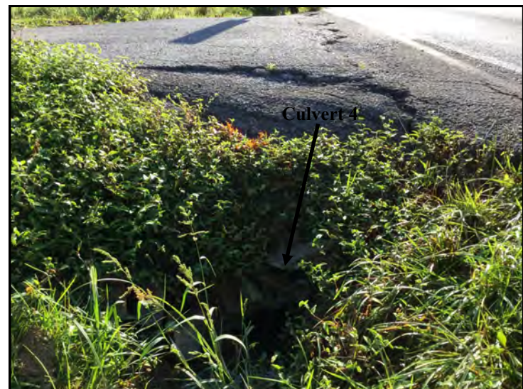
44. View of Culvert 4, looking northeast.
