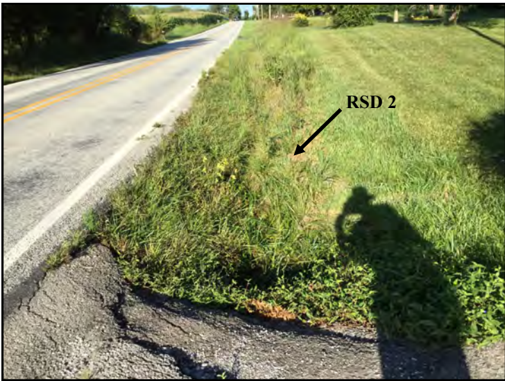
45. View of RSD 2 from Culvert 4, looking southwest.
