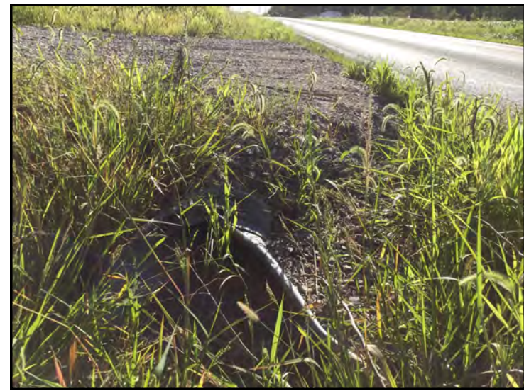
50. View of Culvert 6, looking northeast.
