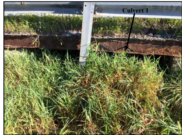
24. View of Culvert 1, looking northeast.
