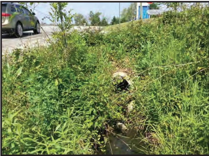
57. View of CV 6, looking northwest. (Taken 5/14/2020)
