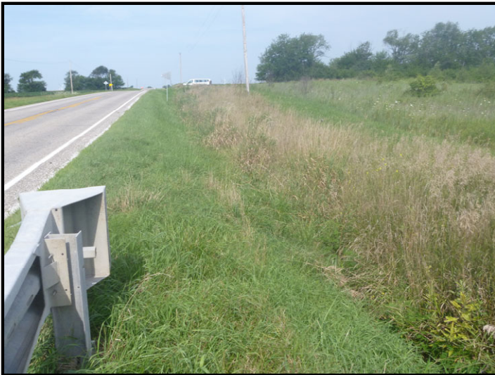
Photo 9 – Northwest Roadside Ditch: Facing west along roadside ditch in northwest quadrant of project area. Plans propose relocating ditch away from the road and extending guardrail.
