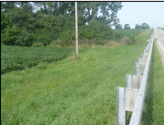
Photo 23 – Southeast Roadside Ditch: Facing southwest toward poorly defined roadside ditch in southeast quadrant of project area. Plans propose relocating ditch away from the road. Per aerials, overhead utilities were recently installed.
