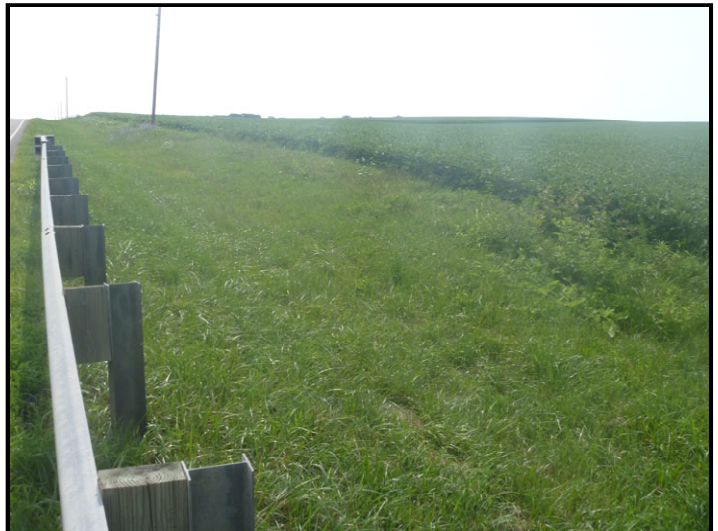
Photo 24 – Southeast Roadside Ditch: Facing southeast toward roadside ditch in southeast quadrant of project area. Proposed plans would move right-of-way and utilities into ag field.
