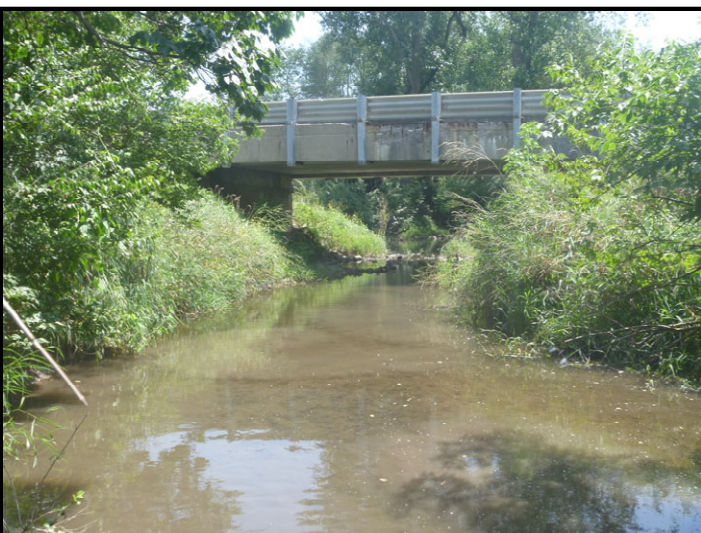
Photo 17 – Greenwood Ditch Bridge: Facing downstream to the south along Greenwood Ditch toward SR 18 bridge (from the north). OHWM measured approximately 24.5 feet wide by 20 inches deep.
