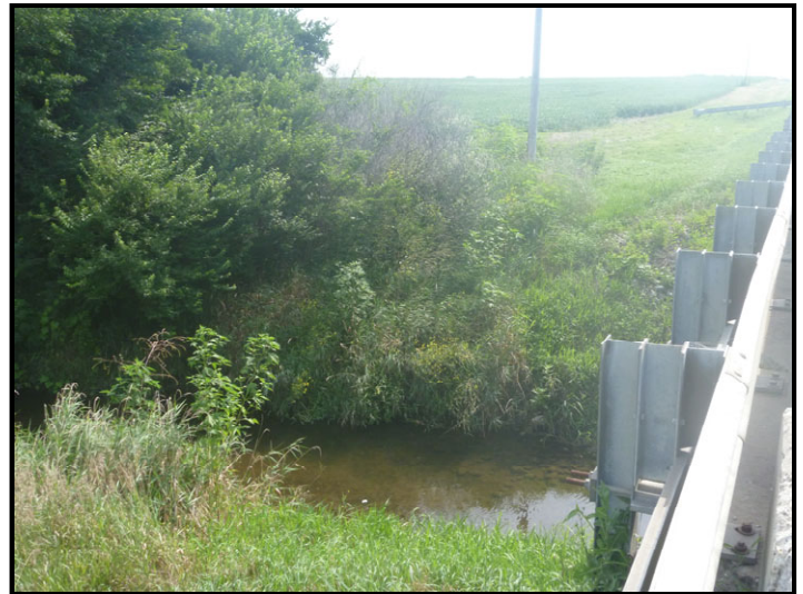
Photo 14 – Greenwood Ditch Crossing: Facing northeast quadrant of bridge and outfall of roadside ditch. Wingwalls and riprap to be installed. Vegetation surveyed in this quadrant were not indicative of wetlands.
