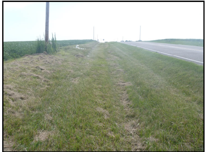
Photo 26 – Northeast Roadside Ditch: Facing east along roadside ditch in northeast quadrant of project area toward western project terminus.
