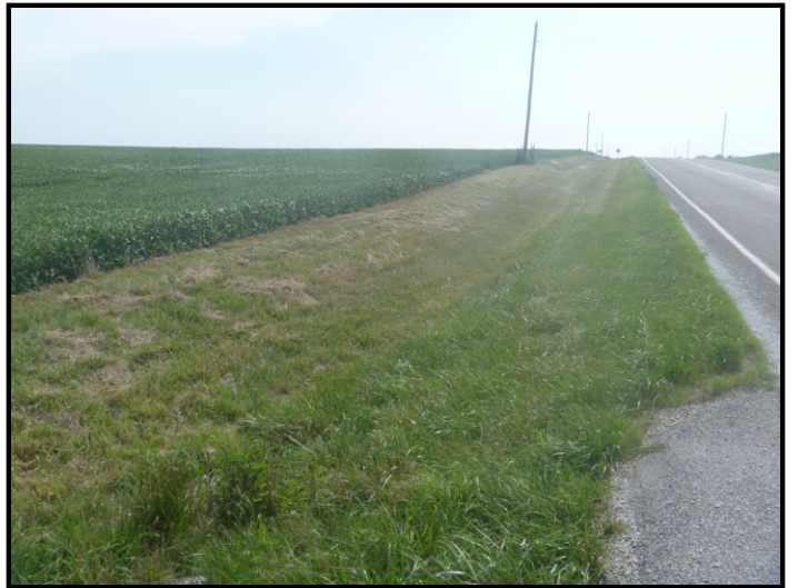
Photo 22 – Northeast Roadside Ditch: At field entrance, facing northeast along roadside ditch in northeast quadrant of project area. Proposed plans would move right-of-way and utilities into ag field.
