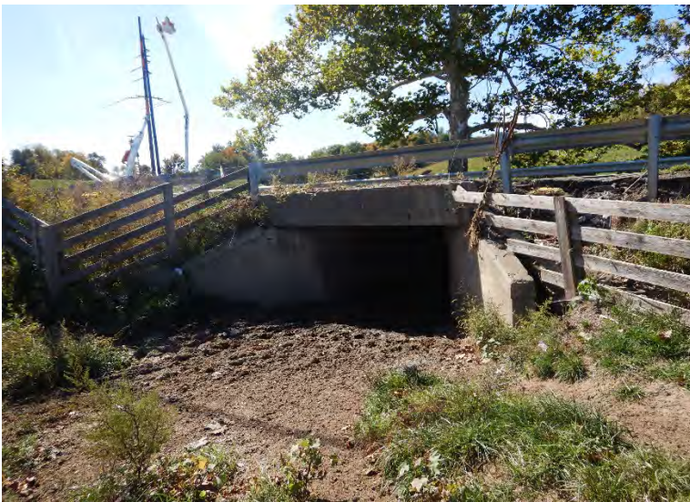
Photo 7: East Side of Structure, Outlet
