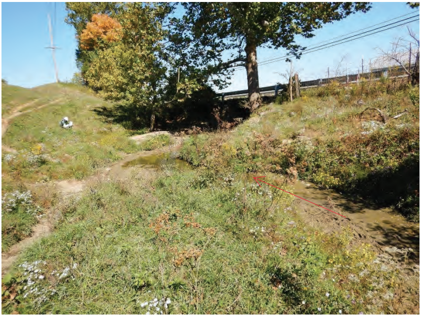
Photo 10: Buck Run, on Westside of CV 056-058-187.65, Facing North Towards Structure
