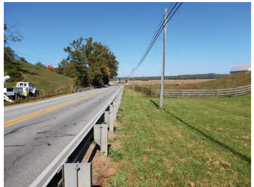
Photo 20: ROW of Eastside of SR 56, Facing North
