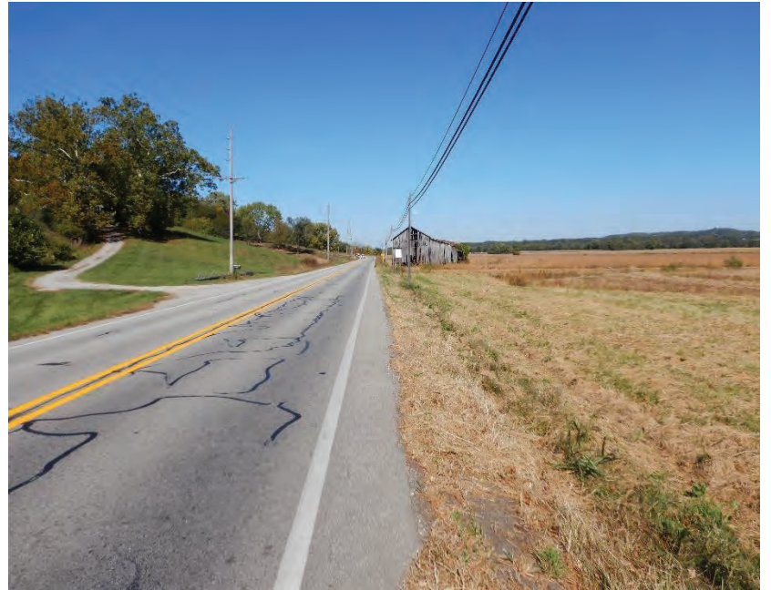
Photo 22: ROW of Eastside of SR 56, Facing North
