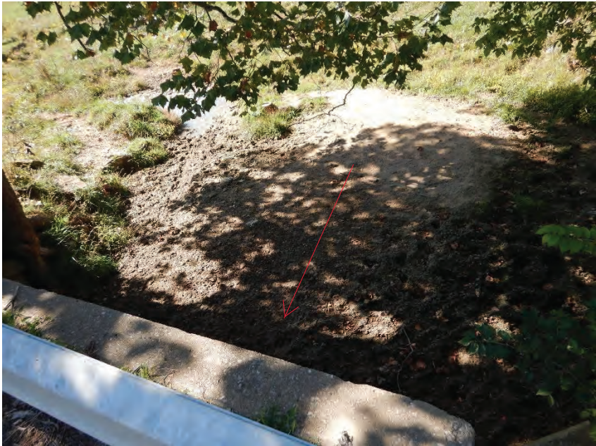
Photo 16: Facing West Towards Buck Run, on Westside of CV 056-058-187.65, From SR 56
