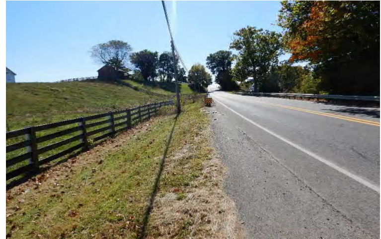
Photo 2: Northern Project Termini, SR 56 Facing South
