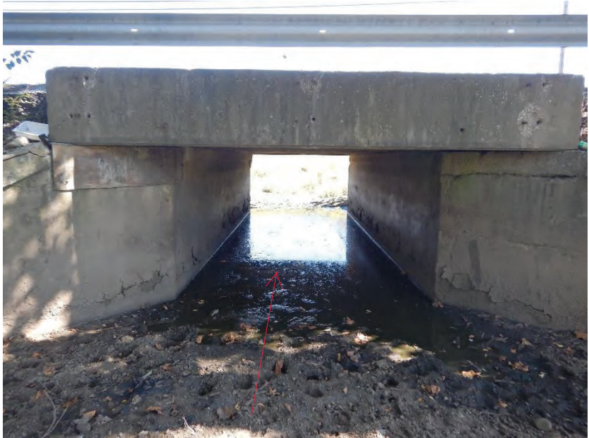
Photo 14: Buck Run, on Westside of CV 056-058-187.65, Facing East Towards Structure
