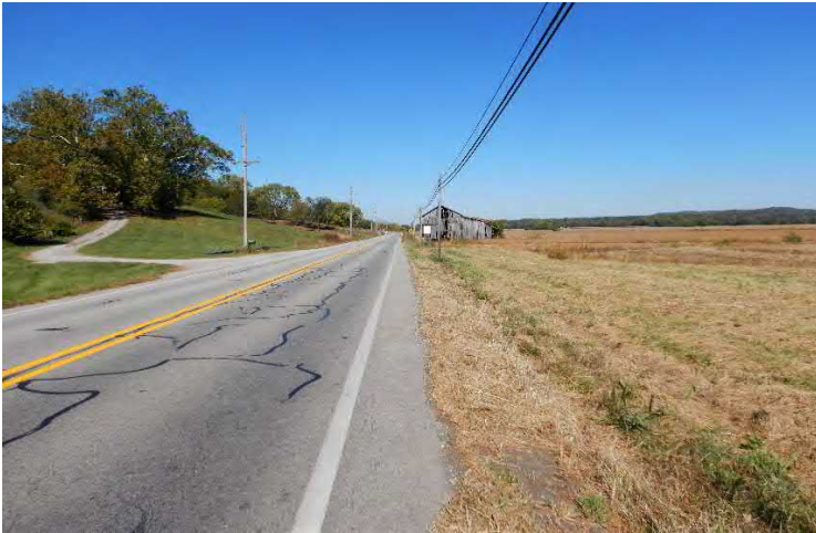
Photo 1: Northern Project Termini, SR 56 Facing North
