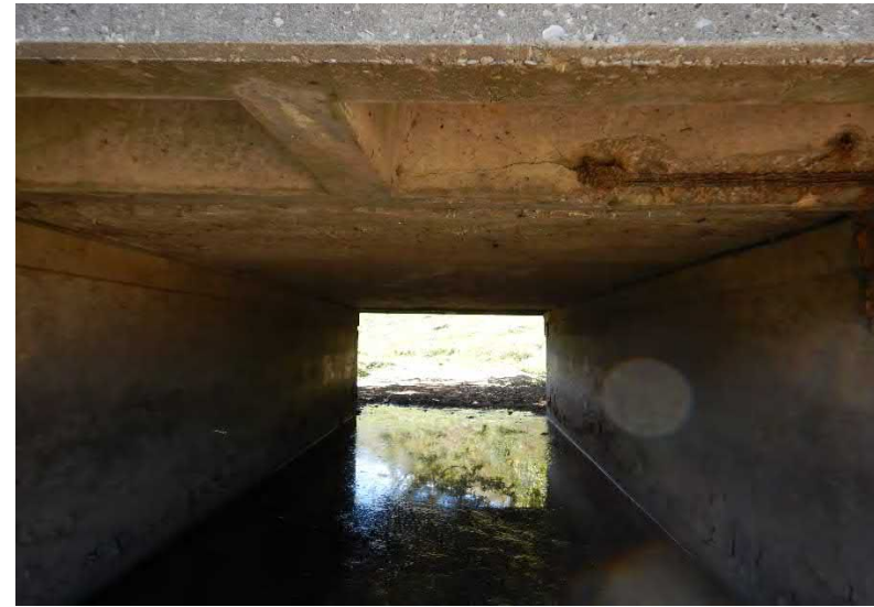
Photo 8: Inside of Structure
