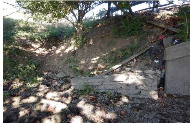
Photo 6: Rock Wall. West Side of Structure
