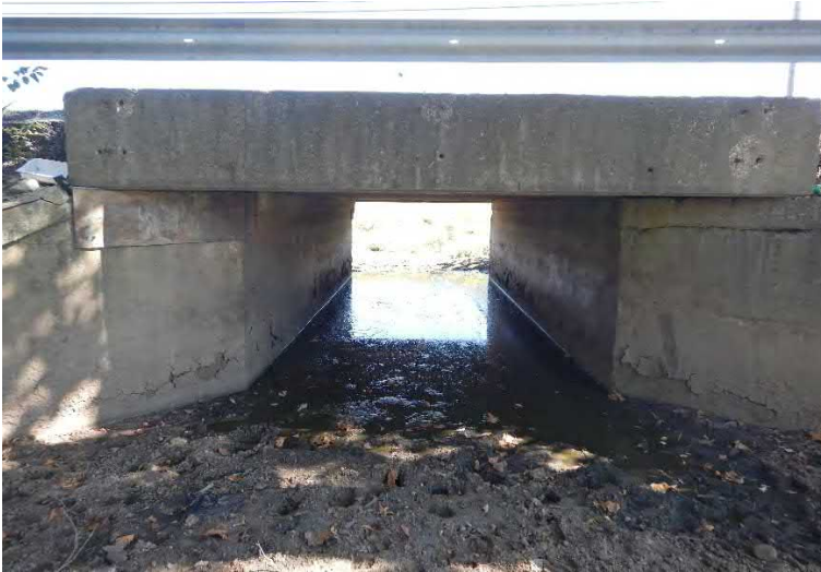
Photo 5: West Side of Structure, Inlet
