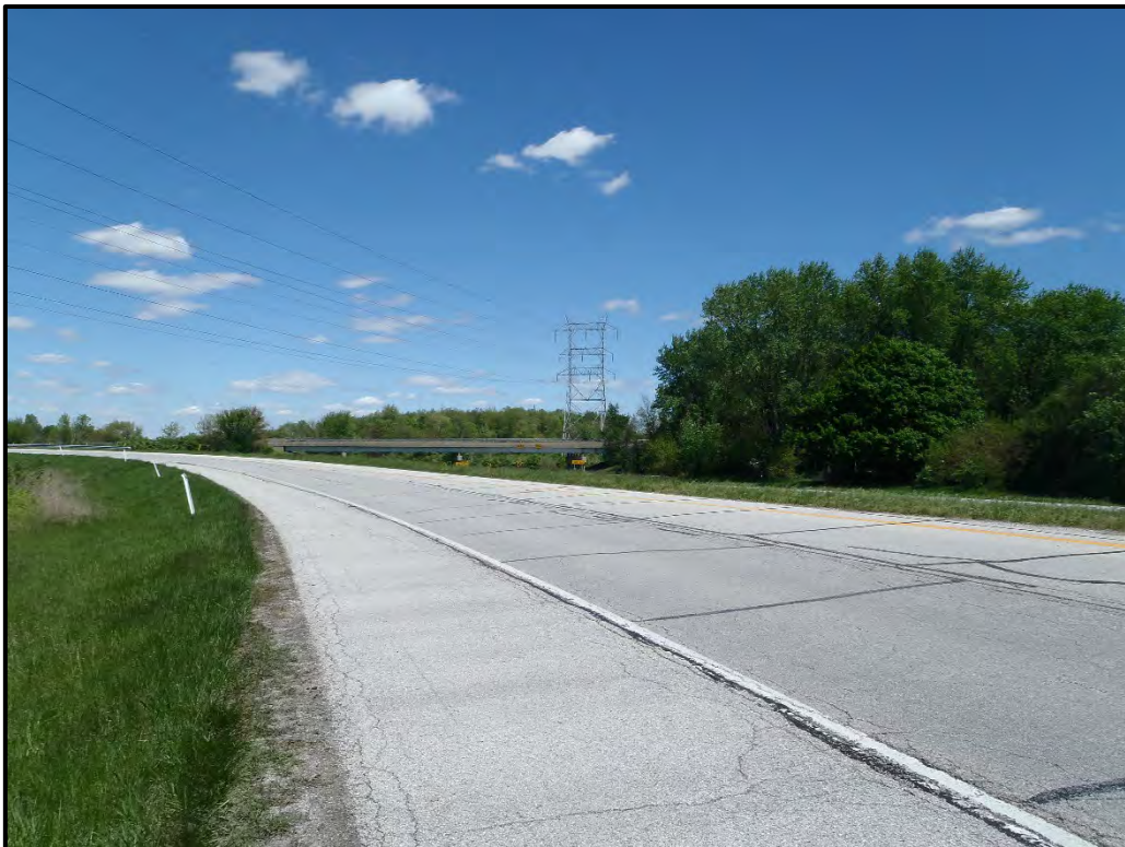
Photo 14: US 41 southbound looking toward the Old US 41 bridge (5-5-21).
