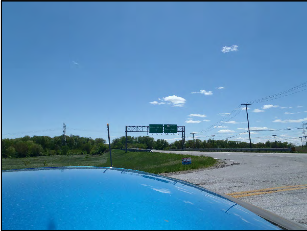
Photo 5: Looking southwest at the exit from the center intersection of Evans Ave and US 41 (5-5-21).
