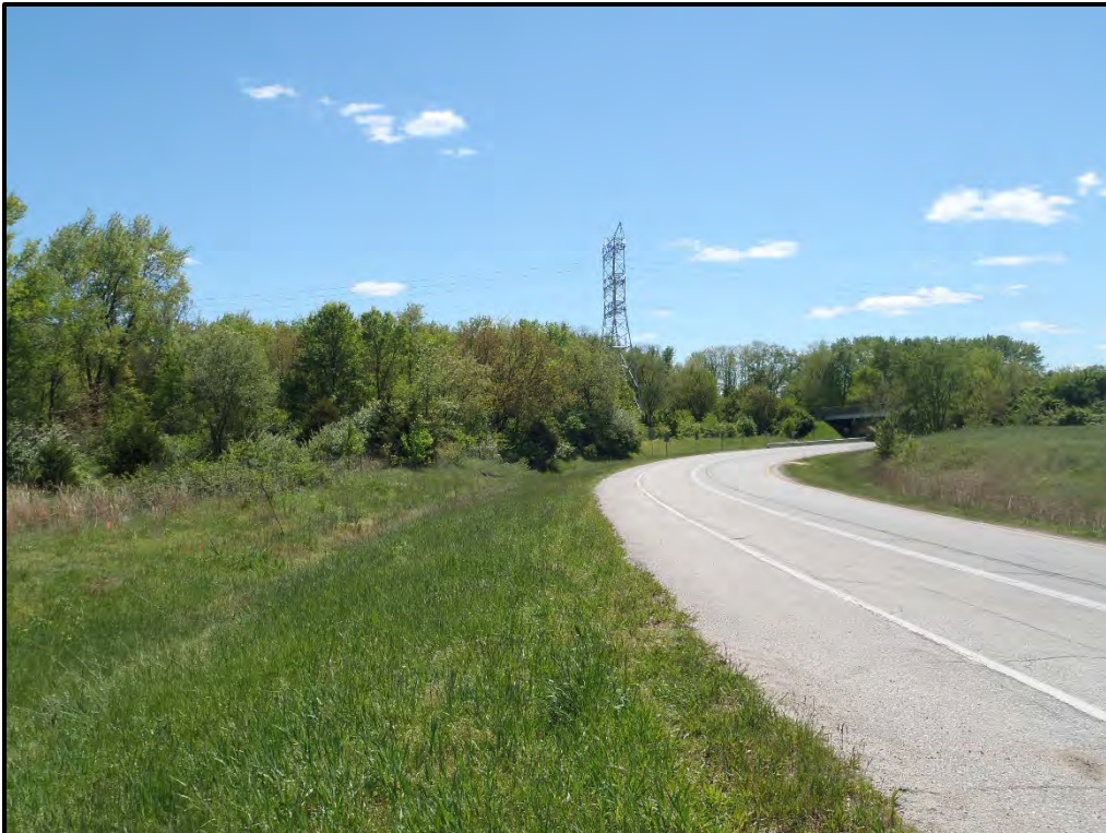
Photo 12: Looking south along north bound US 41 toward the Old US 41 bridge (5-5-21).
