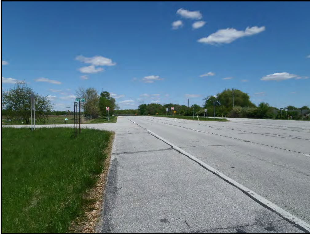
Photo 15: Looking north from the Quinn Rd and US 41 intersection (5-5-21).
