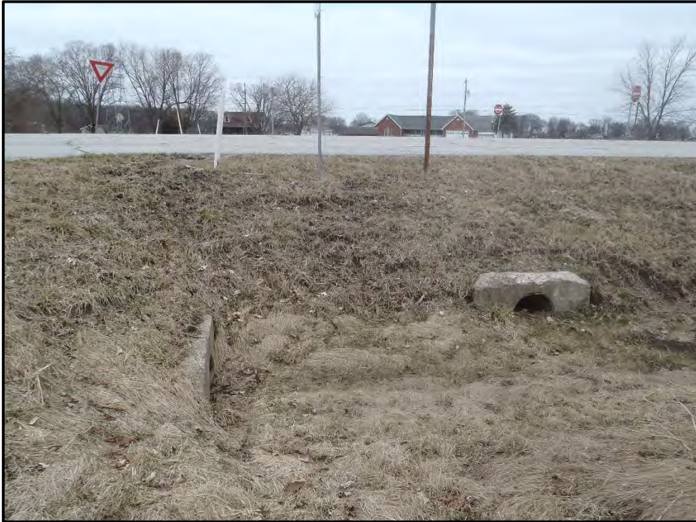
Photo 25: Overflow structures on the northside of Budd Street and US 41 NBL. (3-8-22)
