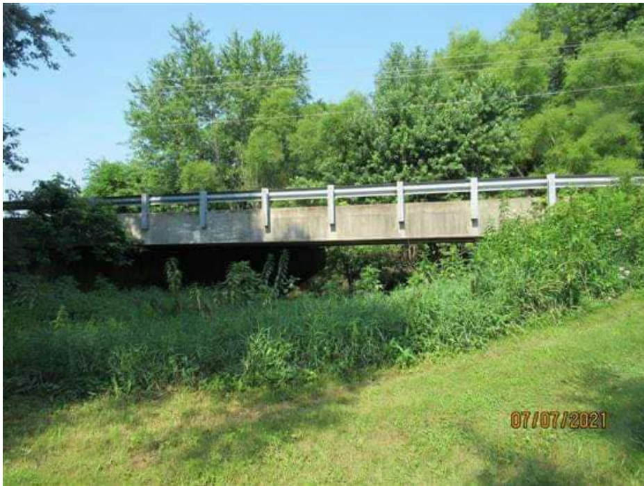
PHOTO 2 Description East Elevation
