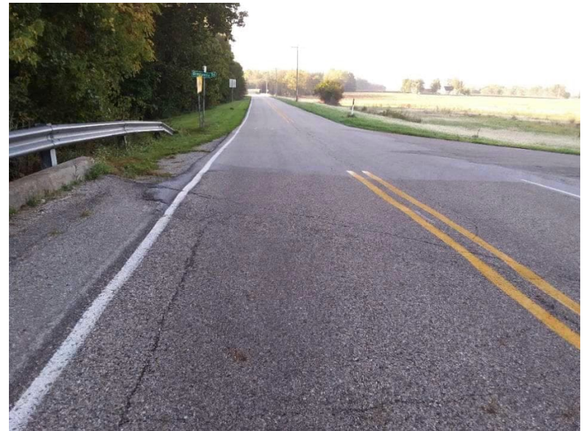
PP-2; Looking south at Johnson County Bridge 98 at the E. Urmeyville Rd and CR 700 E intersection
