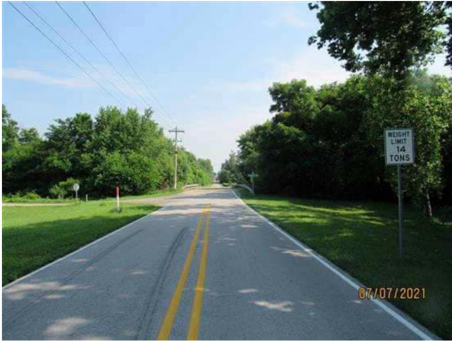
PHOTO 1 Description Alignment Looking North (14 Tons)
