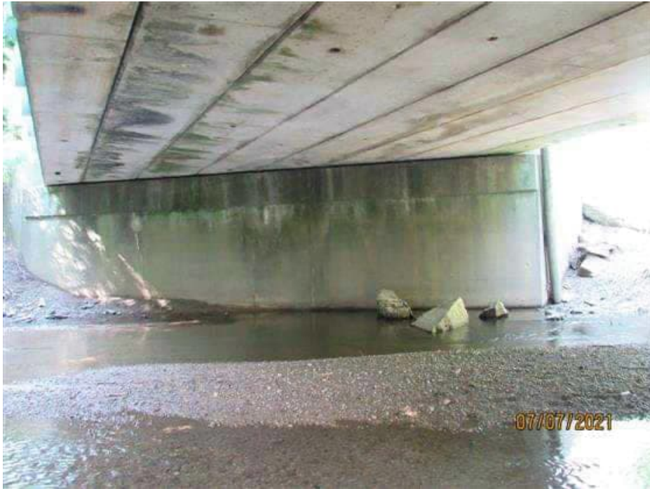
PHOTO 13 Description Bent 1 and Span A Superstructure
