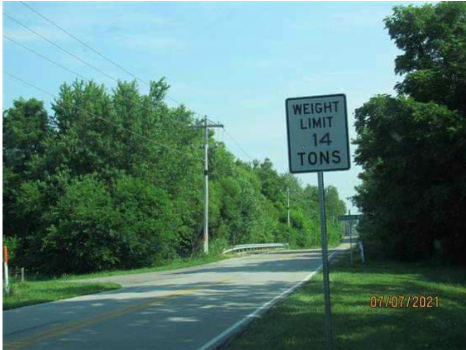
PHOTO 5 Description Alignment Looking North (14 Tons)
