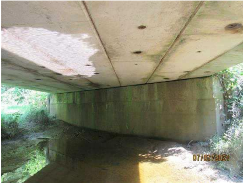
PHOTO 11 Description Bent 3 and Span B Superstructure
