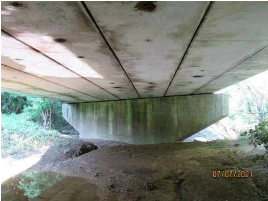
PHOTO 12 Description Pier 2 and Span B Superstructure
