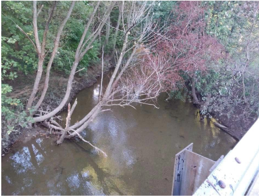
PP-2; Looking west, upstream, from Johnson County Bridge 98 from Little Sugar Creek (2021-10-20)
