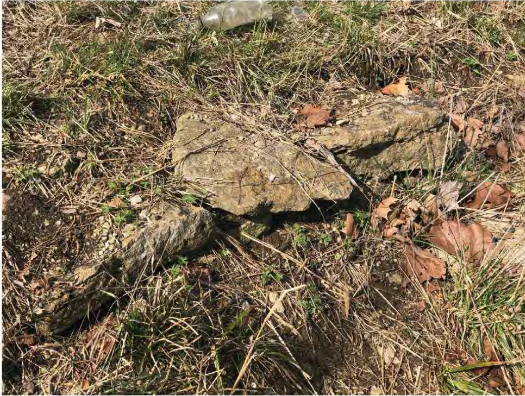
Top of retaining wall:
