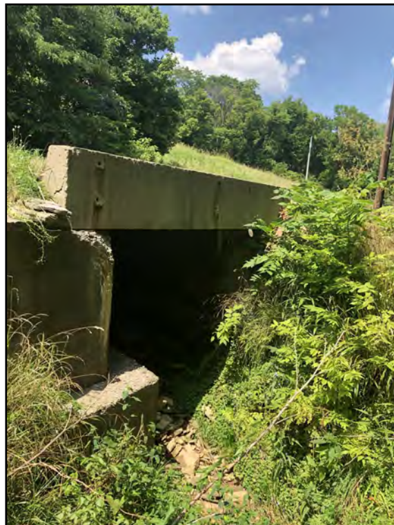
Photo 8: Southeast side of the culvert.
