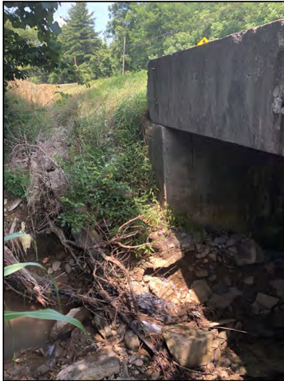
Photo 5: Northwest side of culvert.
