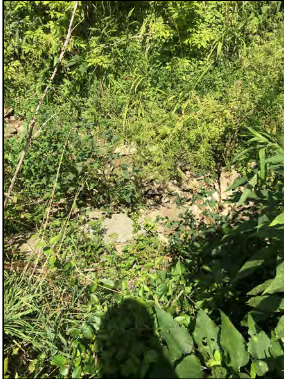
Photo 9: Bank on the southeast side of the culvert. Channel is saturated but no surface water is present.
