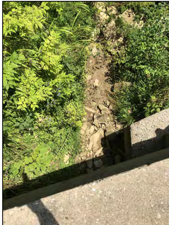
Photo 10: View of the bank of the southeast side of the culvert. Channel is saturated but no surface water is present.
