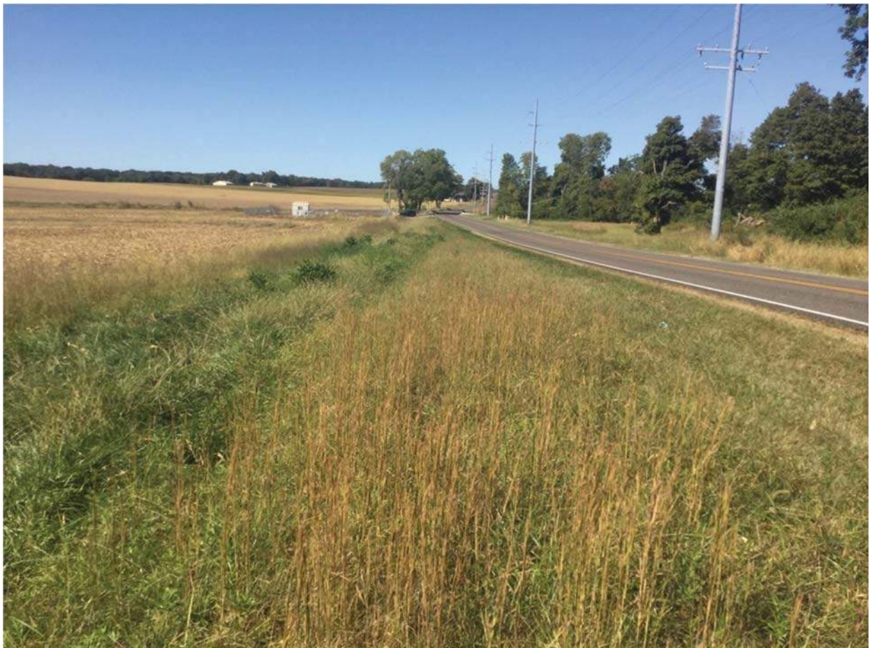
34. View of investigated area and SR 65 looking north
