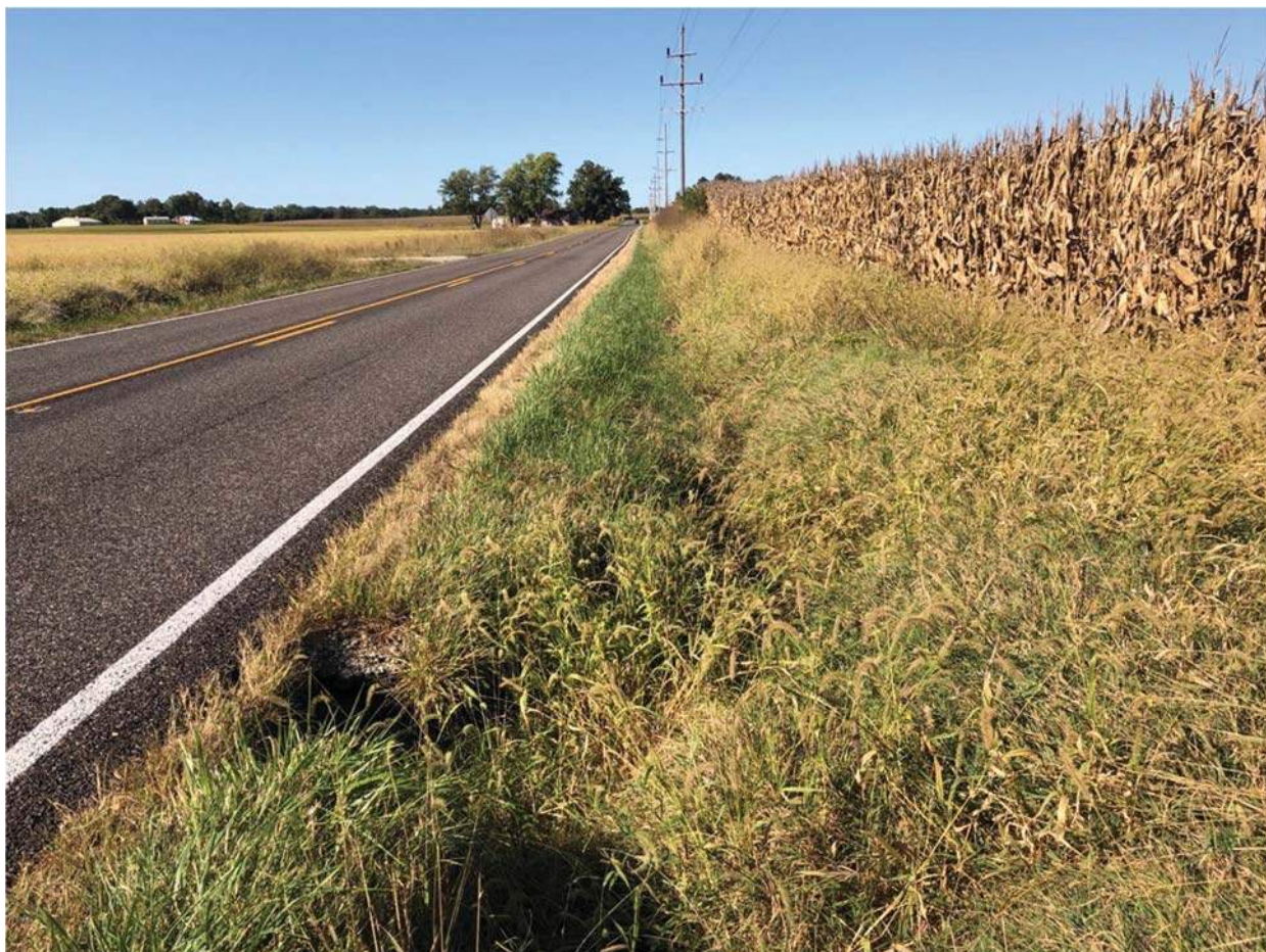
20. View of investigated area and SR 65 looking north
