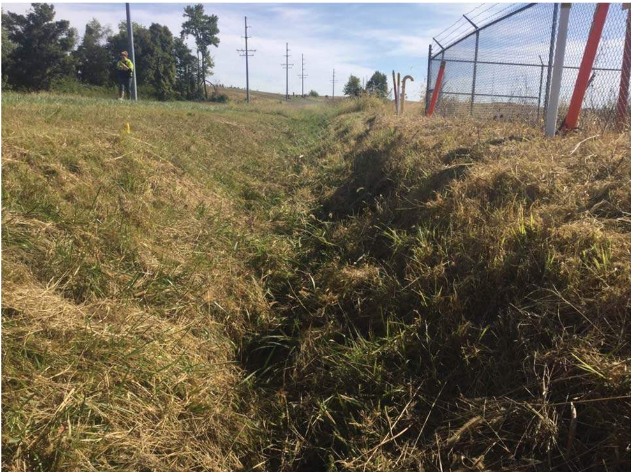
18. View of RSD 1 and investigated area looking south
