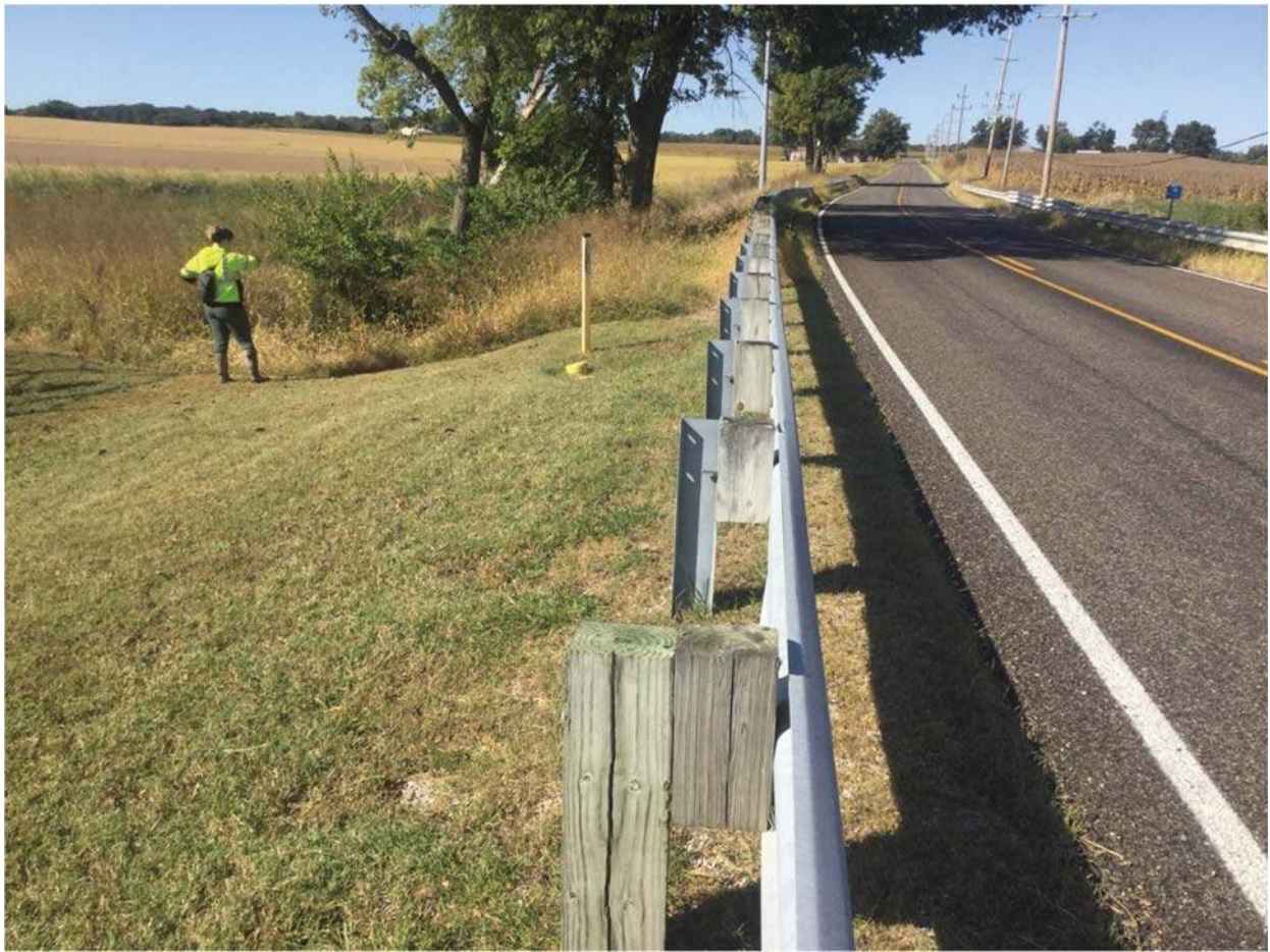
37. View of investigated area and SR 65 looking north
