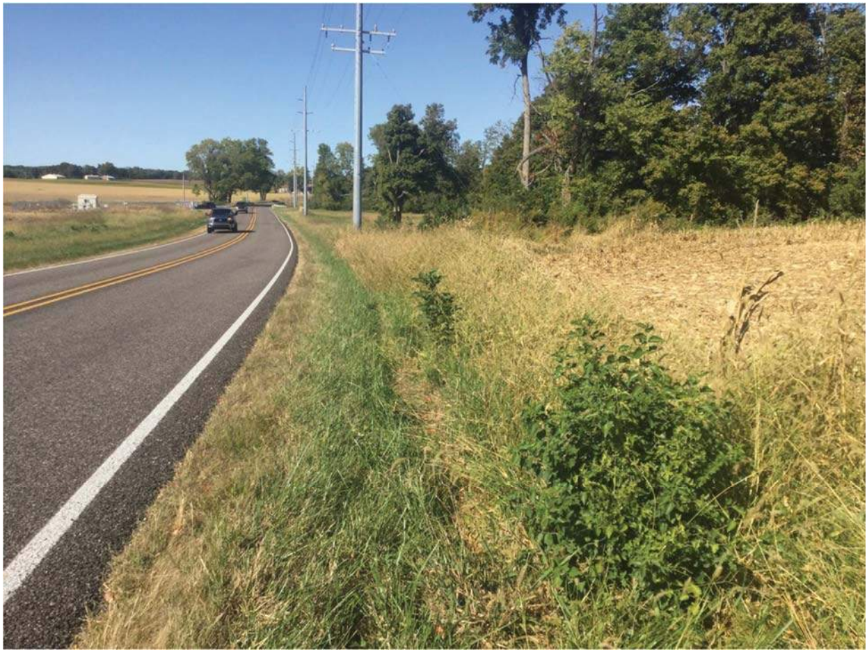
31. View of investigated area and SR 65 looking north
