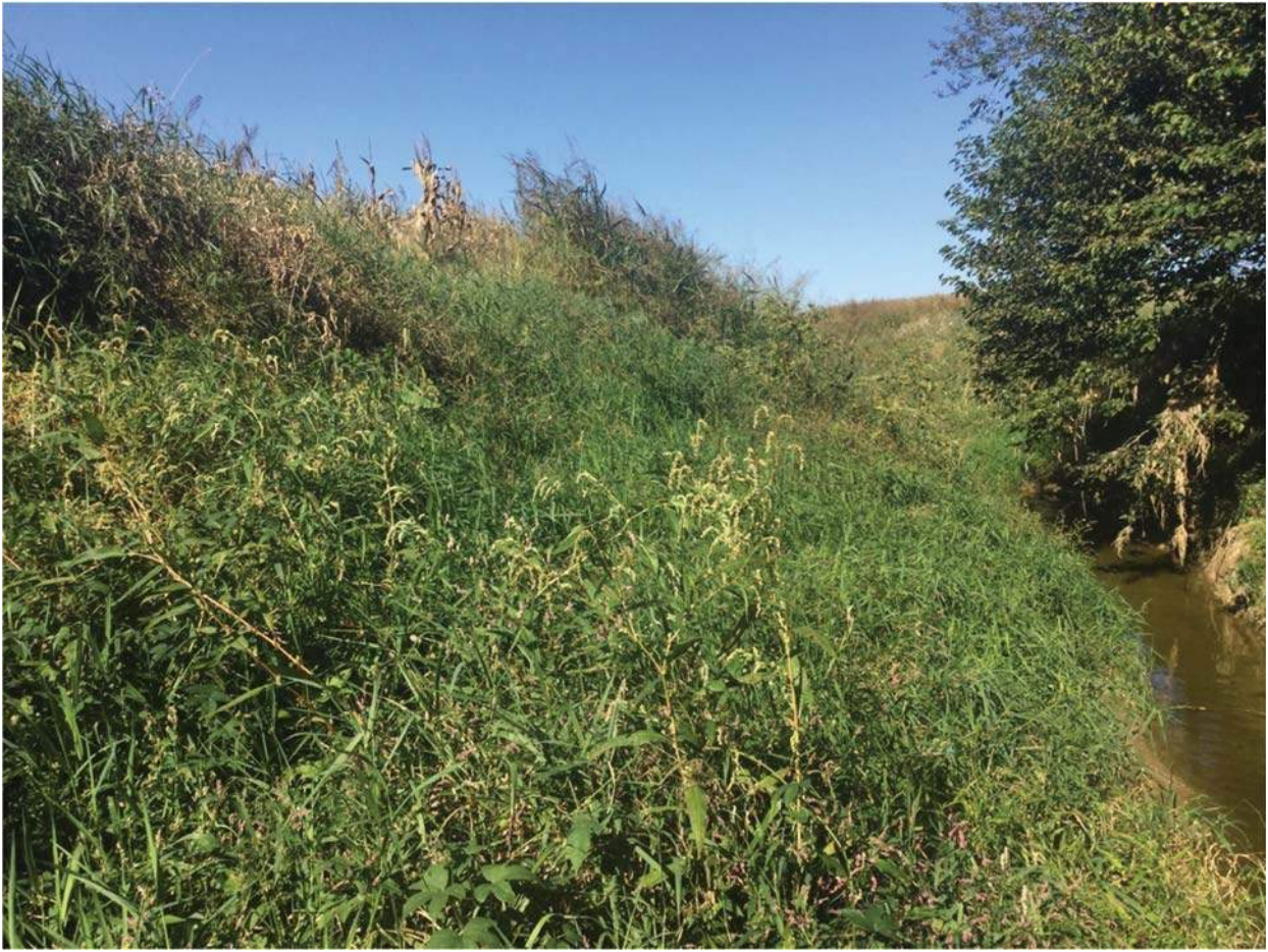
25. View of investigated area and Black River looking east
