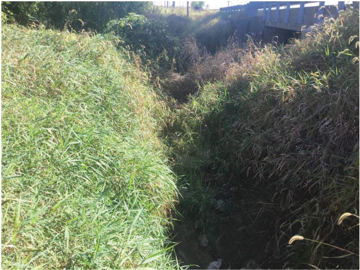
23. View of investigated area and SR 65 bridge looking south
