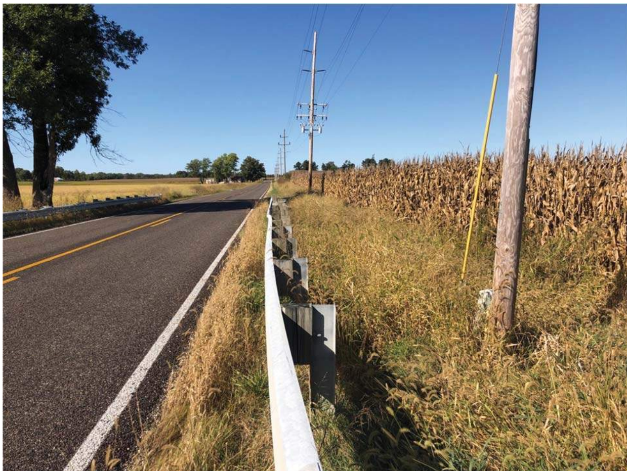
22. View of investigated area and SR 65 looking north
