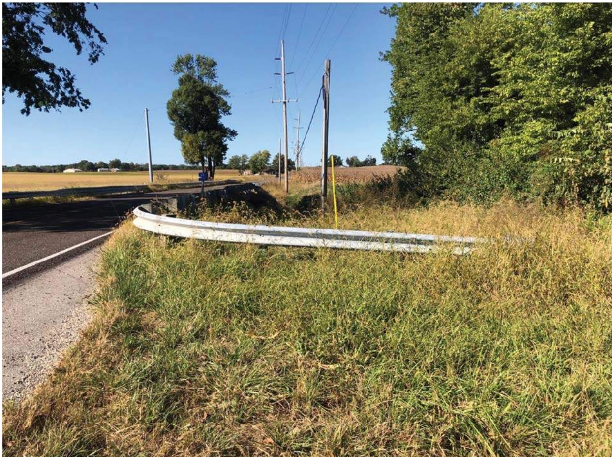
38. View of investigated area and SR 65 looking north
