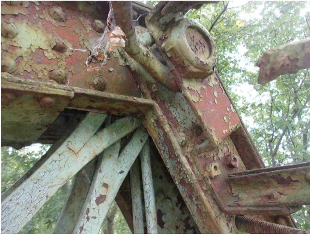
Photo 37: Typical Outside Condition on Upper Chord
