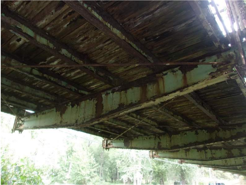
Photo 35: Typical Floorbeam Condition
