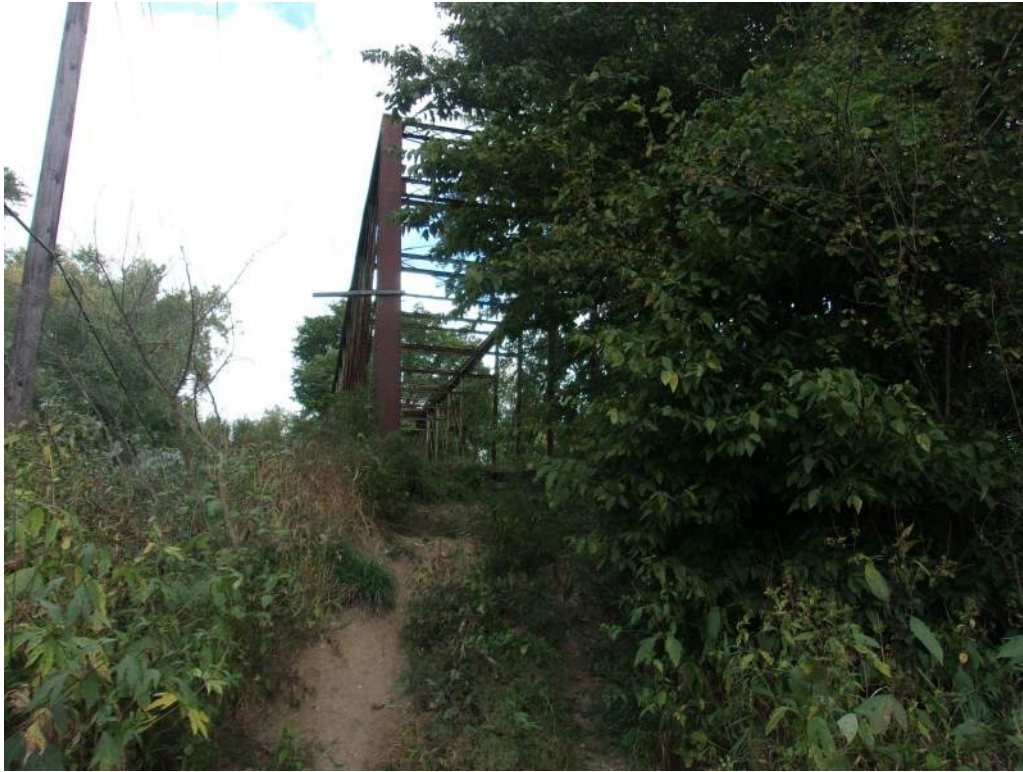
Photo 33: Typical Approach Looking East
