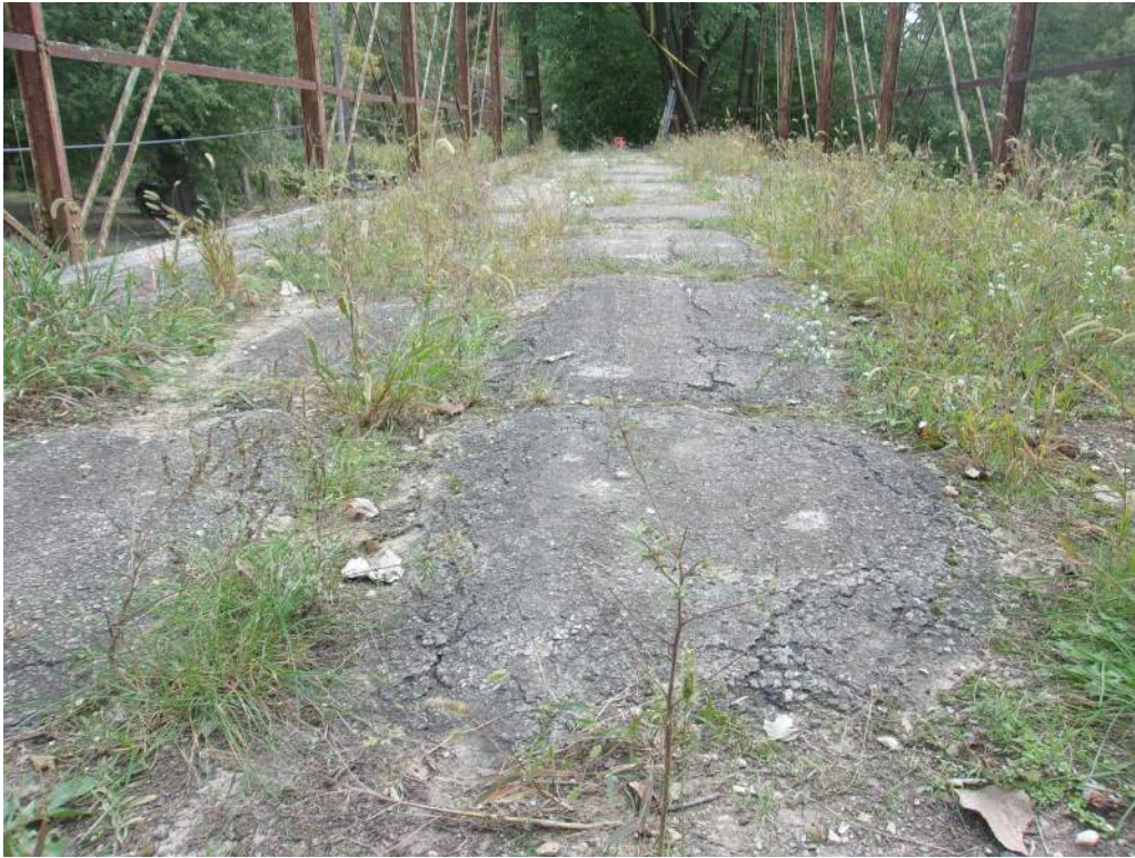
Photo 7: Typical Asphalt Wearing Surface
