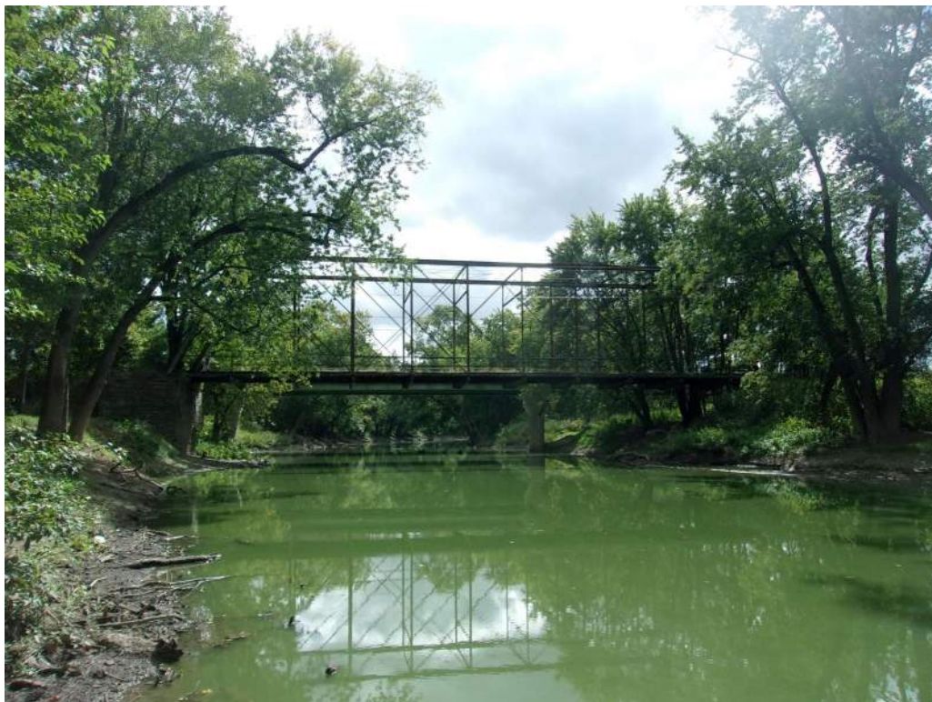
Photo 30: Bridge Elevation Looking South
