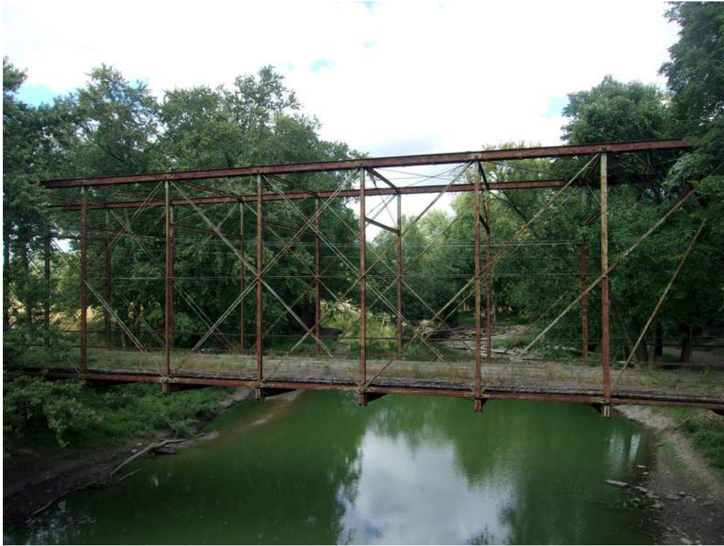
Photo 31: Bridge Elevation Looking North
