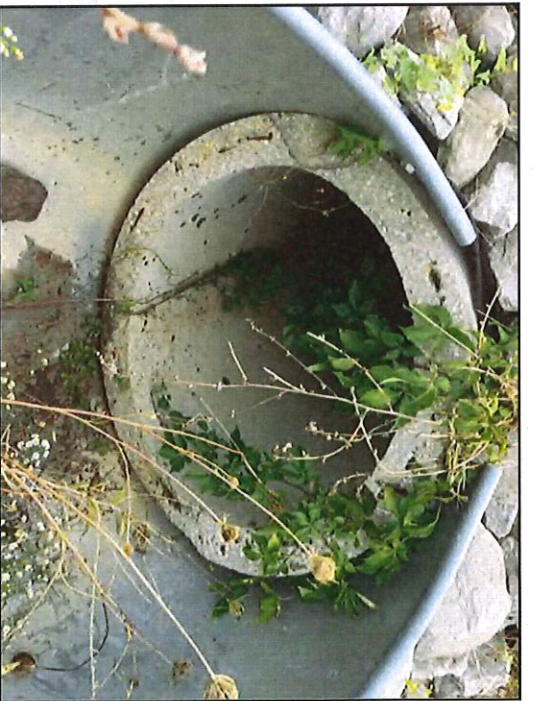
34. View of culvert, approximately 24 inches in diameter, looking east.
