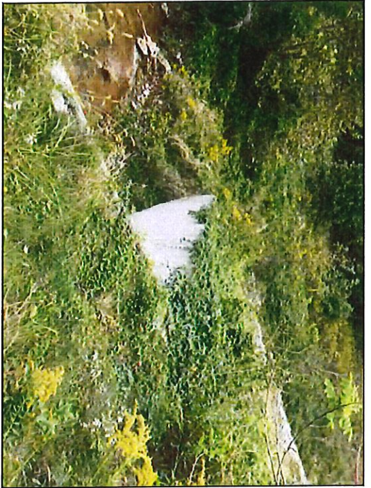
61. View of southeastern bank of UNT 1 and RSD 7, looking northeast.
