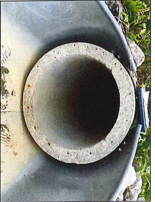
37. View of culvert, approximately 30 inches in diameter, looking east.
