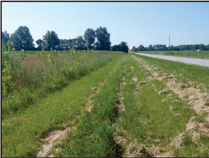
Photo 25 – Southeast Quadrant: Facing south along the east side of SR 159 along the vegetated right-of-way beyond the southern terminus of RSD-1.
