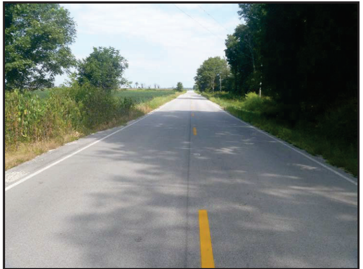
Photo 10 – SR 159 Crossing of UNT to Splunge Creek: Facing north along SR 159 from the top of the small structure at Splunge Creek. Topography is flat and land use is forested, agricultural, and rural residential.
