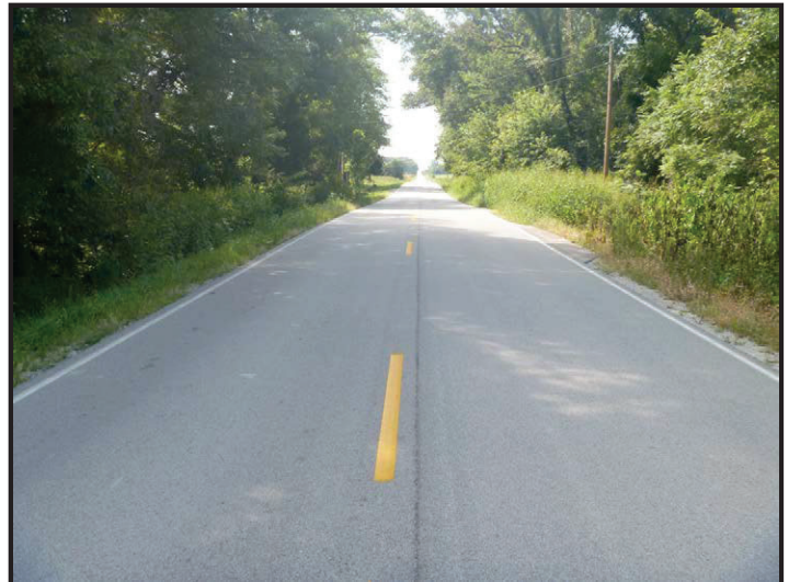
Photo 58 – Project Setting at Culvert: Facing south along SR 159 from immediately north of the subject small structure and toward the primary part of the project area.
