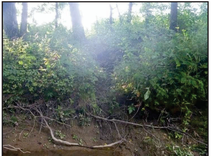
Photo 6 – Erosional Feature at UNT to Splunge Creek: Facing northwest toward the outfall of an erosional feature (EF-1) that carries field drainage into UNT to Splunge Creek.
