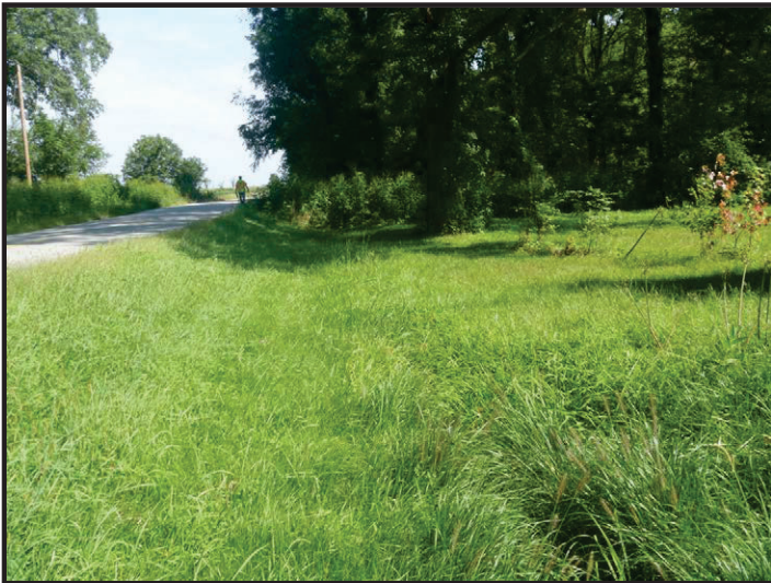
Photo 31 – Southeast Quadrant, RSD-1: Facing downgrade to the north along RSD-1. The ditch becomes poorly defined along the remaining segment toward its outfall into UNT to Splunge Creek.
