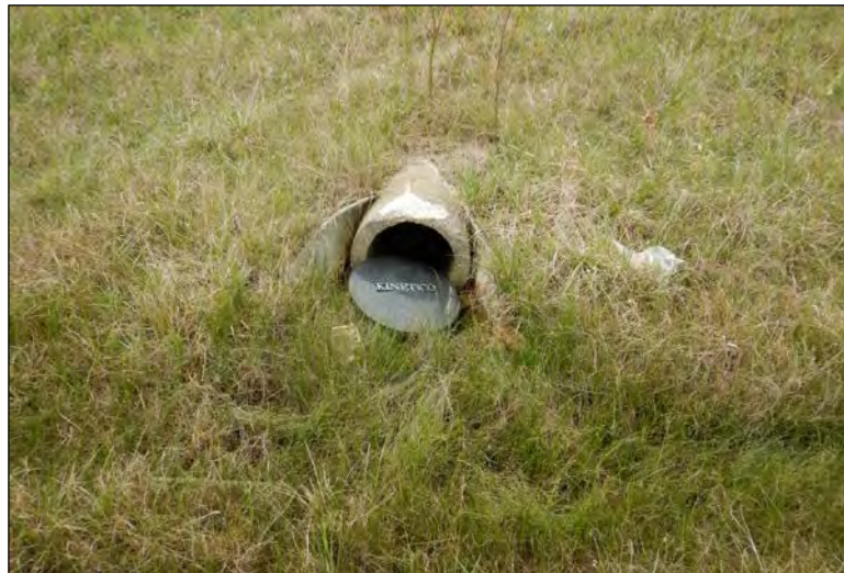
Photo 55: Culvert opening to Wetland 6.
