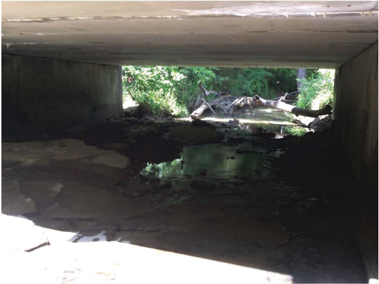
5. View of Slate Creek and investigated area looking north
