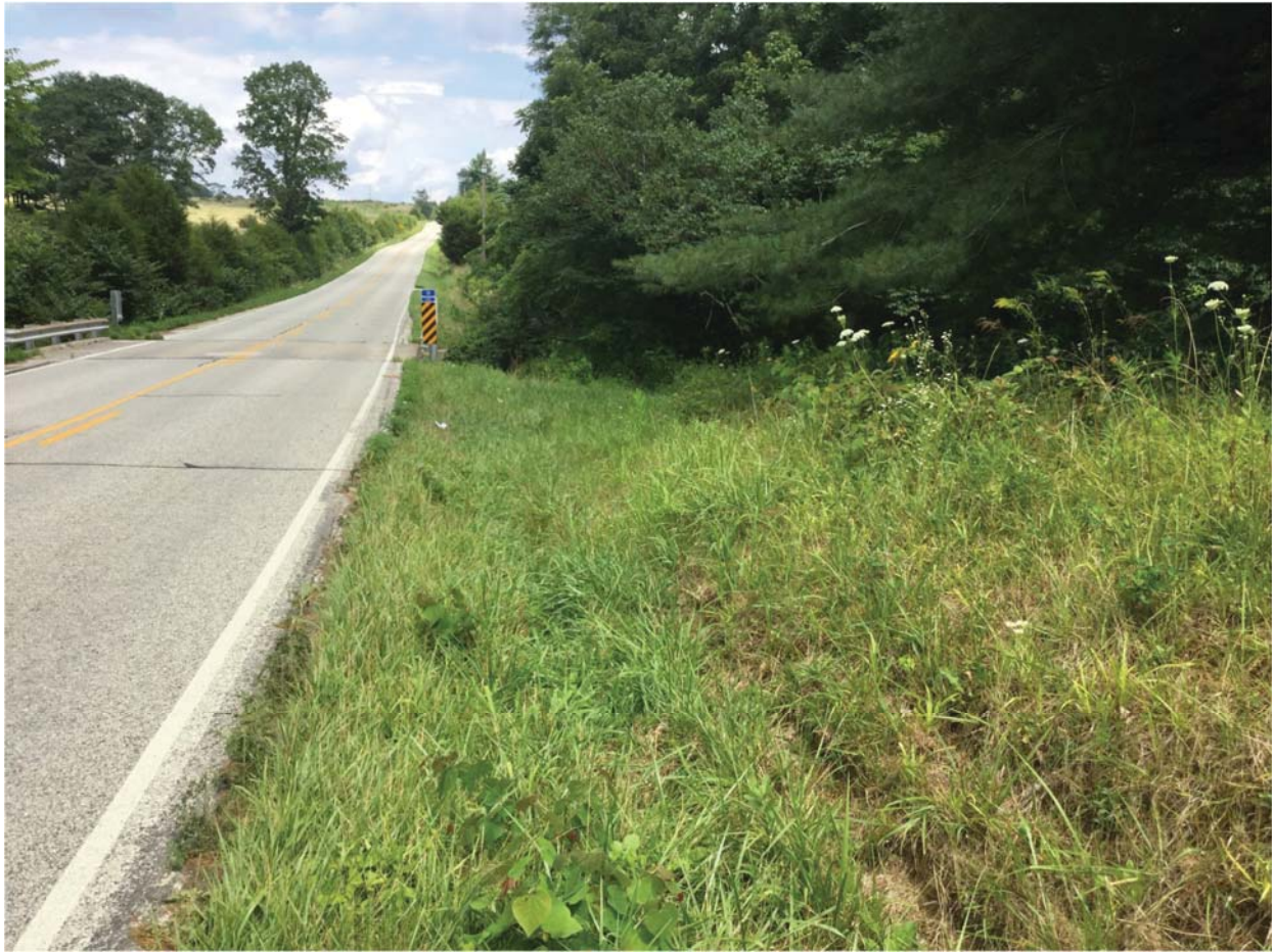
23. View of investigated area and SR 250 looking southeast
