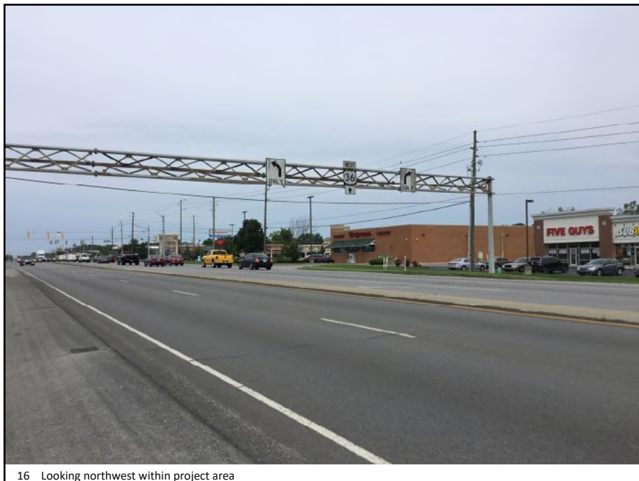
16 Looking northwest within project area
