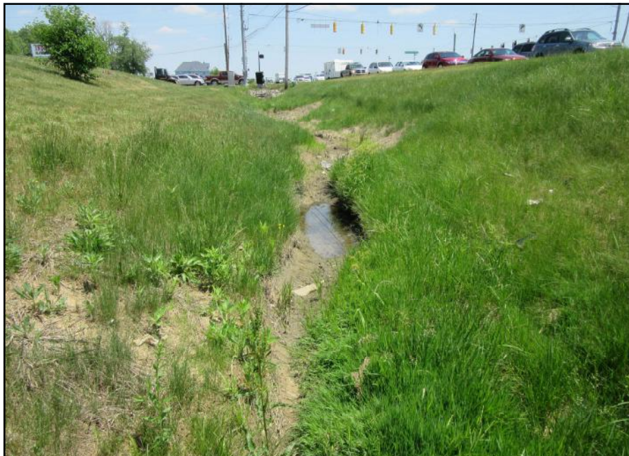
9 Looking east at UNT 1 to Avon Creek
