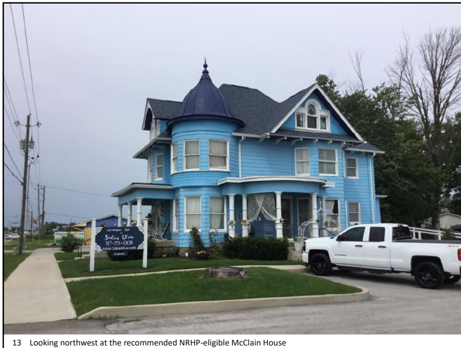
13 Looking northwest at the recommended NRHP-eligible McClain House
