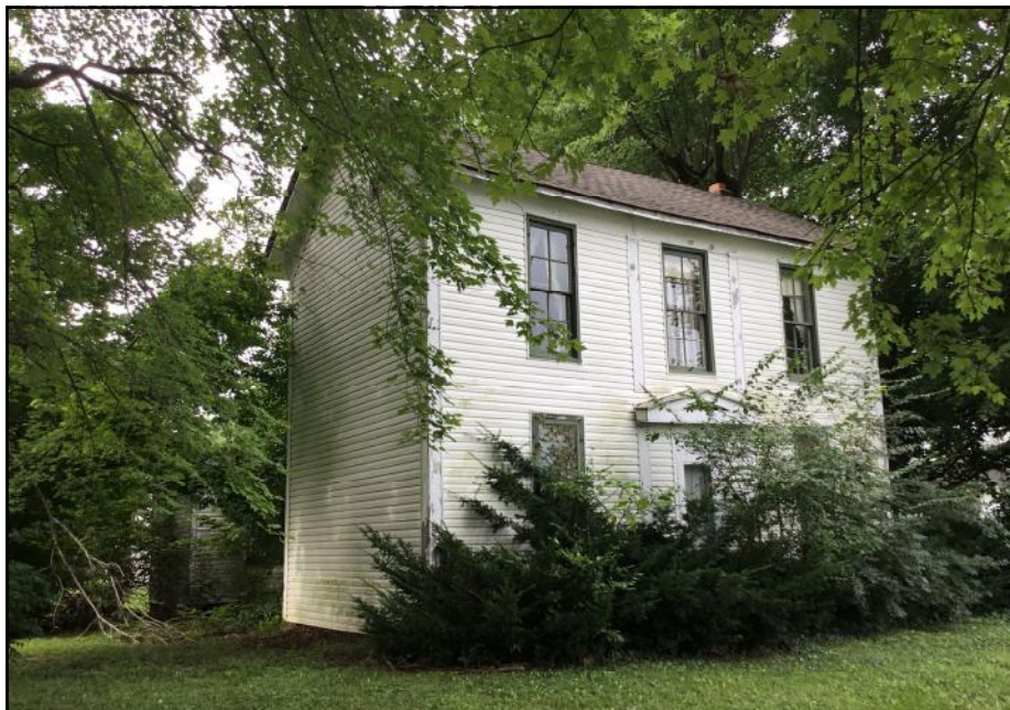
18 Looking southwest at the recommended NRHP-eligible David Faucett House
