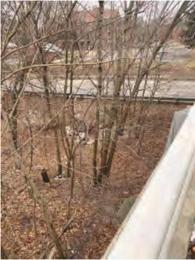
Photo 21. Facing west to south side of bridge to be removed.
