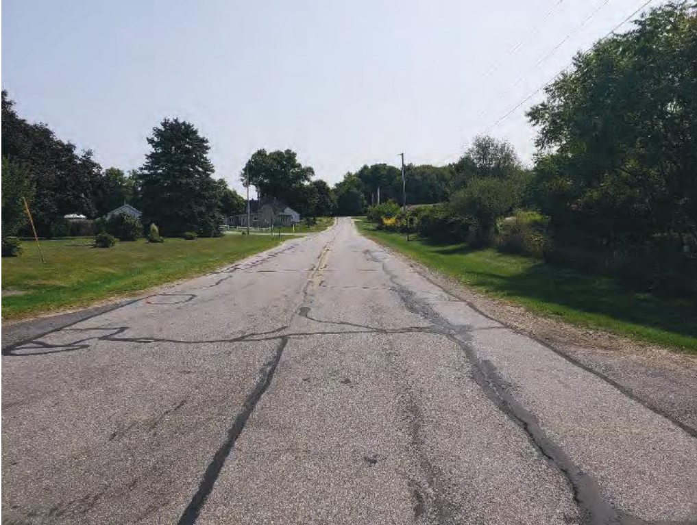
1. Facing east on Northport Rd. at 300E
