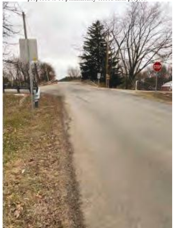
Photo 16. Facing east to intersection of Northport Rd and Northport Rd (Kelly St) and bridge to be removed over SR 9.
