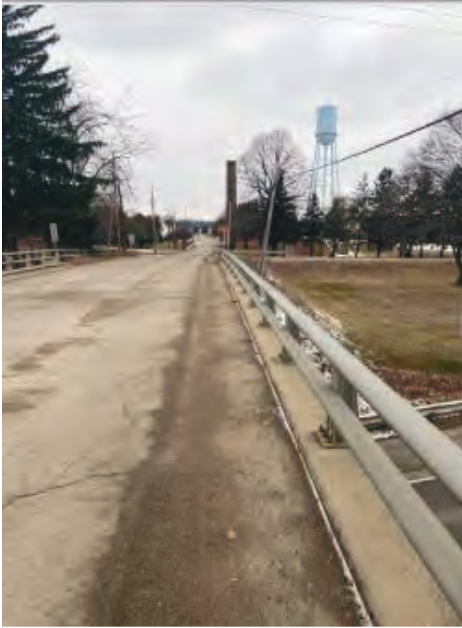
Photo 17. Facing west on bridge to be removed over SR 9.
