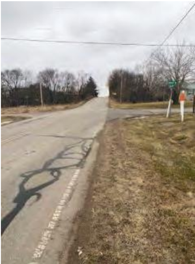
Photo 18. Facing west from eastern project endpoint at the intersection of Northport Rd and CR 300 E to bridge over SR 9 to be removed.
