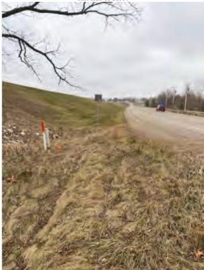
Photo 10. Facing south from east side of SR 9 from southern project endpoint.
