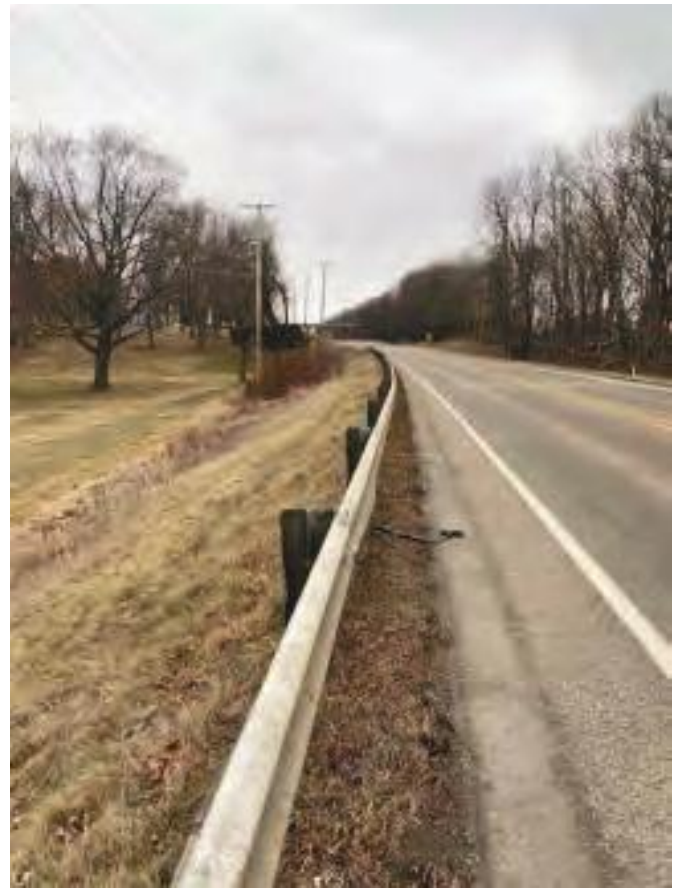
Photo 11. Facing north from west side of SR 9, near southern project endpoint.
