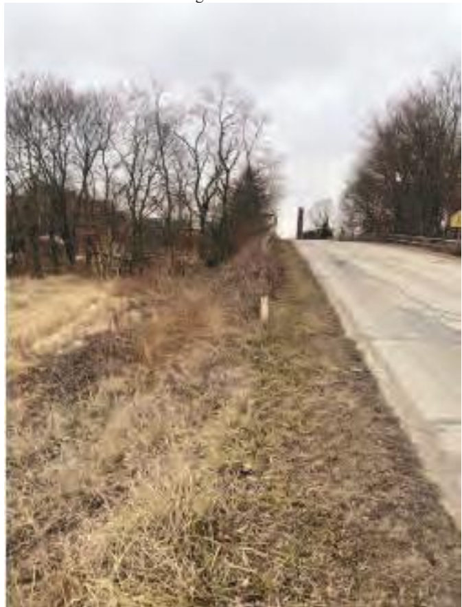
Photo 20. Facing west along south side of Northport Rd to bridge to be removed.
