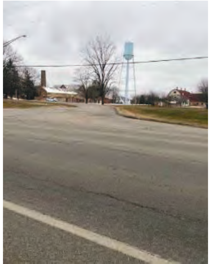
Photo 3. Facing southwest to Northport Rd intersection; this roadway and approach proposed for removal.
