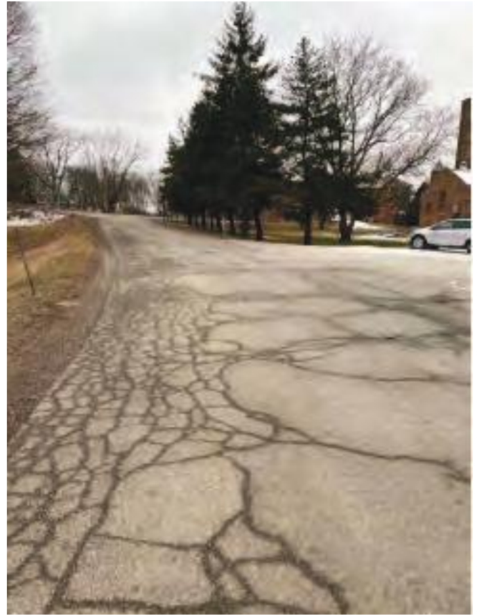
Photo 15. Facing southwest along section of Northport Rd (Kelly St) proposed to be permanently closed after project.
