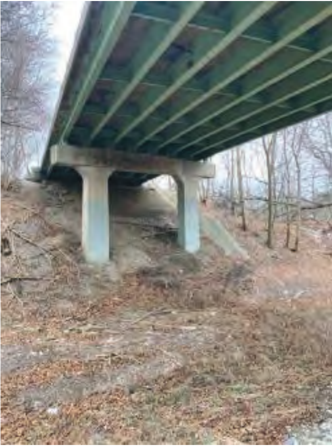
Photo 5. Eastern bridge pier, facing southeast.
