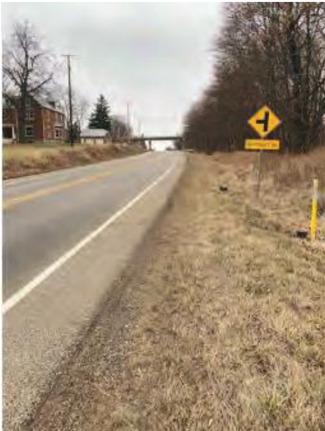
Photo 9. Facing north to bridge proposed for removal, east side of SR 9.
