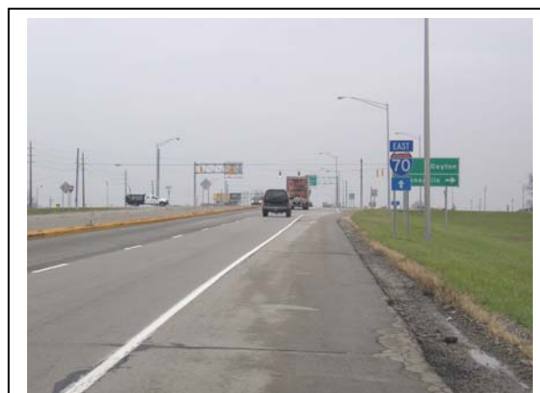
SR 9 is widened to four lanes as it approaches the I-70 interchange.
