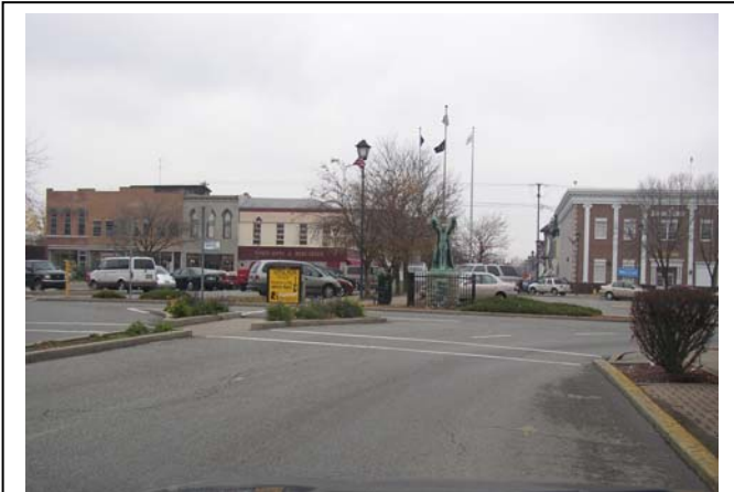
SR 9 is four lanes from I-74 to downtown Shelbyville, but capacity is limited through the downtown area.
