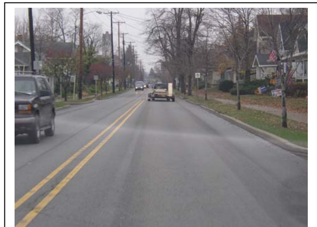
SR 9 is a two-lane street with curb and gutter where it passes through Greenfield.
