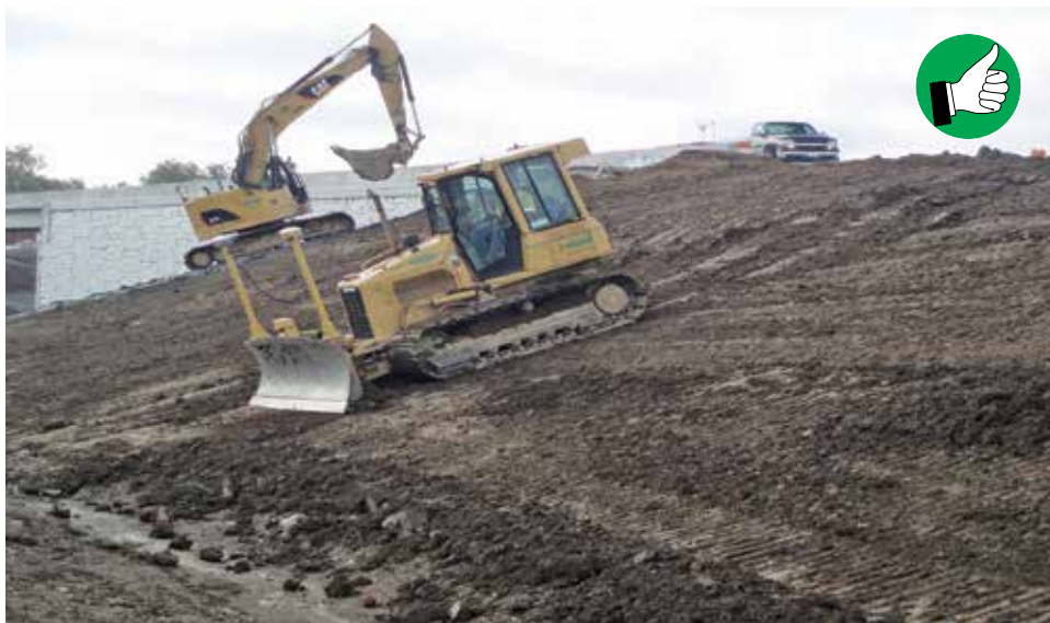
Operate bulldozer or other tracked vehicle up and down slopes before seeding to create tread-track depressions for catching and holding seed.
