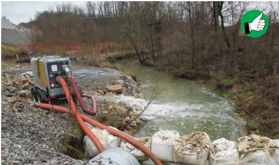
Good placement of cofferdam, pump around discharge and filter bag.
