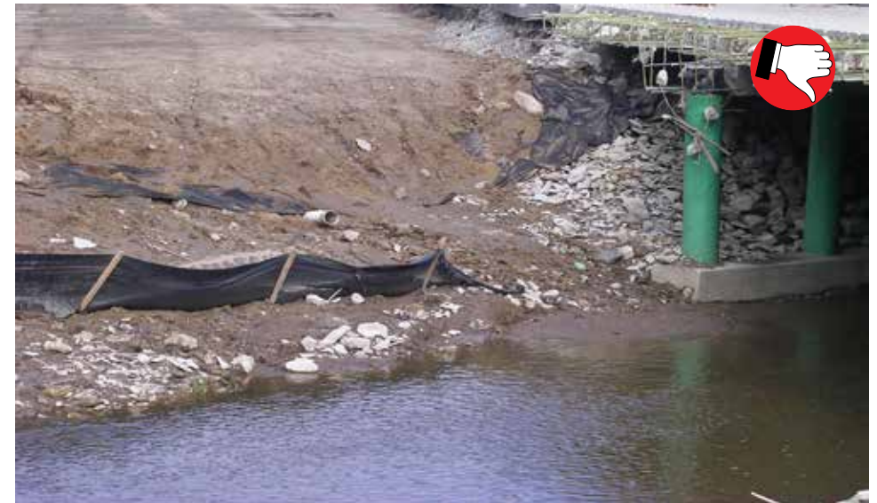
A rock filter berm would have been the correct BMP for this situation. Silt fence not sufficient and not functioning properly, sediment has moved into the stream from the unprotected slope and bank.
