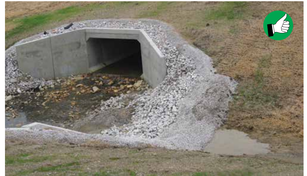
Sediment trap placed in an appropriate location close to stream with filter stone.
