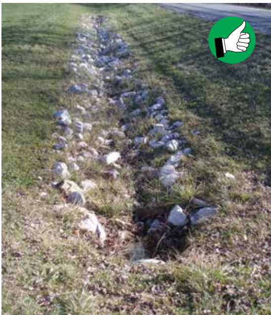
Permanent riprap ditch with correct shape and placement.
