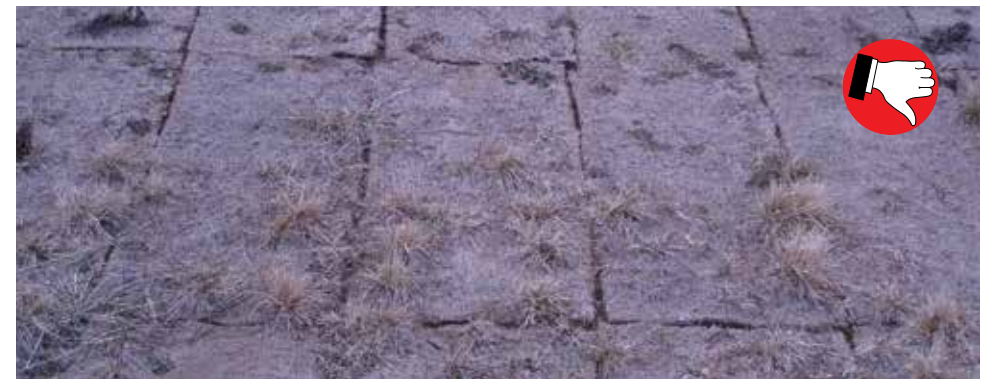
Sod was not adequately watered or otherwise maintained.
