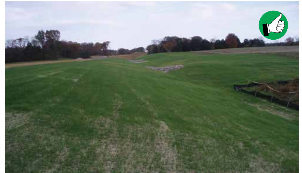
Temporary seed or permanent seed as early as possible to reduce dust on a construction site.
