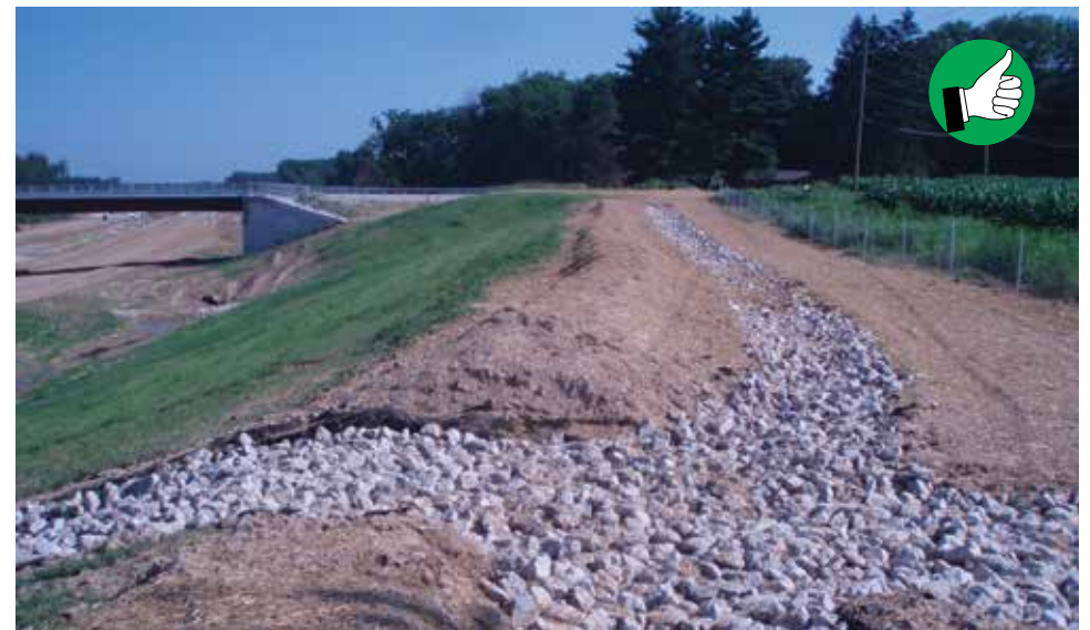
Example of permanent diversion interceptor installation.
