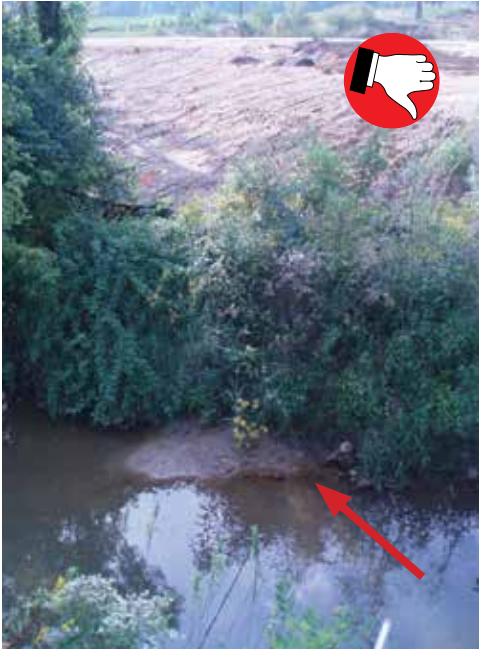
Narrow strip of vegetation on the bank is only partially protecting the stream. Note the sediment entering the waterway.
