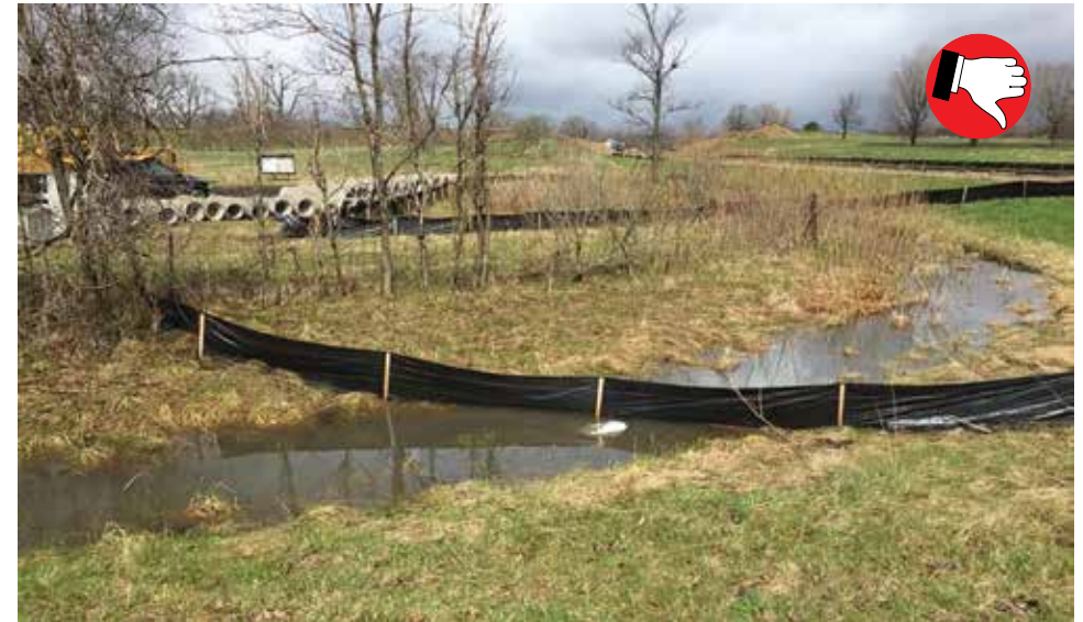
Silt fence is not an appropriate BMP for concentrated flows, nor can it be used across jurisdictional waterways.
