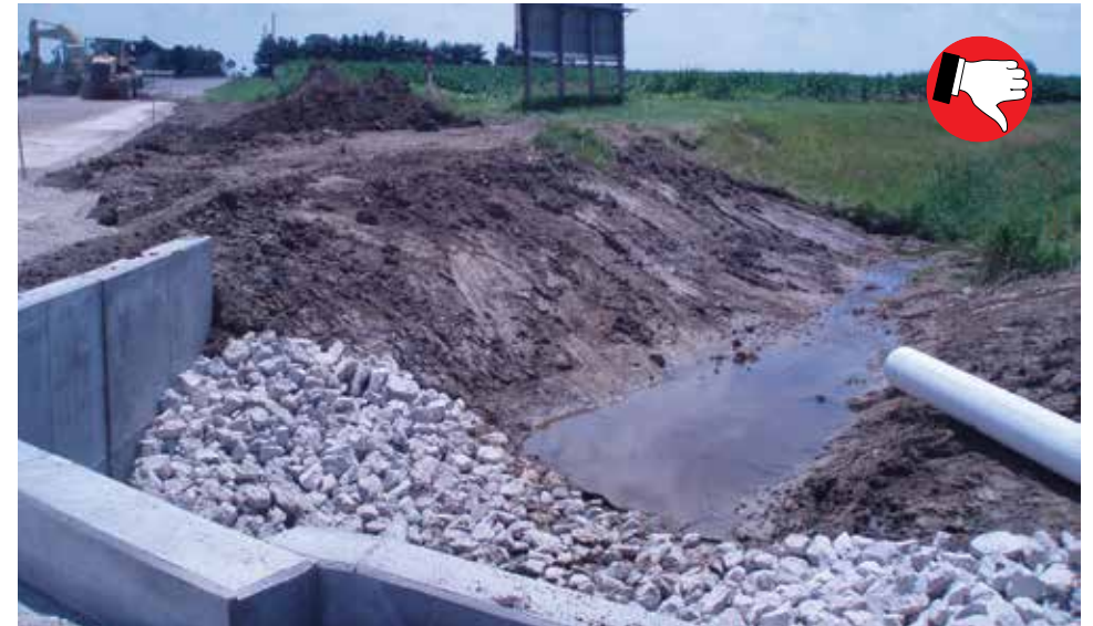
Pump around was removed prior to channel bank stabilization.
