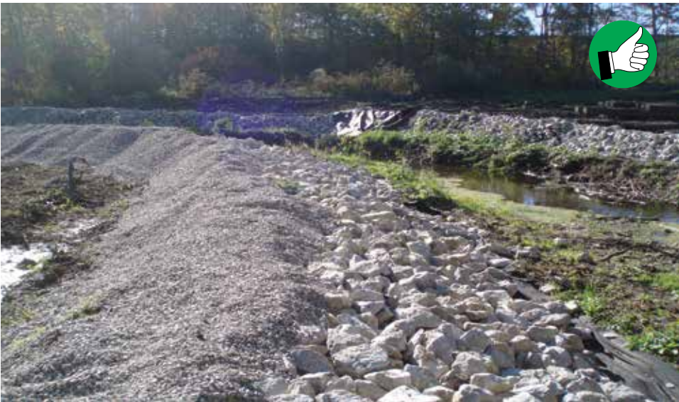
Filter berm protecting creek with geotextile, revetment riprap and filter stone. Note existing vegetation left in place between filter berm and waterway.
