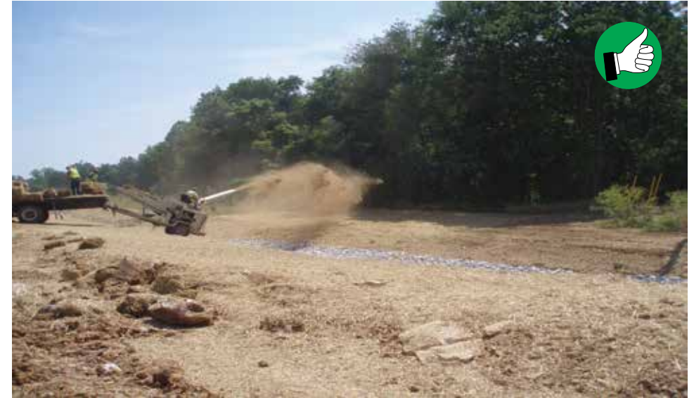
Covering exposed soil with mulch is an effective dust control practice.
