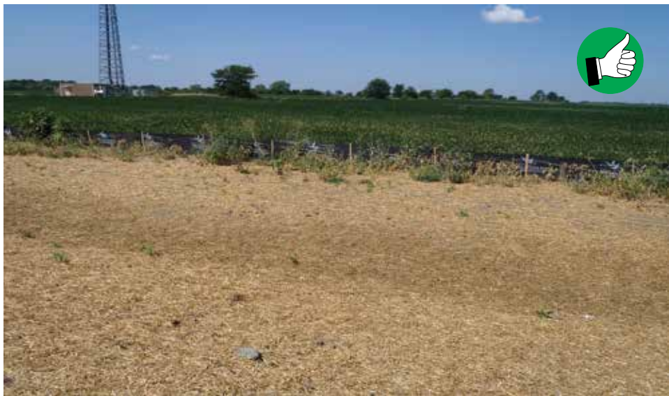
Mulch applied adequately and uniformly.
