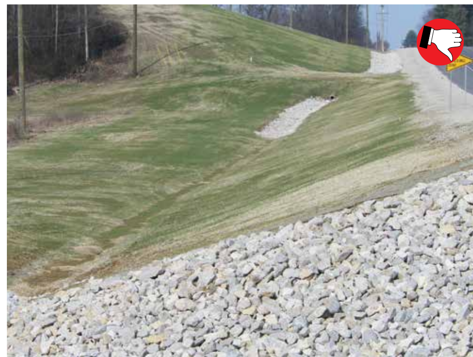
The site does not yet meet 70 percent uniform density but likely will with time. Final grade and seed as early as possible to allow more time for thick vegetation growth.
