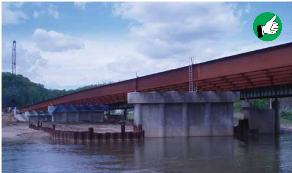
Steel sheet piling used for a working platform within the waterway.
