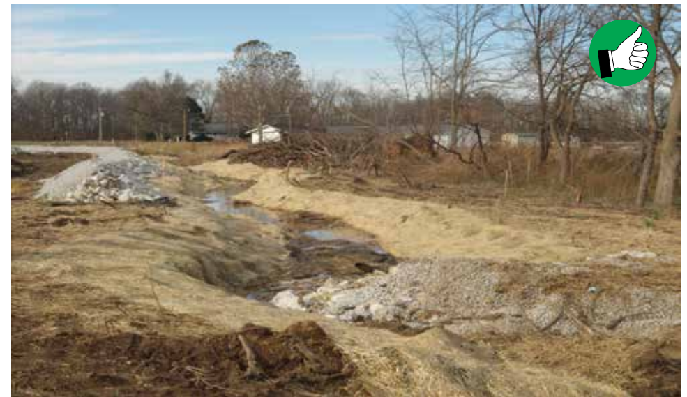
Blankets can be used as temporary or permanent erosion control around hot spots such as creek banks.
