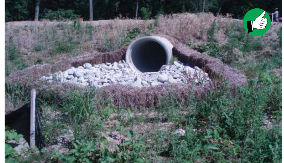
Although not an INDOT standard, straw bales and riprap functioning well for culvert inlet protection.
