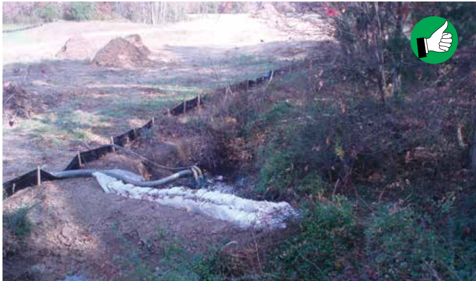
Water tight cofferdam on upstream side with adequately sized pump.
