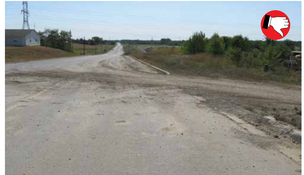
Insufficient #2 stone on construction entrance. Note tracking onto public roadway. Mud tracked onto paved roads becomes a safety issue.
