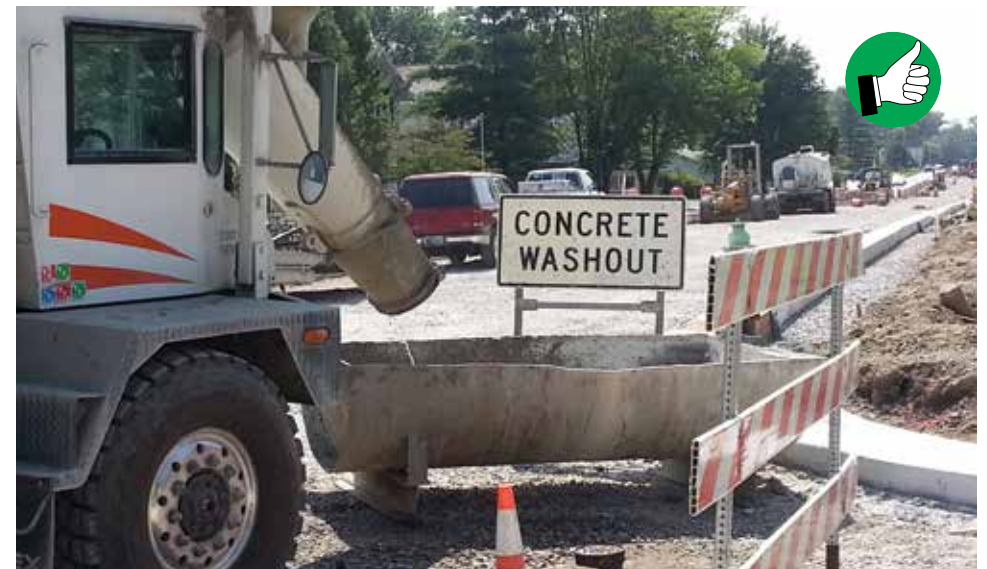
Concrete washout water held within an impermeable container with signage.
