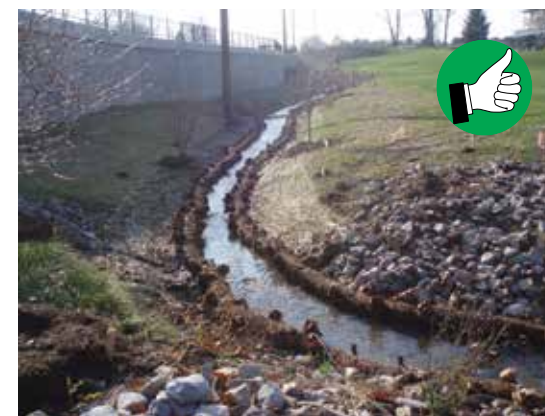
Filter socks used for channel stabilization.
