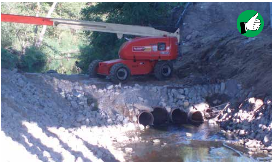
Temporary crossing with adequate pipe capacity. These temporary impacts must be permitted, usually by the contractor, prior to installation and should be removed as soon as practical.
