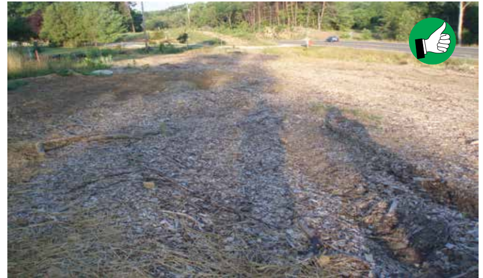
Wood chips from tree clearing used as erosion control for sheet flow area.
