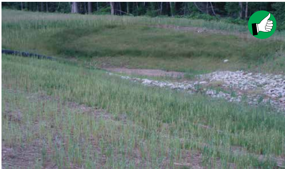
Temporary vegetation and slope drains providing slope stability.
