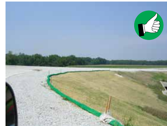
Filter socks can be used on the edge of pavement to slow water before vegetation is established.
