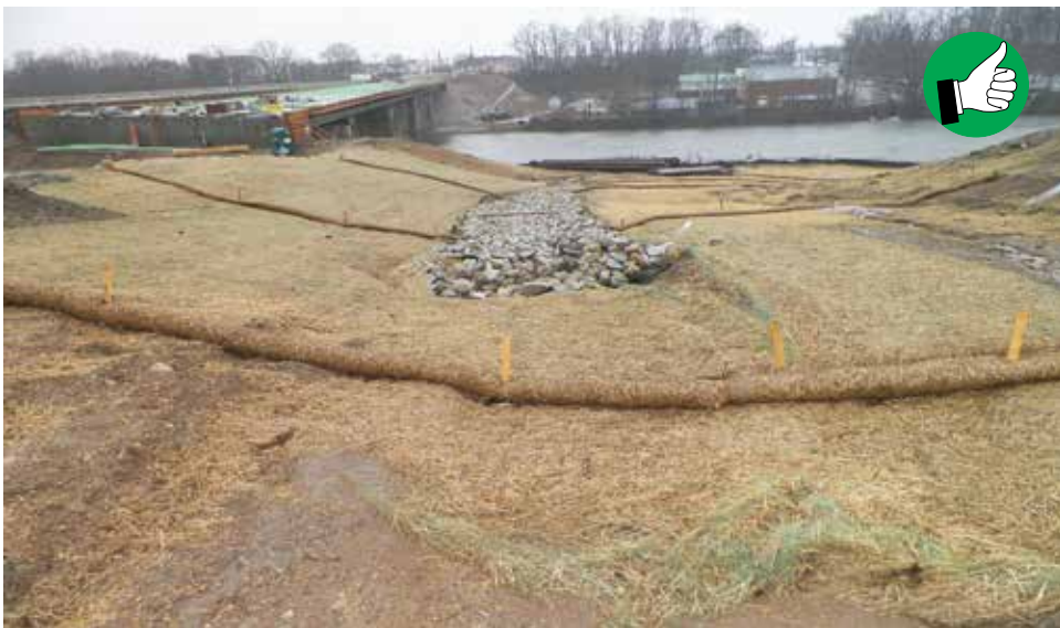
Filter socks can be placed horizontally across a slope to shorten a slope's length and prevent rill and gully erosion.
