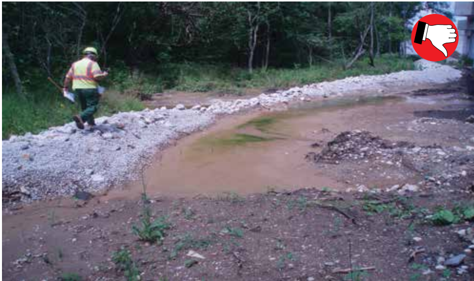
Filter berm after a large rain event that needs maintenance.
