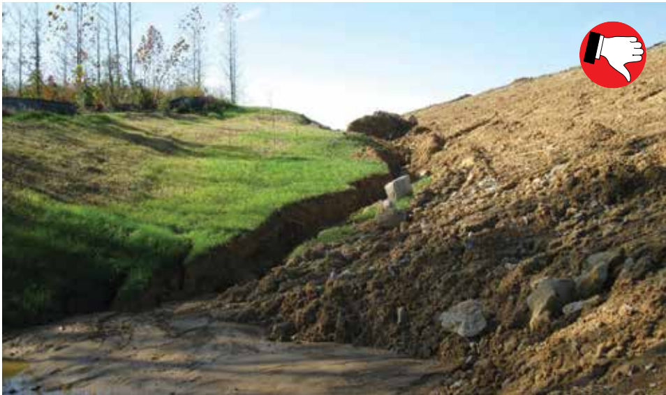
Permanent riprap should be installed in steep ditches to prevent gully erosion.
