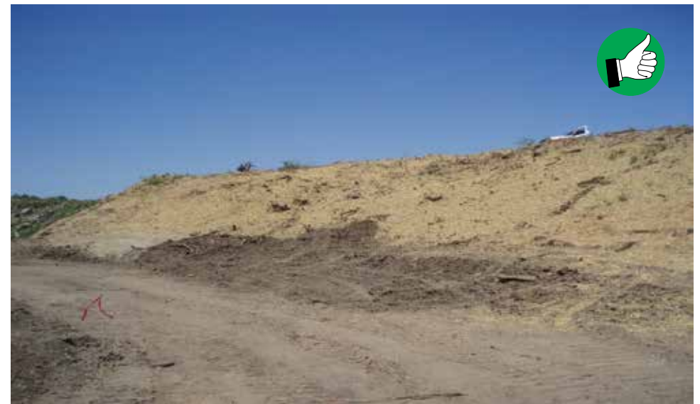
Stockpiled soil protected with mulch.
