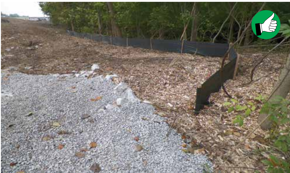
“J” hook the end of the silt fence uphill to prevent water from bypassing fence.
