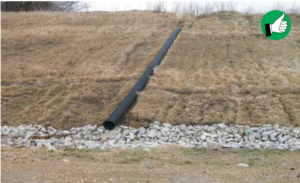
Slope drains properly constructed with a stable outlet.
