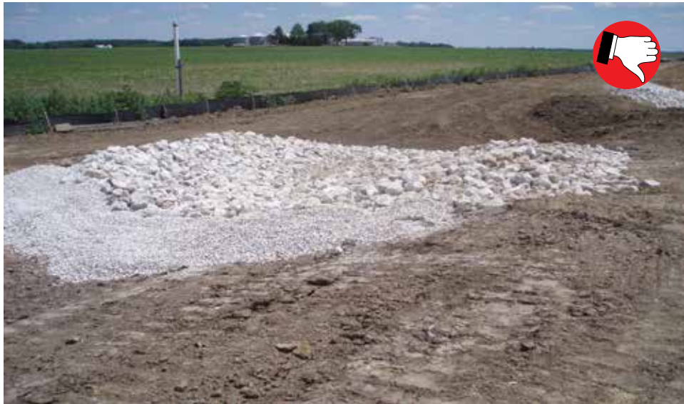
Check dam is much bigger than necessary. Wasted material, wasted money, can cause flooding, and will be much more difficult to remove.
