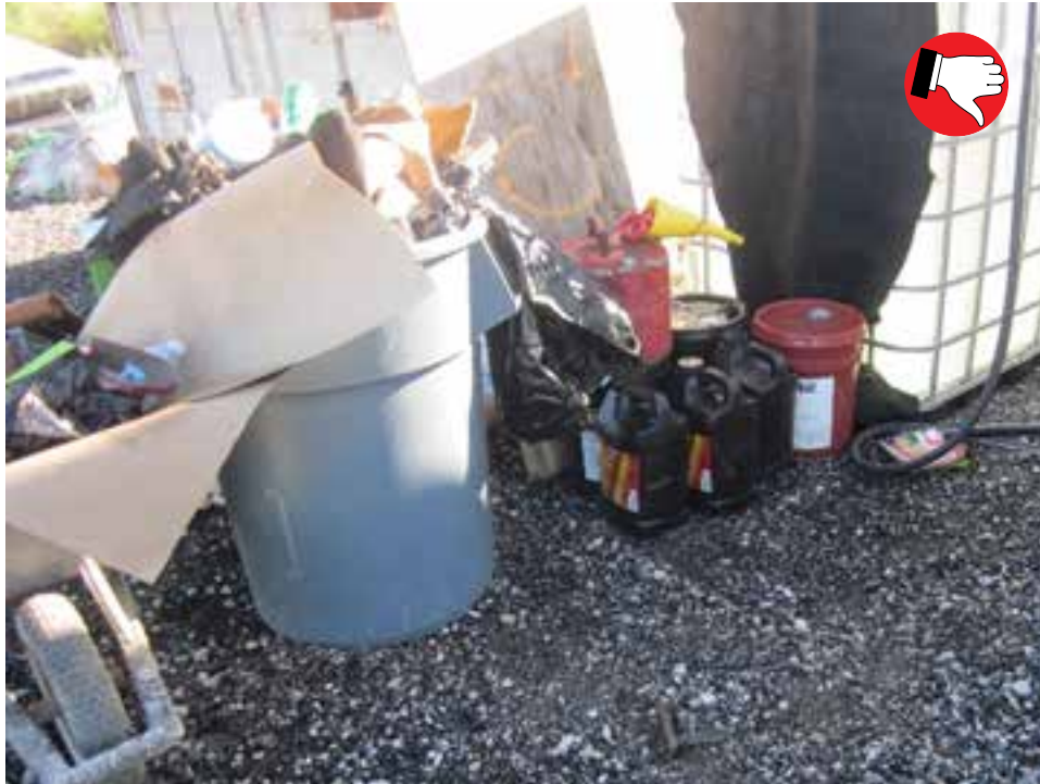
Trash and liquids not stored properly.
