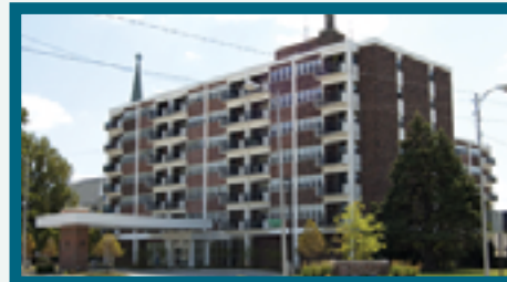
RAD I PROJECT #14-14 RENOVATIONS to John F. Kennedy Towers Modernization of 99 units located in a 7 story High Rise. Located at 315 SE Martin Luther King Jr. Blvd. Evansville, Ind.
