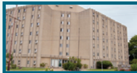
RAD I PROJECT #14-14 RENOVATIONS to White Oak Manor Modernization of 115 units located in a 7 story High Rise. Located at 509 N. St. Joseph Avenue, Evansville, Ind.
